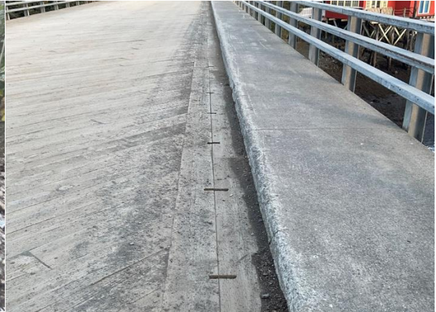
Seldovia Slough Bridge Deck Drains
