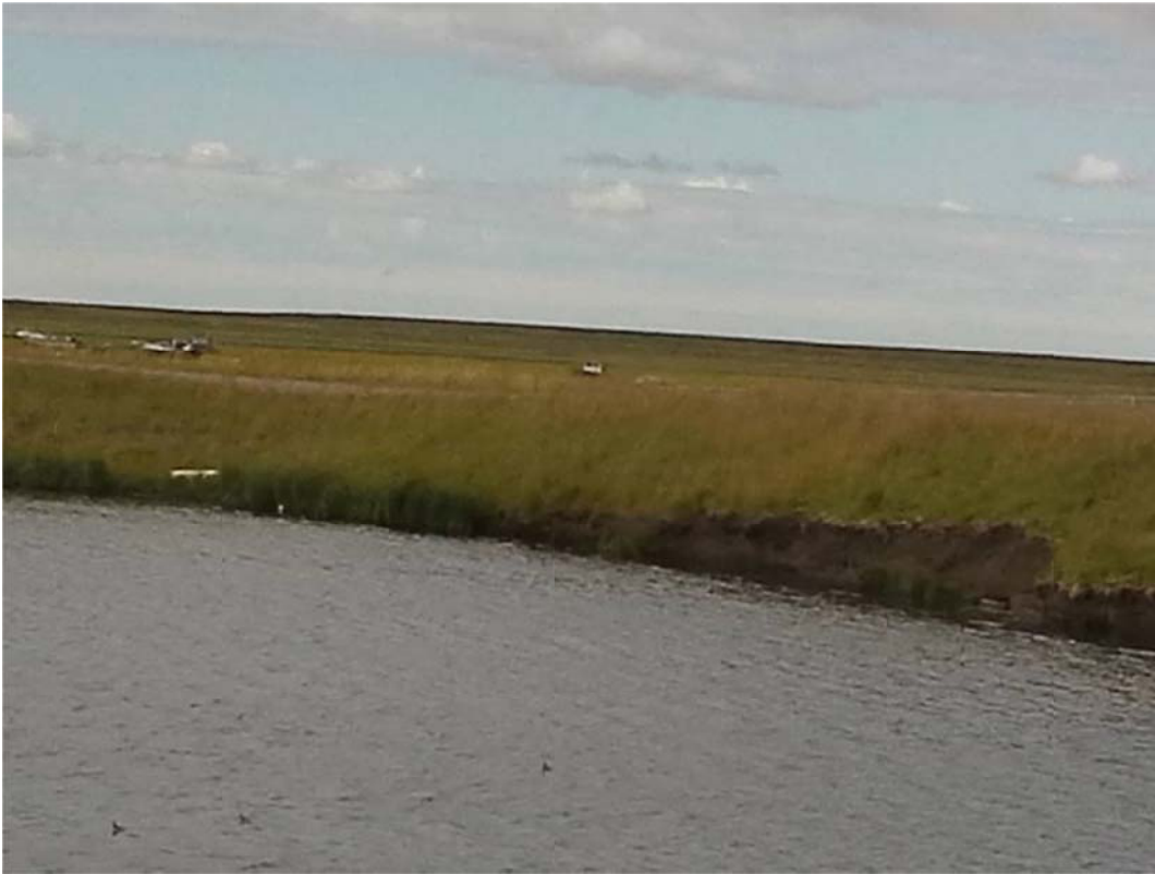
Photo of erosion during summer months. This erosion is exhibiting calving of the berms above the erosion blanket. Photo provided by Susan Randlett.
