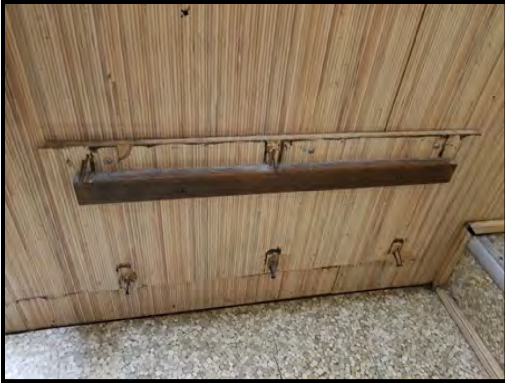
Figure 11: Women's shower, water damage along wall and floor.
