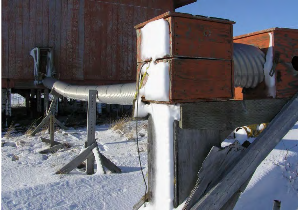
Figure 3 - Well System and Transmission Line
