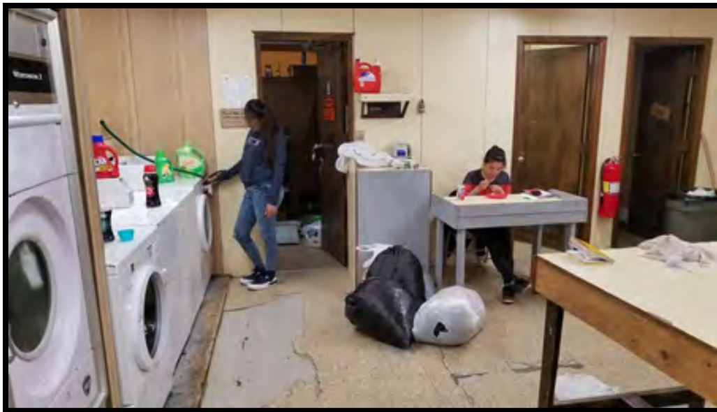
Figure 8: Washer, manual filling with hose.
