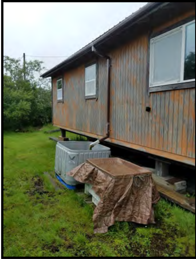
Figure 19: Rainwater collection system.
