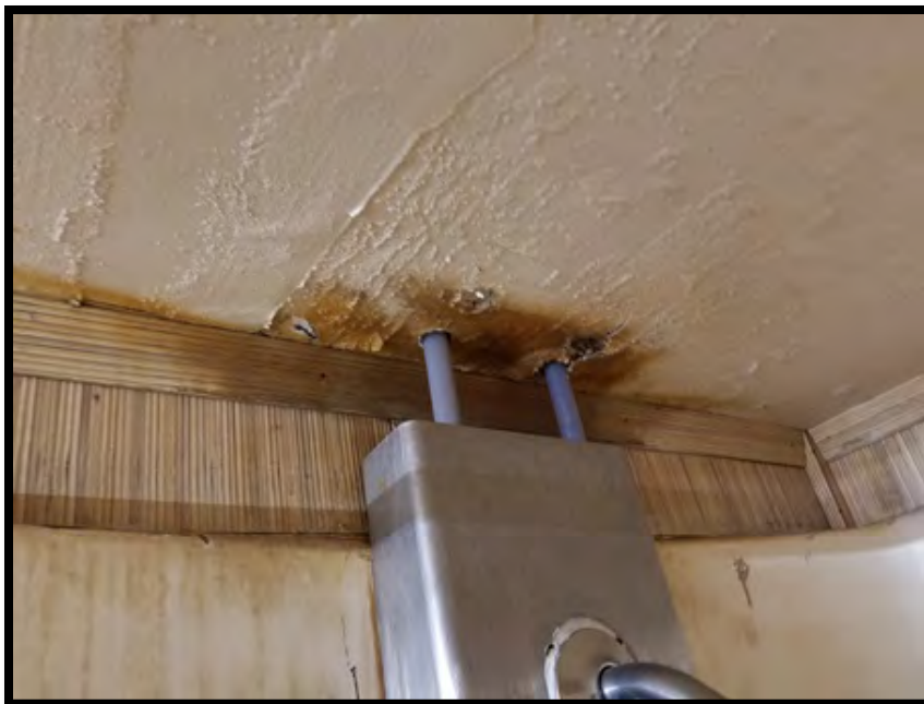
Figure 10: Women's shower, water damage and mold.
