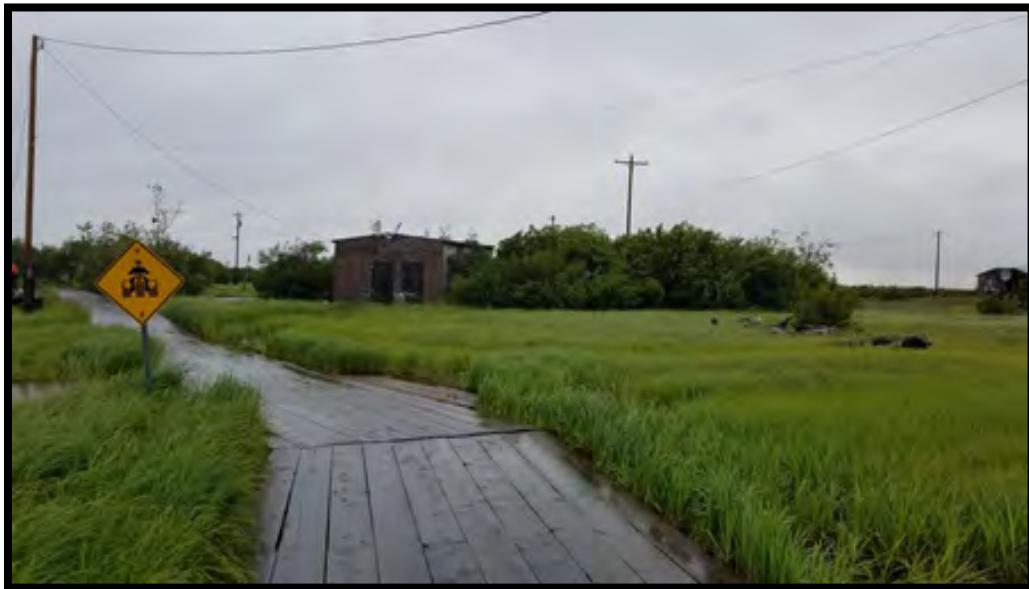
Figure 14: Typical boardroad, floating on tundra and marshy area
