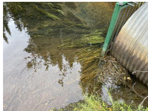
Picture 18 - Scour evident at culvert inlet and outlet
