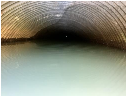
Picture 31 - West culvert outlet. Culvert settlement is occurring mid-culvert.
