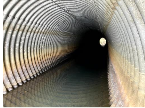
Picture 23 - Culvert integrity is evidenced by a lack of deflection; high-water mark is visible near the crown of the culvert.
