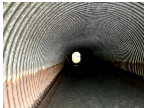
Picture 15 – Flattening of culvert is evident in the middle section; rust is present to 1/3 of culvert height.
