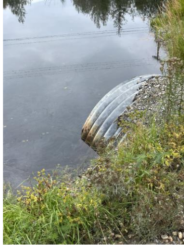
Picture 7 – Culvert outlet
