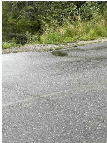
Picture 9 – Road settlement occurring over culvert inlet
