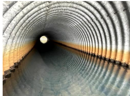
Picture 36 - Culvert is not settling or deforming
