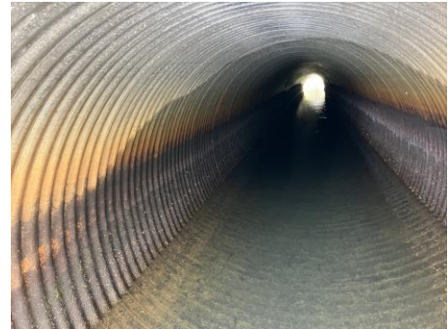
Picture 19 - Rust visible on sidewall with fish swimming in culvert Picture 20 - Culvert has maintained structural integrity
