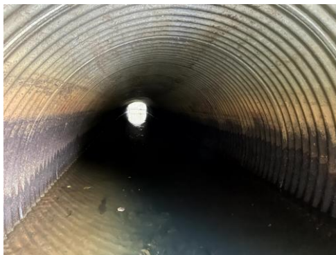
Picture 17 - Interior rust to \frac{2}{3} height of the culvert wall
