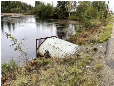
Picture 35 - Hurst Road culvert inlet
