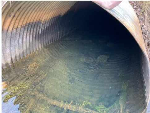
Picture 19 - Rust visible on sidewall with fish swimming in culvert Picture 20 - Culvert has maintained structural integrity
