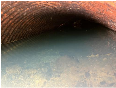
Picture 29 & 30 - West culvert inlet shows debris and significant rust accumulation.
