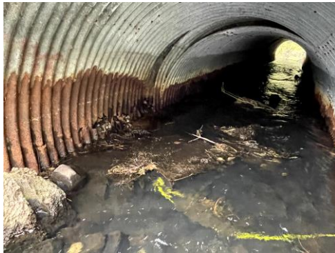
Picture 11 - Culvert rusted out and seams separating
