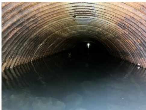
Picture 27 - East culvert inlet, rust line shows that the culvert frequently ran full in the past (likely when plugged by beaver debris)
