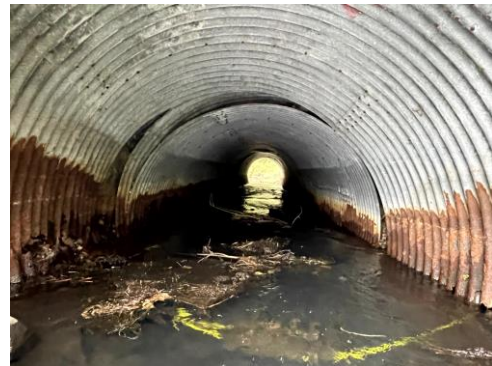
Picture 10 – Culvert seams separating at inlet
