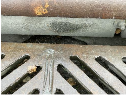
Picture 16 - Storm drain is filled with sediment
