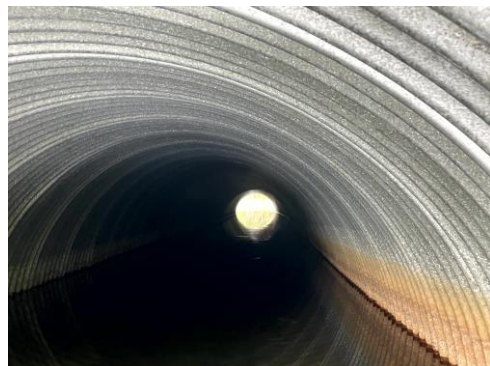
Picture 6 – Interior of 7' culvert demonstrates culvert's integrity
