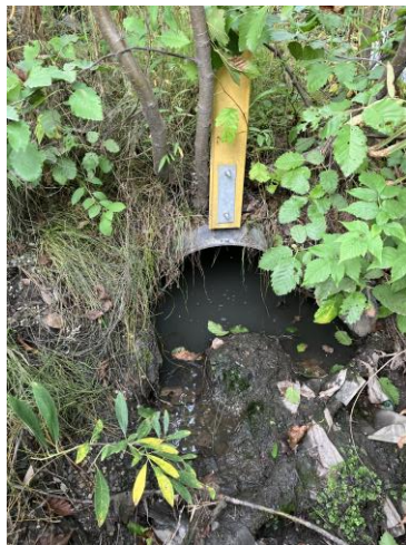
Picture 24 - Storm drain outlet is partially obscured
