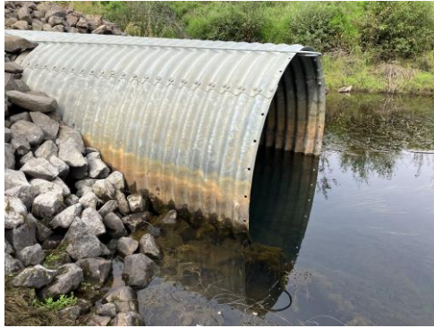
Picture 22 - Rock at the inlet and outlet prevent bank scour
