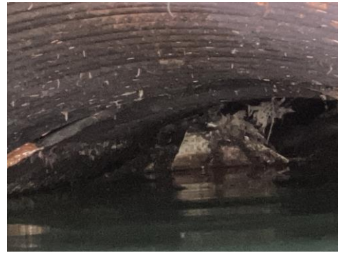
Picture 29 & 30 - West culvert inlet shows debris and significant rust accumulation.
