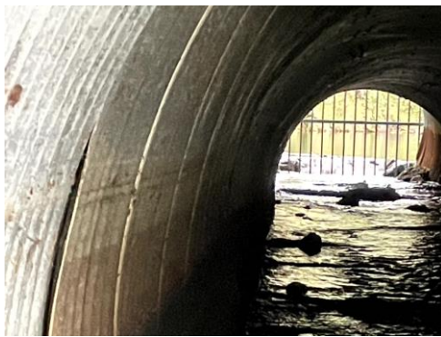
Picture 11 - Culvert rusted out and seams separating
