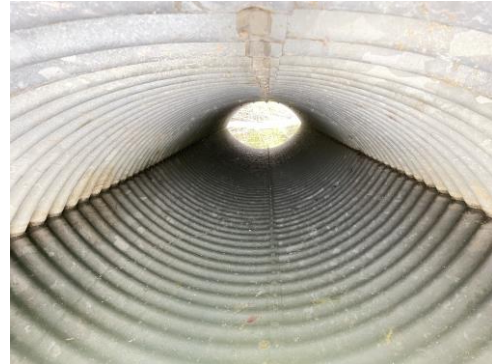
Picture 8 – Culvert interior shows minimal rust and deformation.
