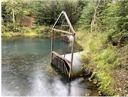
Picture 26 - The outlet of east culvert is in the background and outlet of west culvert is in the foreground. The east culvert has been cleared of debris and is fully functional. The west culvert is partially blocked by both debris and culvert settlement.
