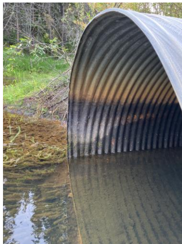
Picture 21 - Rust at culvert outlet
