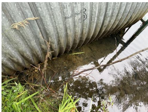
Picture 14 - Scouring along the exterior of the culvert
