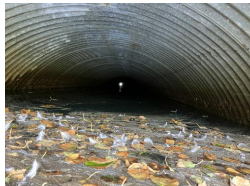
Picture 28 - East culvert outlet. Some settlement is evident.
