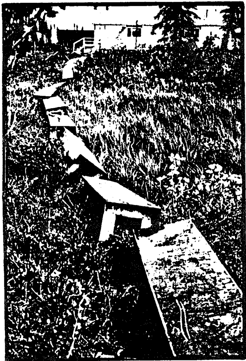
UTIDOR SECTIONS BEFORE CONNECTION
