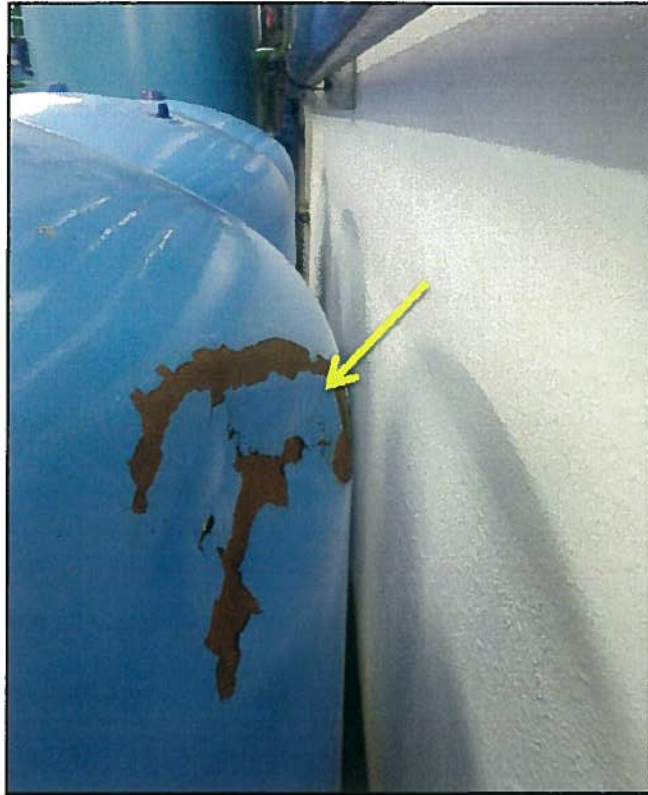
Figure 21: Damaged (Dented) Hydropneumatic Tank
