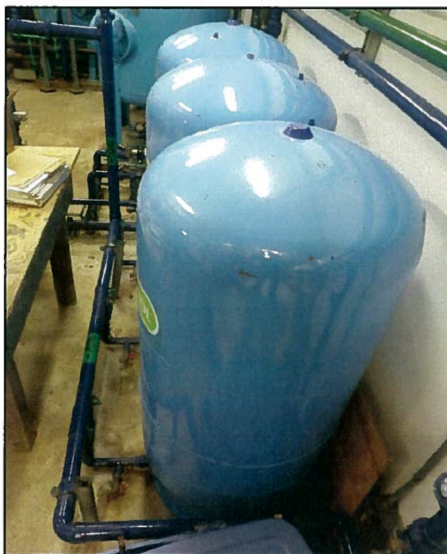
Figure 20: Hydropneumatic Tanks
