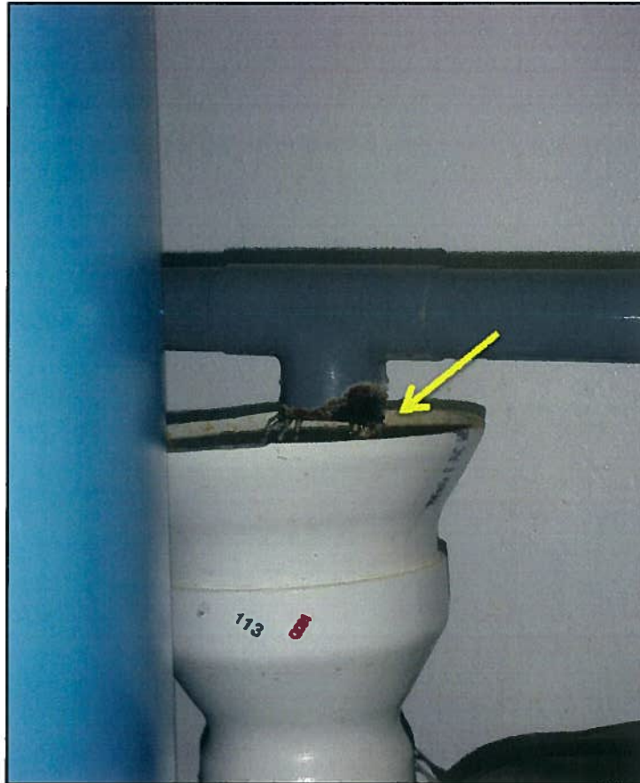
Figure 9: Filter Backwash Discharge Into Sump - Air Gap (<2D)
