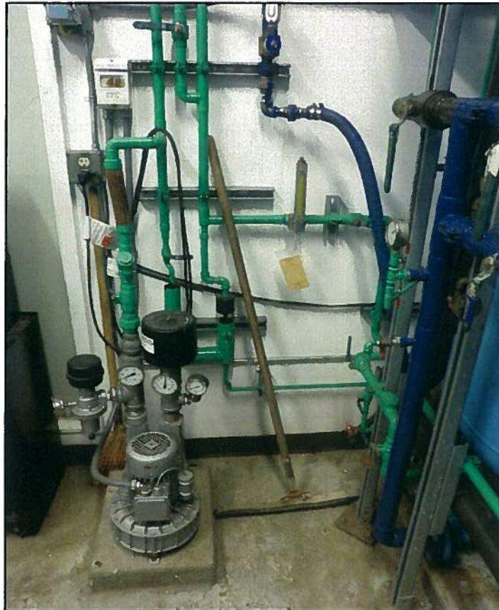
Figure 15: Air Blower Setup for Air Scour
