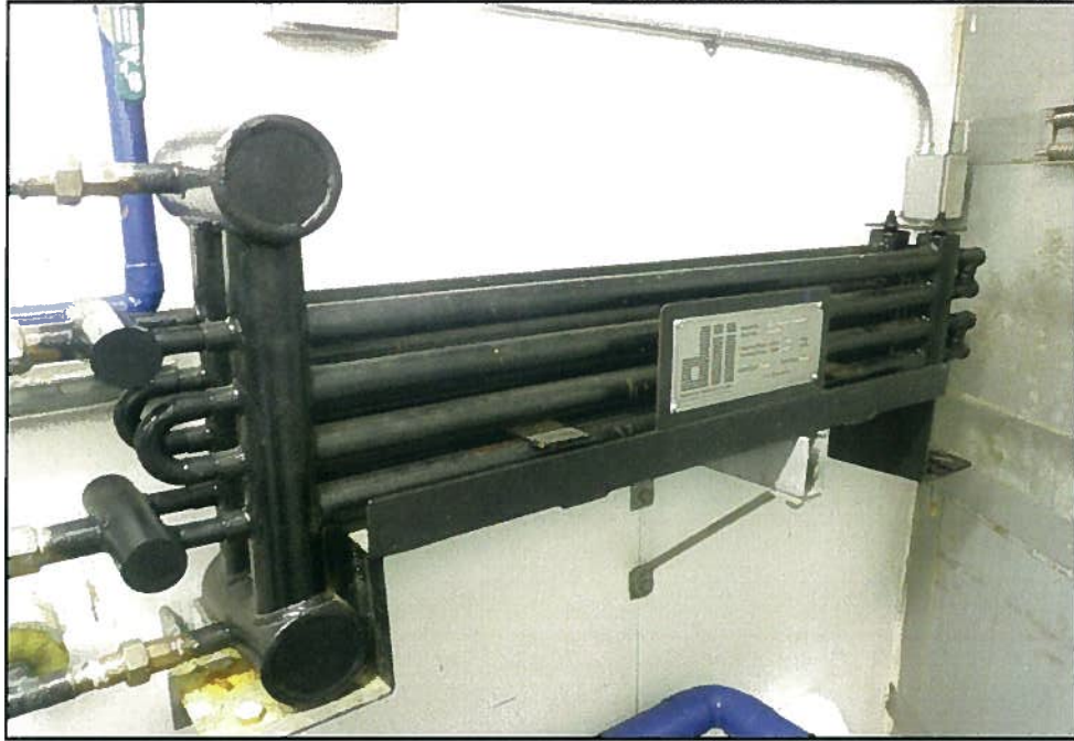
Figure 17: Heat Exchanger
