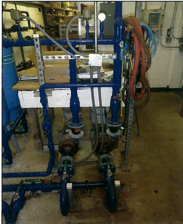
Figure 18: Distribution Pressure Pumps
