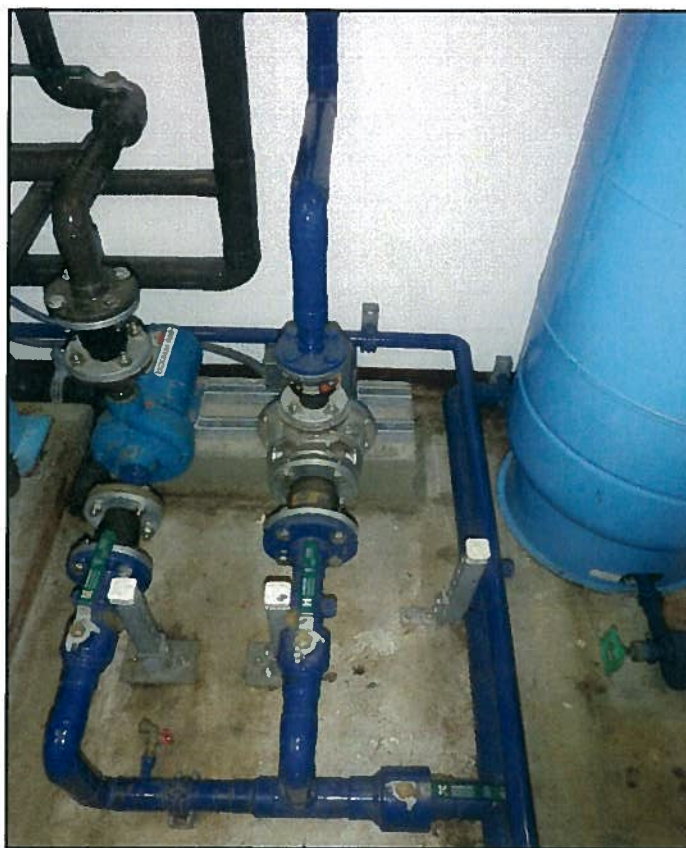
Figure 19: Backwash Pump & Truck Fill Pump
