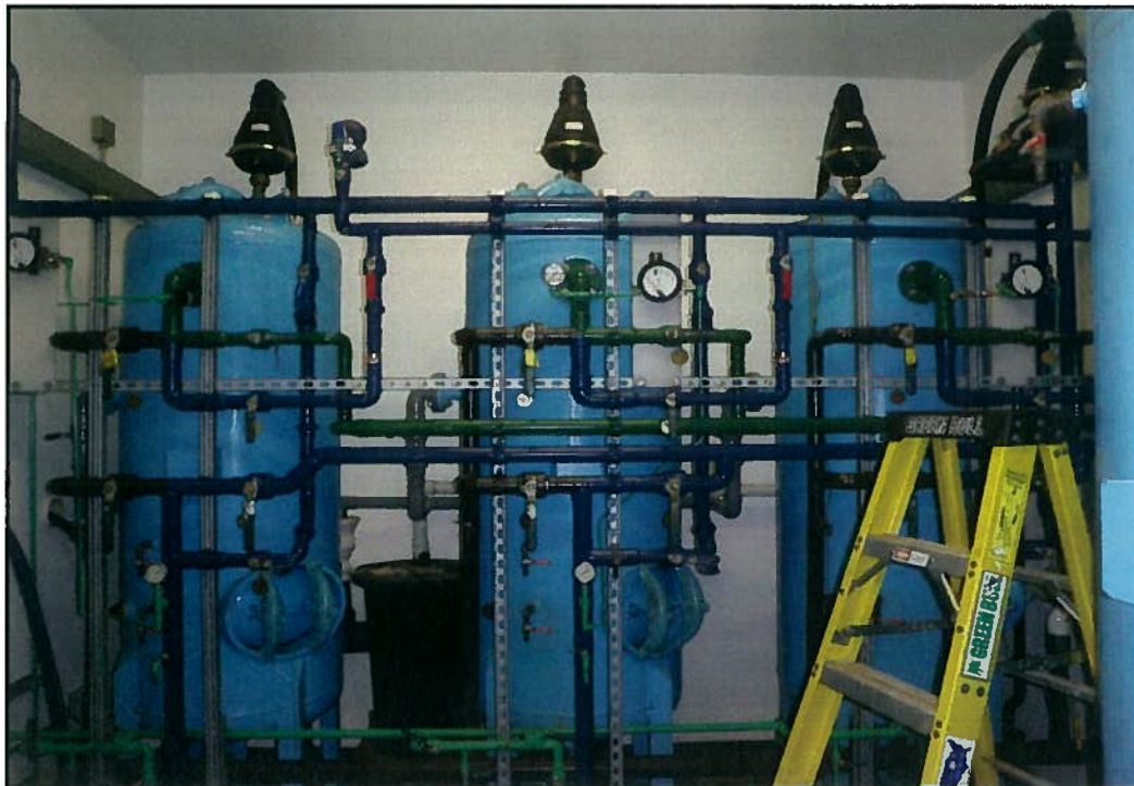
Figure 12: Greensand Filters
