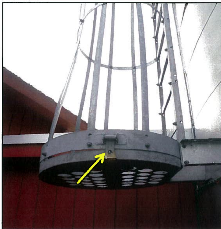
Figure 24: Locked WST Access Ladder
