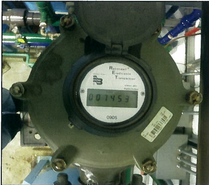
Figure 13: Backwash Flow Meter (Not Functioning)
