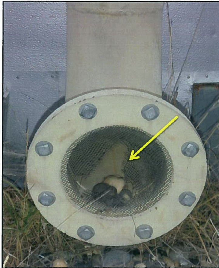
Figure 23: Torn WST Overflow Screen
