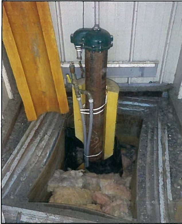
Figure 5: Well Casing
