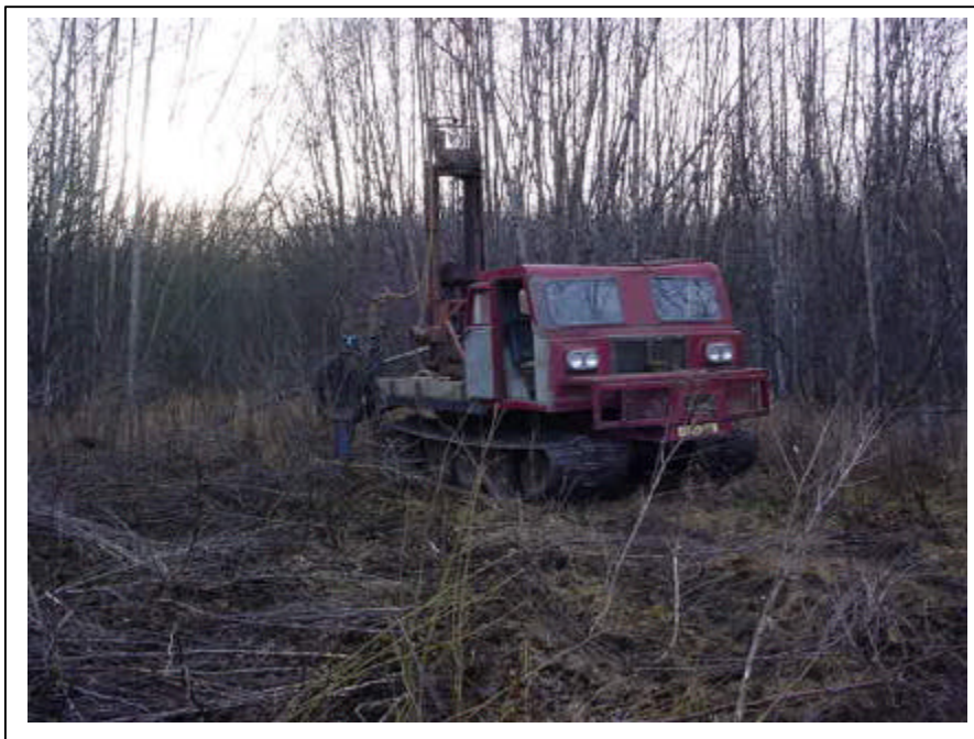
Photograph 19: Looking southwest, Boring FB1 was advanced in the southwest corner of Area F.
