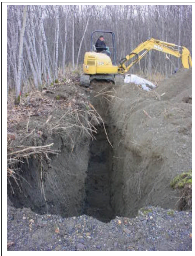
Photograph 2: Looking northwest, the northwestern septic trench was advanced along the former septic lines toward the seepage pit.
