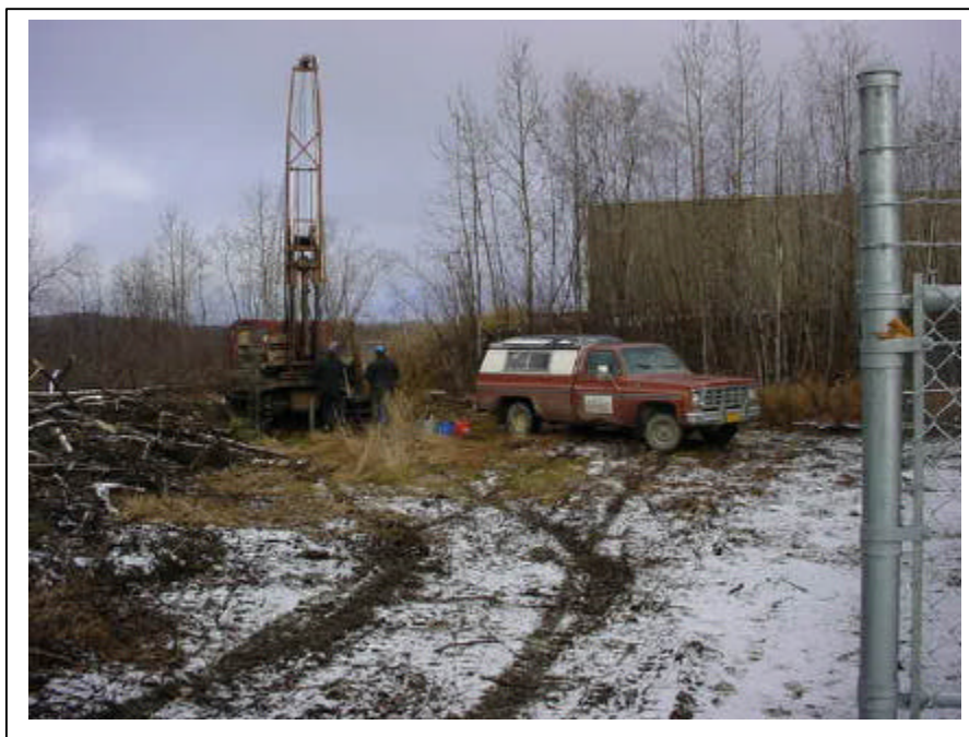
Photograph 16: Looking north, Boring B5 was advanced to the southeast of Area F.
