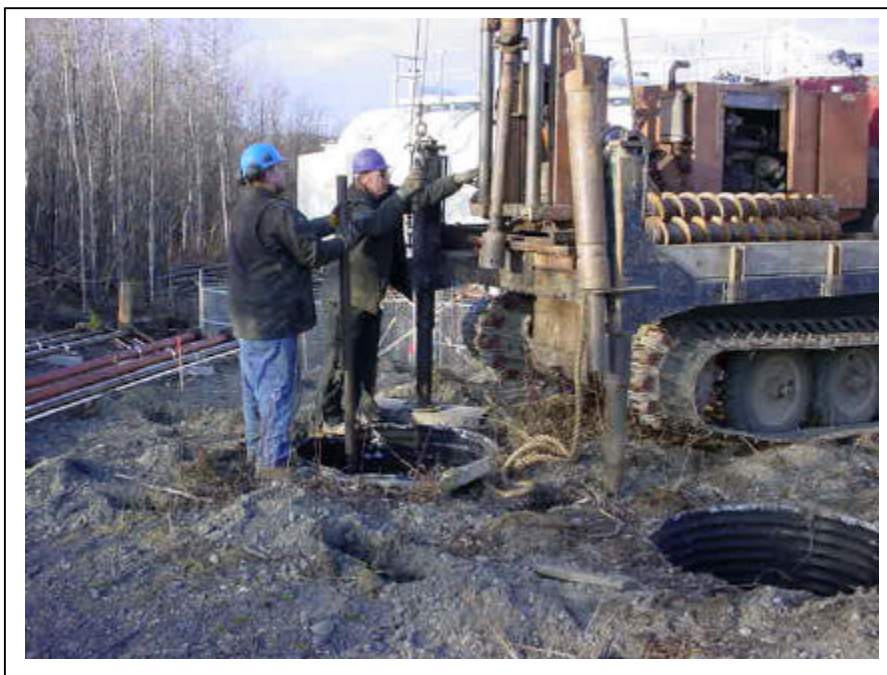
Photograph 12: Looking northwest at CMP2, a split-spoon sampler was used to sample the CMP.
