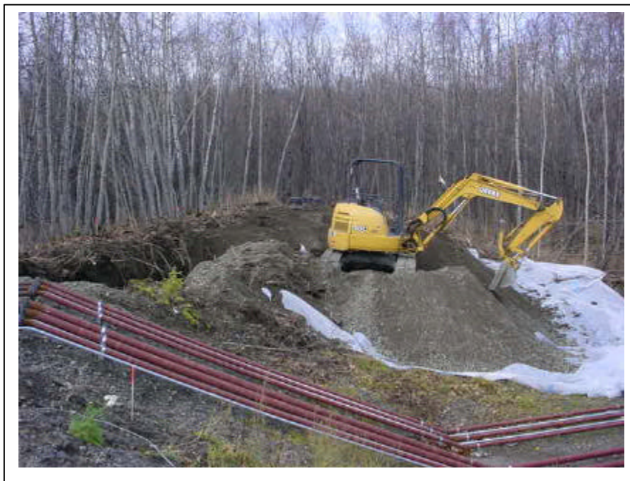
Photograph 6: Looking northwest, the trench was backfilled following sampling activities.
