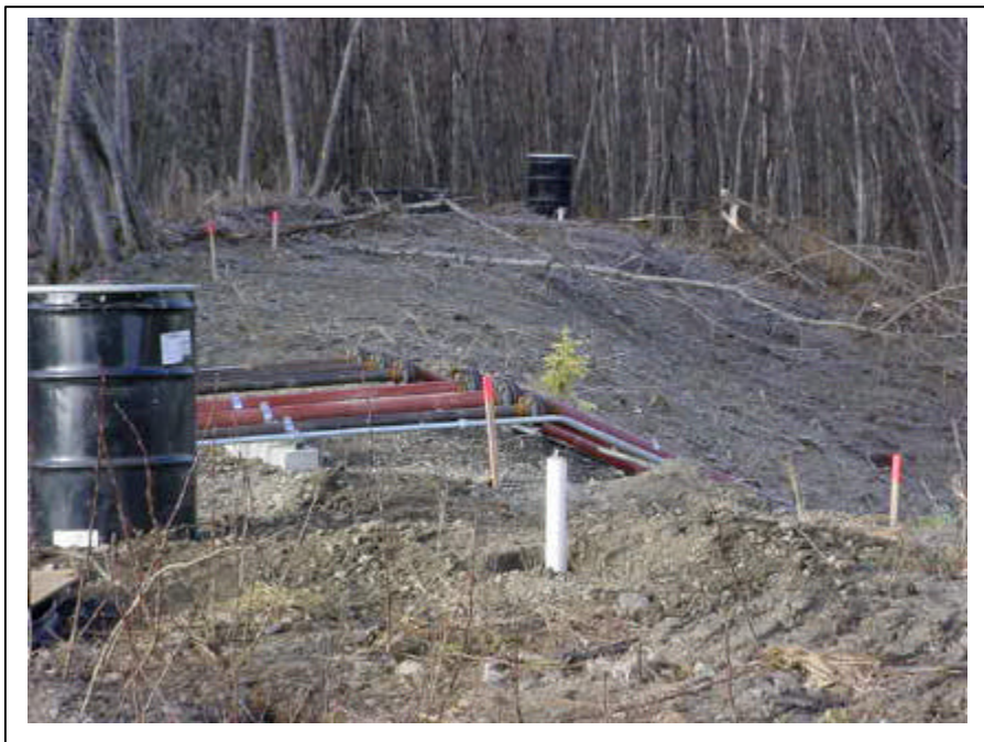
Photograph 17: Looking northwest, Monitoring Wells MW1 (back) and MW2 (front) were installed in Borings B1 and B2, respectively.
