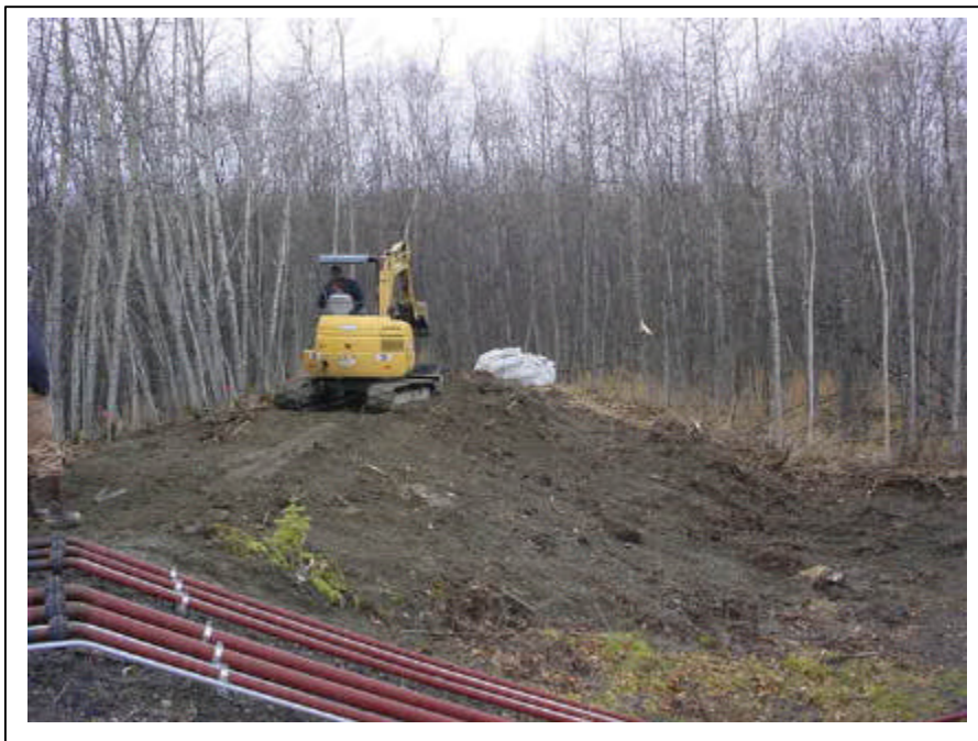
Photograph 7: Looking northwest, the northwest septic trench was compacted with the tracks of the backhoe following backfill activities.
