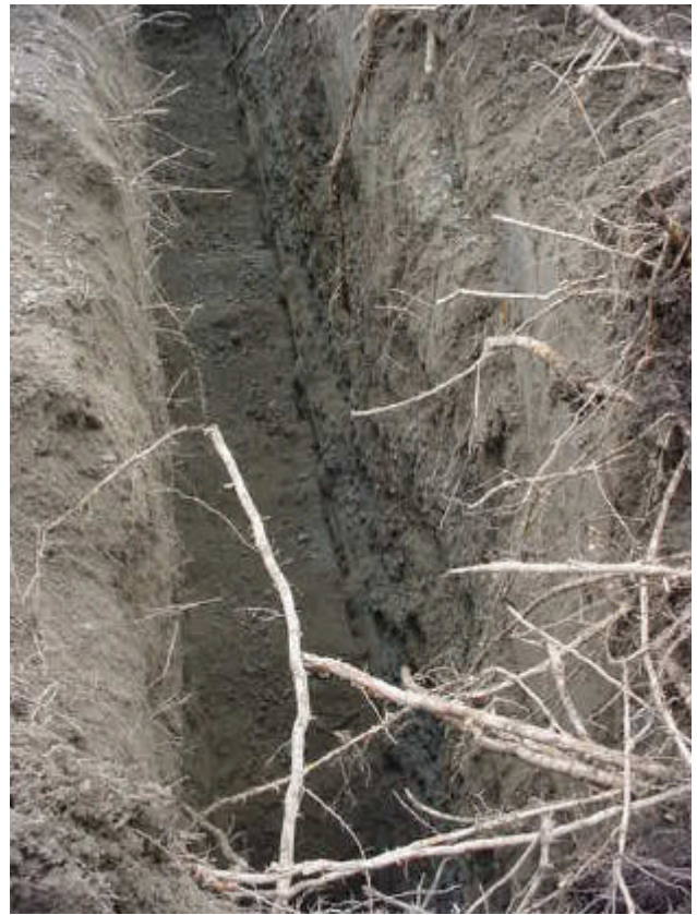
Photograph 3: Looking southeast into the northwest septic trench, the former septic line (on the right at the bottom of the trench) was encountered at 9.5 to 10 feet bgs.
