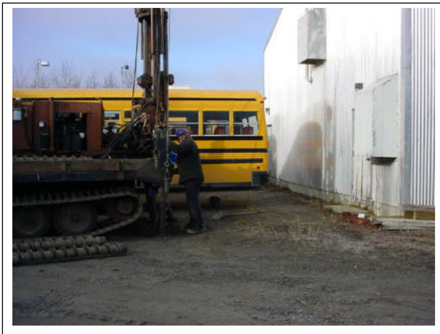
Photograph 15: Looking northwest, Boring B4 was advanced to the south of the KSD maintenance building.
