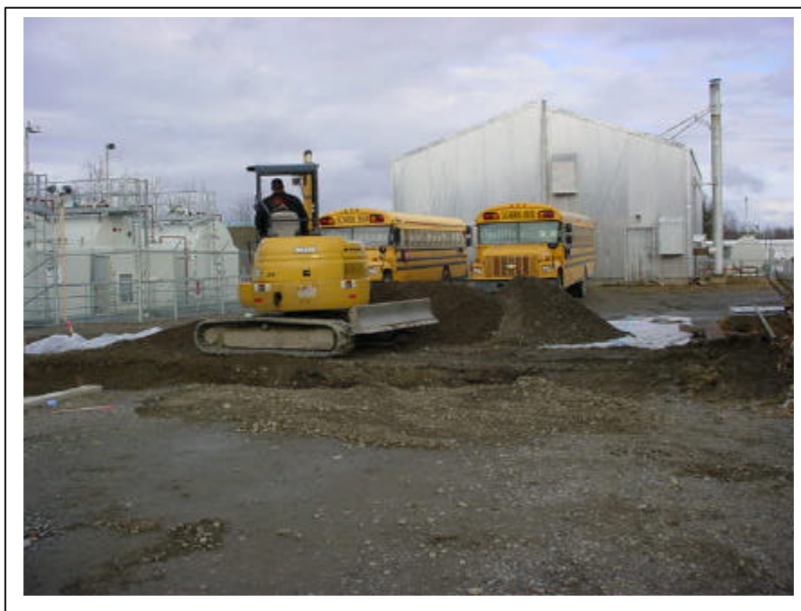
Photograph 8: Looking north, the southeastern septic trench was backfilled following sampling activities.
