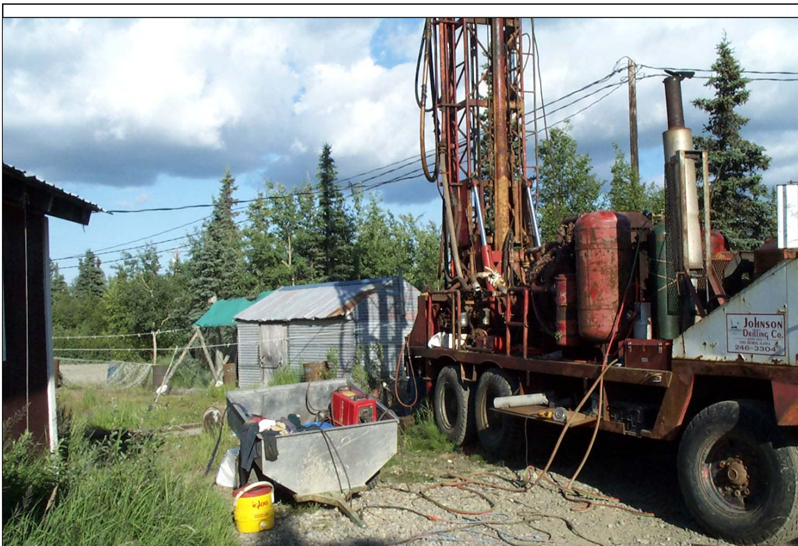
Well Site 02NELS-07. Drill rig and miscellaneous equipment set up during drilling operation.
