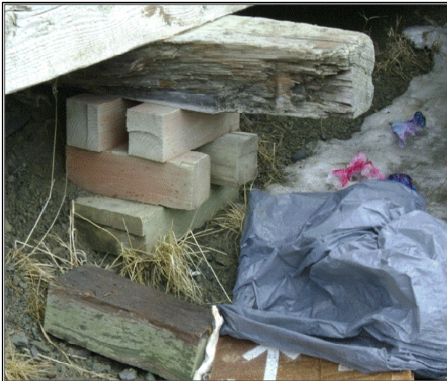
Photo 2: Detail of undermined building cribbing below abandoned watering point.
