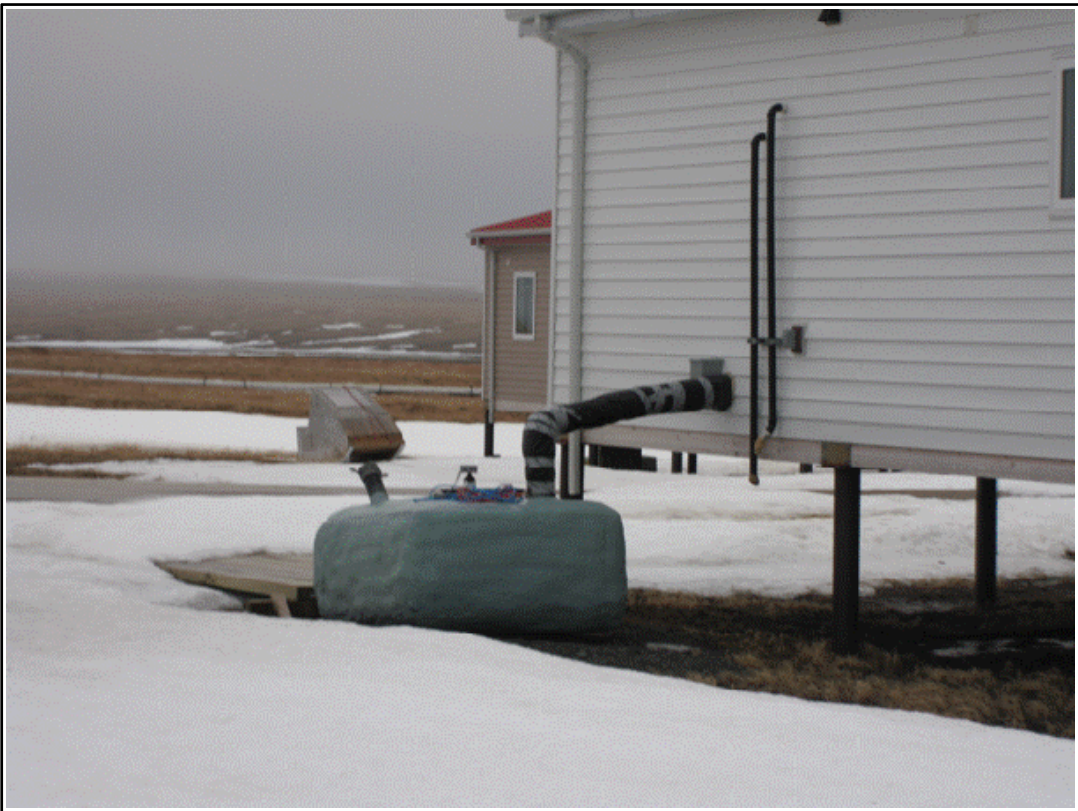
Photo 30: FTH holding tank at HUD subdivision home.
