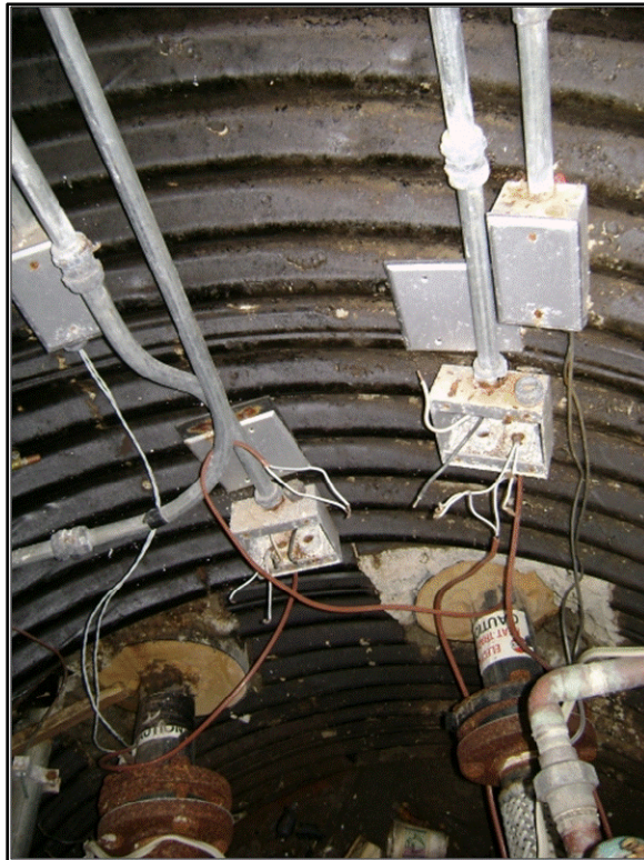
Photo 20: Valve pit of Watering Point #2. Heat trace power and sensor wiring.
