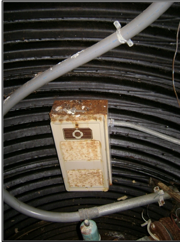
Photo 19: Valve Pit heater for Watering Point #2.
