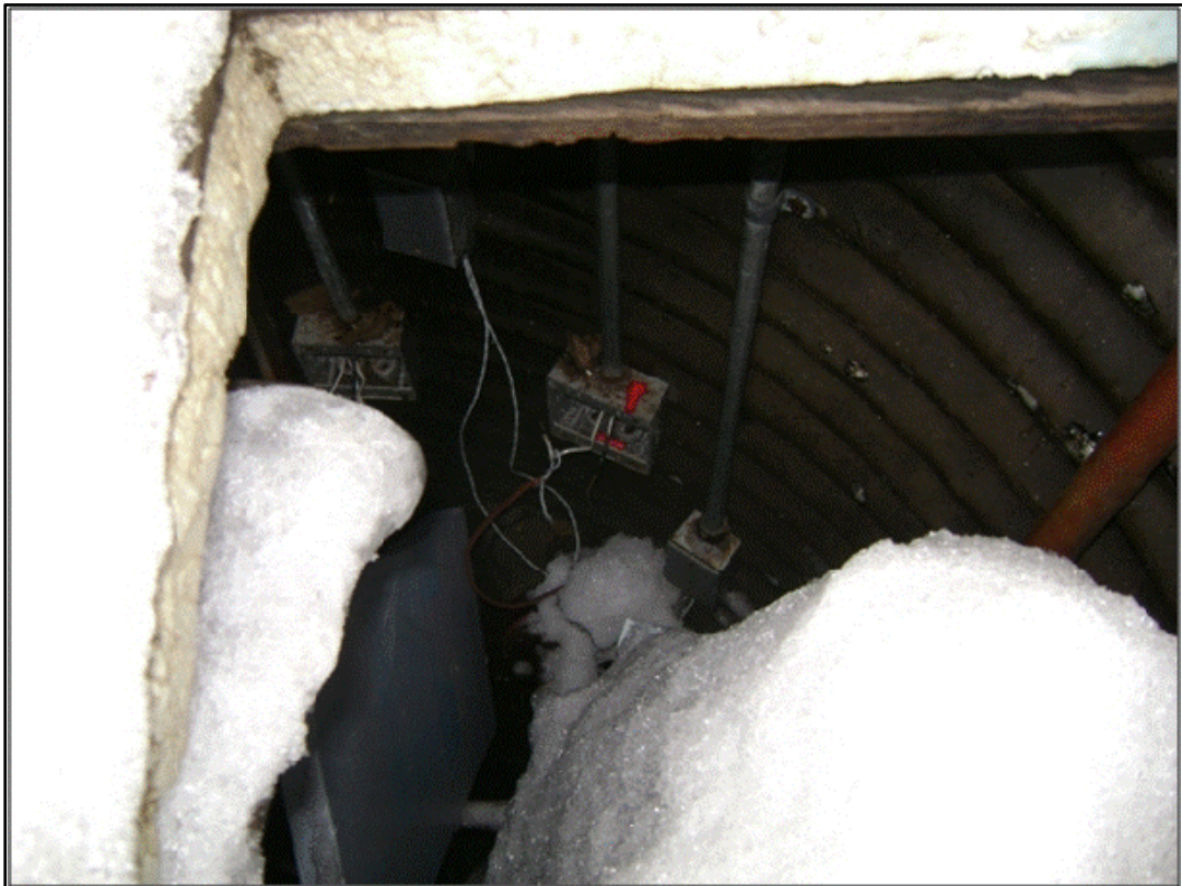
Photo 18: Valve pit of Watering Point #3. Snow packed with heat trace power and sensor wiring connections exposed.
