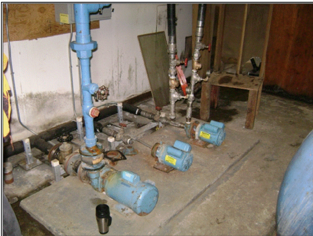
Photo 13: Backwash pump (foreground) and pressure pumps (only one serviceable).
