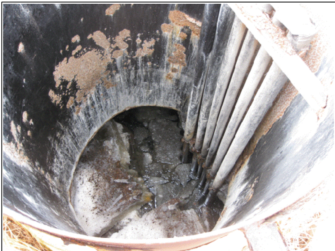
Photo 36: Frozen outlet in dosing tank on the In-Complete septic system.
