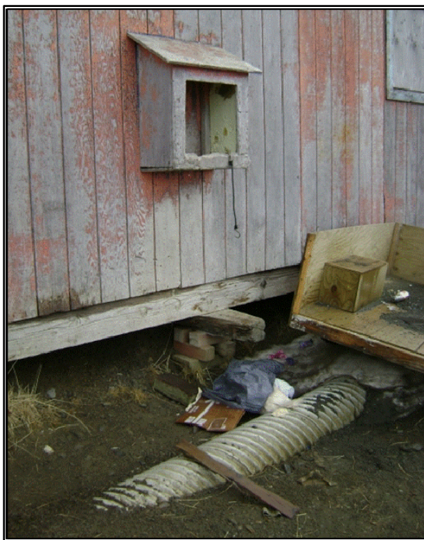
Photo 3: Abandoned watering point showing erosion of building footings. Arctic pipe from water source previously buried has been exposed.
