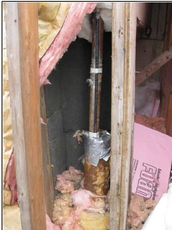
Photo 42: Exposed section of 4-inch steel well serving the former BIA school water system. Note the duct tape well cover.
