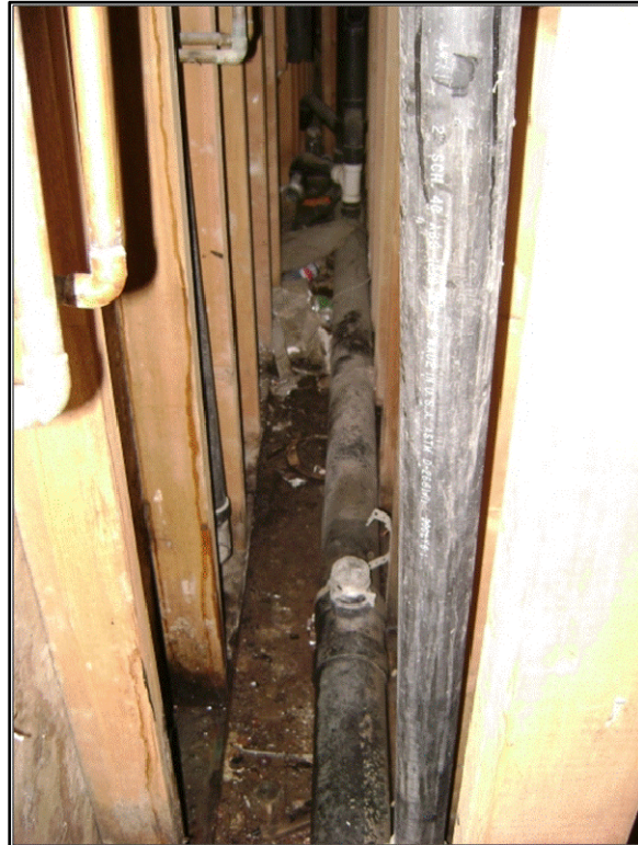
Photo 10: Showing disconnected drainage piping improperly sealed.
