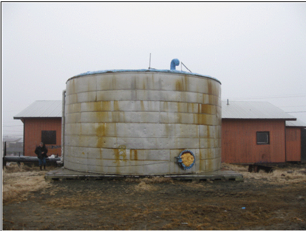
Photo 34: Deteriorated 50,000-gallon bolted steel water storage tank on timber foundation.
