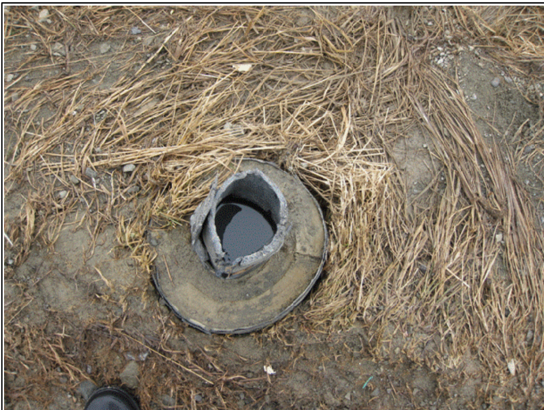
Photo 40: Overflowing sewage in observation pipe on the drainfield serving the Washeteria, teacher housing, and school.
