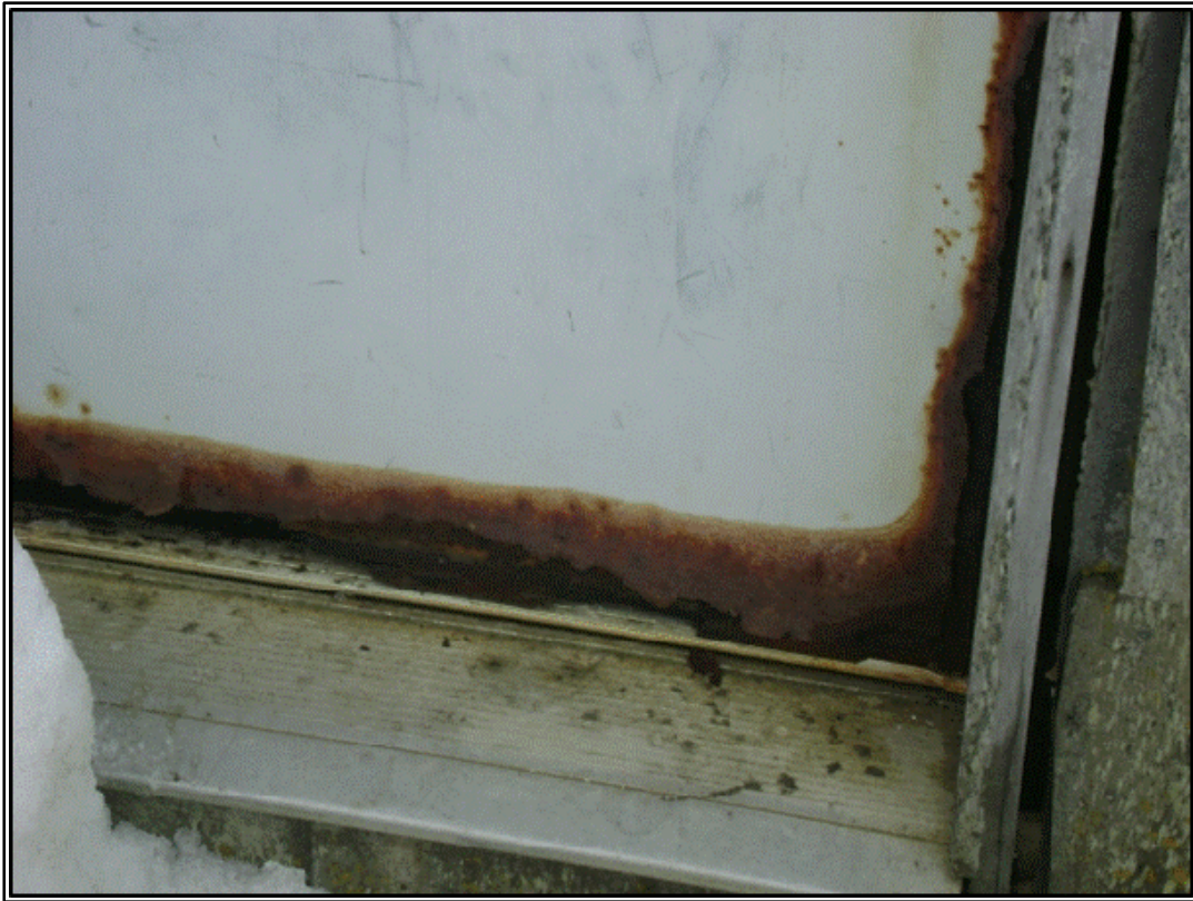
Photo 21: Bottom of Watering Point #5 door. Corrosion is typical of most watering points.
