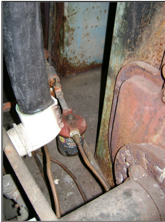
Photo 11: Boiler 2 burner showing firebox leakage and melting of combustion air inlet piping.
