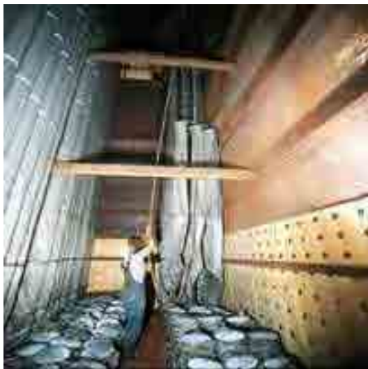
Figure 4-1. Photograph of fabric filter compartment with filter bags [Source: www.hamon-researchcottrell.com ]
