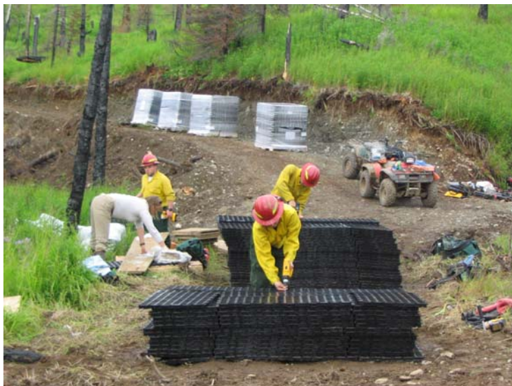
Figure 1: 7/22/2008; Div. of Forestry Interns help stage geoblock on newly graded trail reroute near Grandpa's Water Hole
