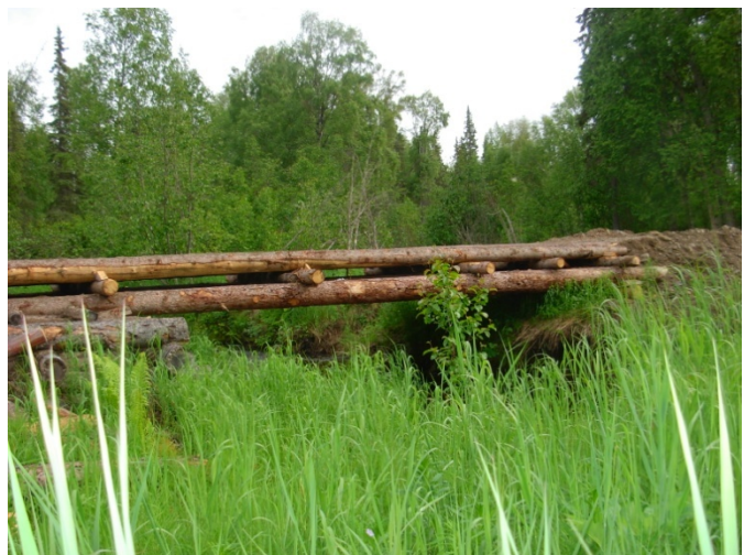
Photograph 3. ATV bridge across Chijuk Creek at Oilwell Road.
