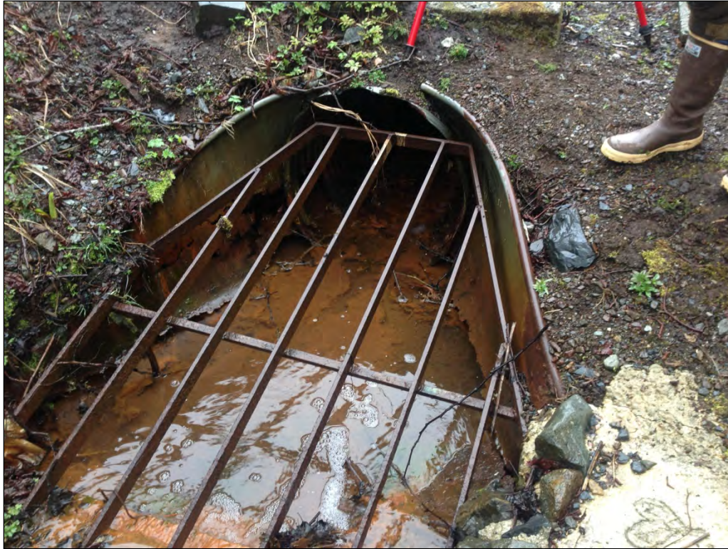
Figure E-24. Erosion of CMP invert at culvert inlet near 1602 Davidoff Street.
