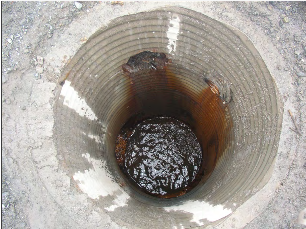
Figure E-23. Poor condition CMP manhole riser at 1601 Davidoff Street.
