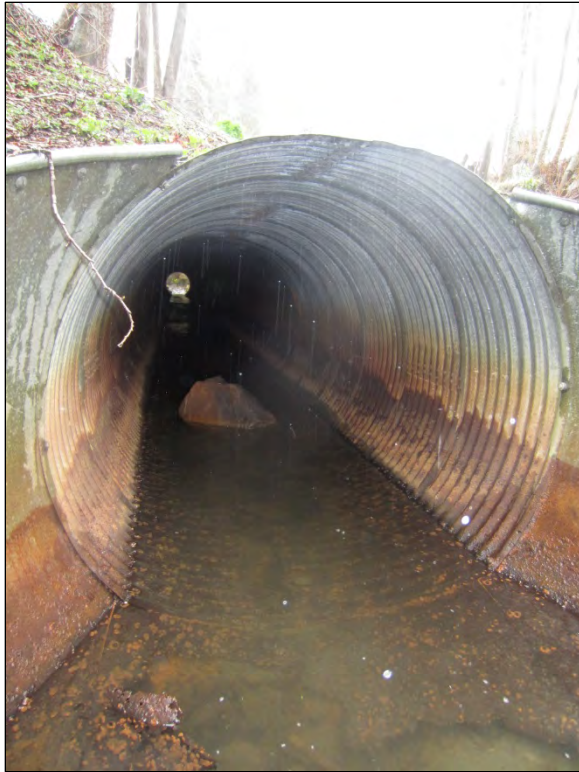
Figure E-35. Looking upstream at inlet of 60-inch CMP crossing Peterson Avenue.
