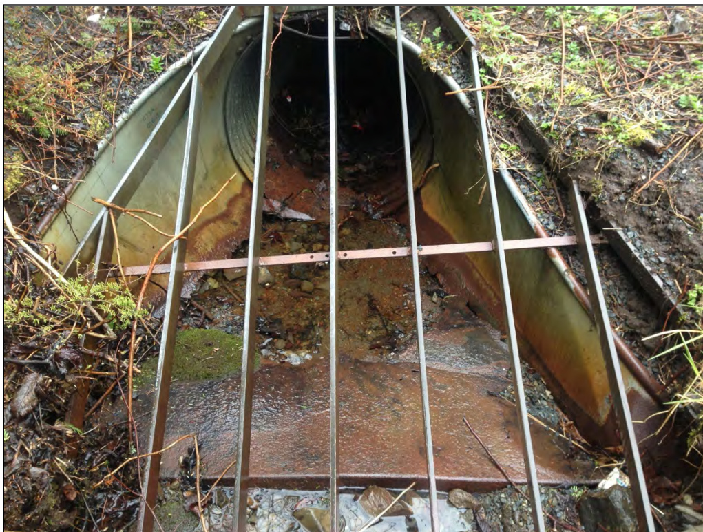
Figure E-27. Erosion of CMP invert at 306 Charteris Street.
