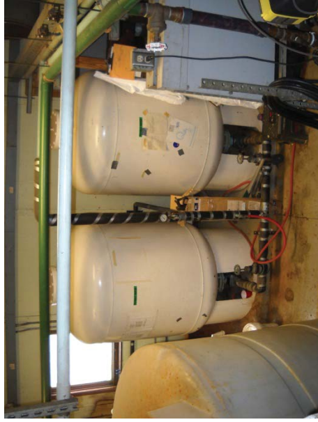
Pressure Tanks (backwash surge tank on left foreground)
