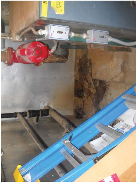
Leaky (glaciated) wastewater line from WTP/Washeteria (notice iron content in filter backwash water).
