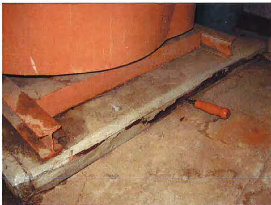
Photo No. 16: Boiler Room – Wood platform supporting hot water tank
