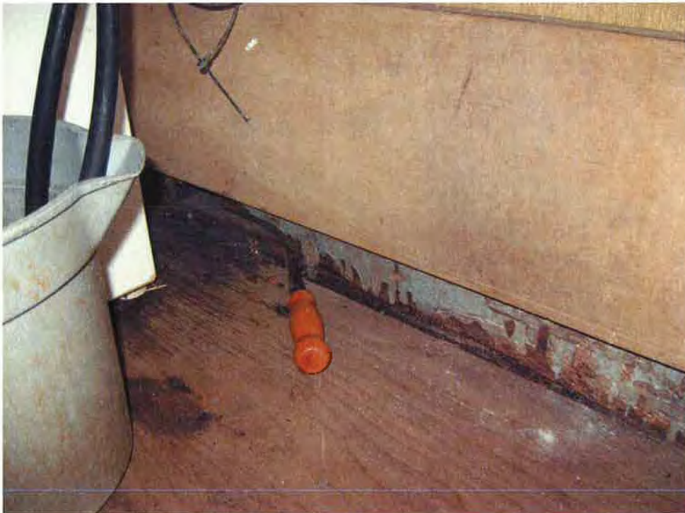
Photo No. 14: Washeteria - Rot at base of wall separating Washeteria and Boiler Room
