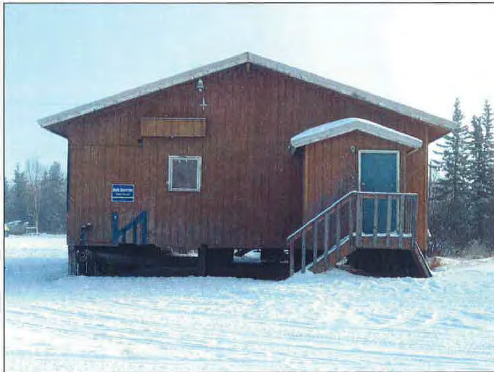
Photo No. 3: West Elevation Note: Non-compliant railing at stairs
