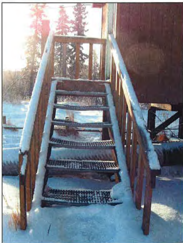
Photo No. 5: East Entry Stairs Note: 1. Non-compliant railing 2. Damaged stair treads
