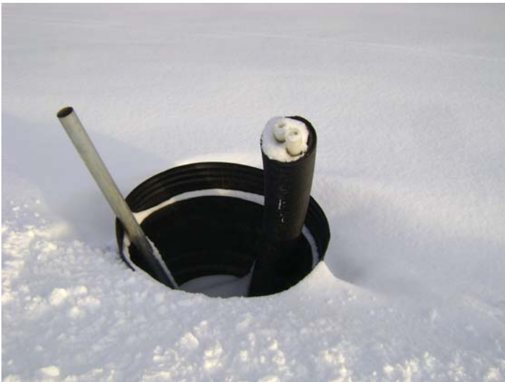
Waste Heat Piping conduit on opposite side of road from power plant.
