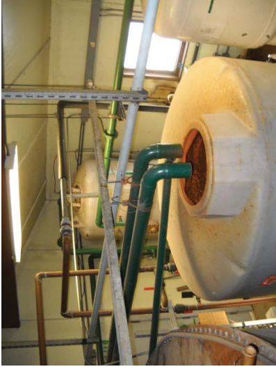
Treatment Room (cw from left, treated water tank, greensand filter, pressure tank, backwash water surge tank)
