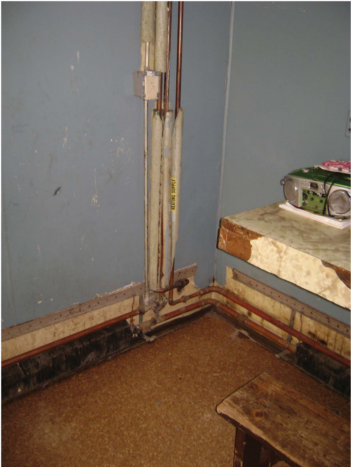
Baseboard heaters with missing covers and damaged fins.
