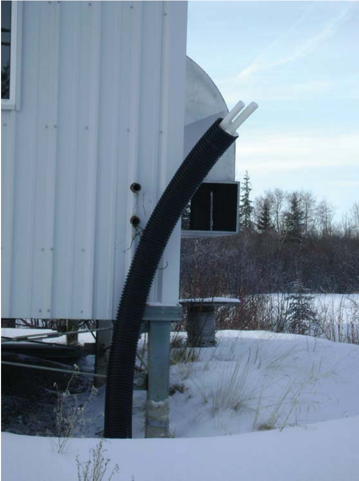
Waste Heat Piping conduit at exterior of power plant.
