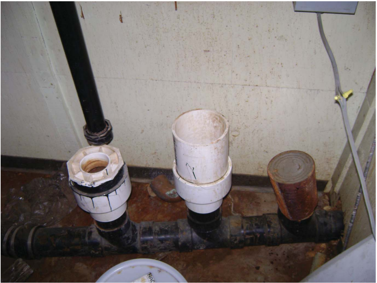
Open connections at Backwash drain line. Line is broken at exterior of building wall
