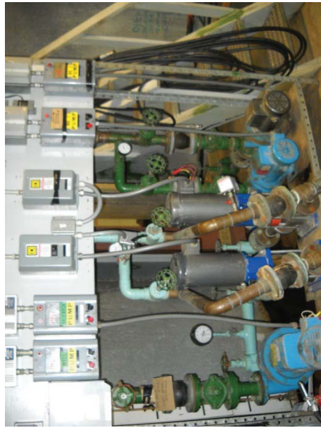
Treatment System Pump Manifold
