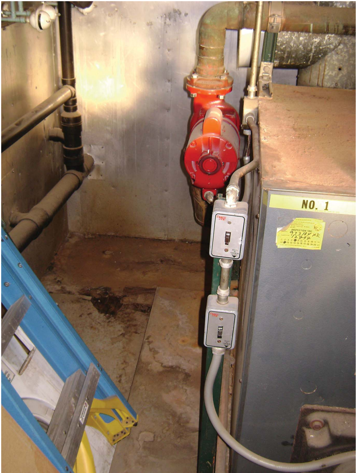
Boiler and Circulation Pump
