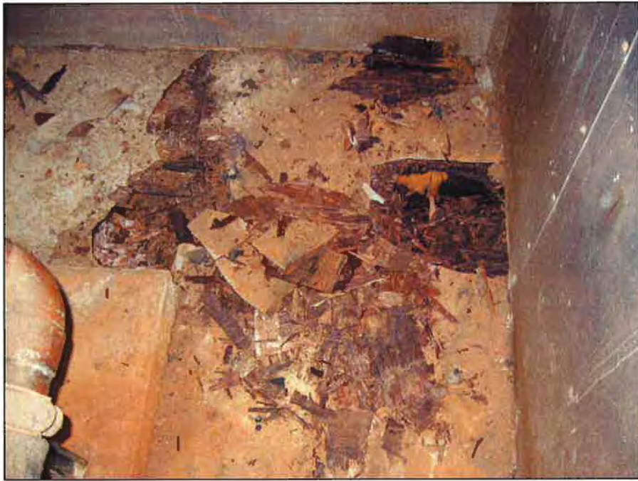
Photo No. 17: Boiler Room – Rotten plywood and joists behind Boiler No. 2
