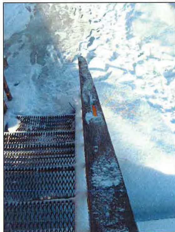
Photo No. 6: West Entry Stairs Note: Rotten stairrail
