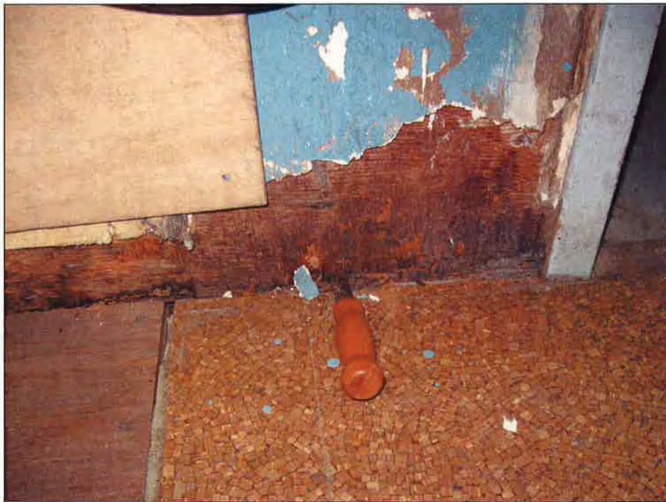
Photo No. 13: Washeteria – Rot at base of wall separating Washeteria and Boiler Room
