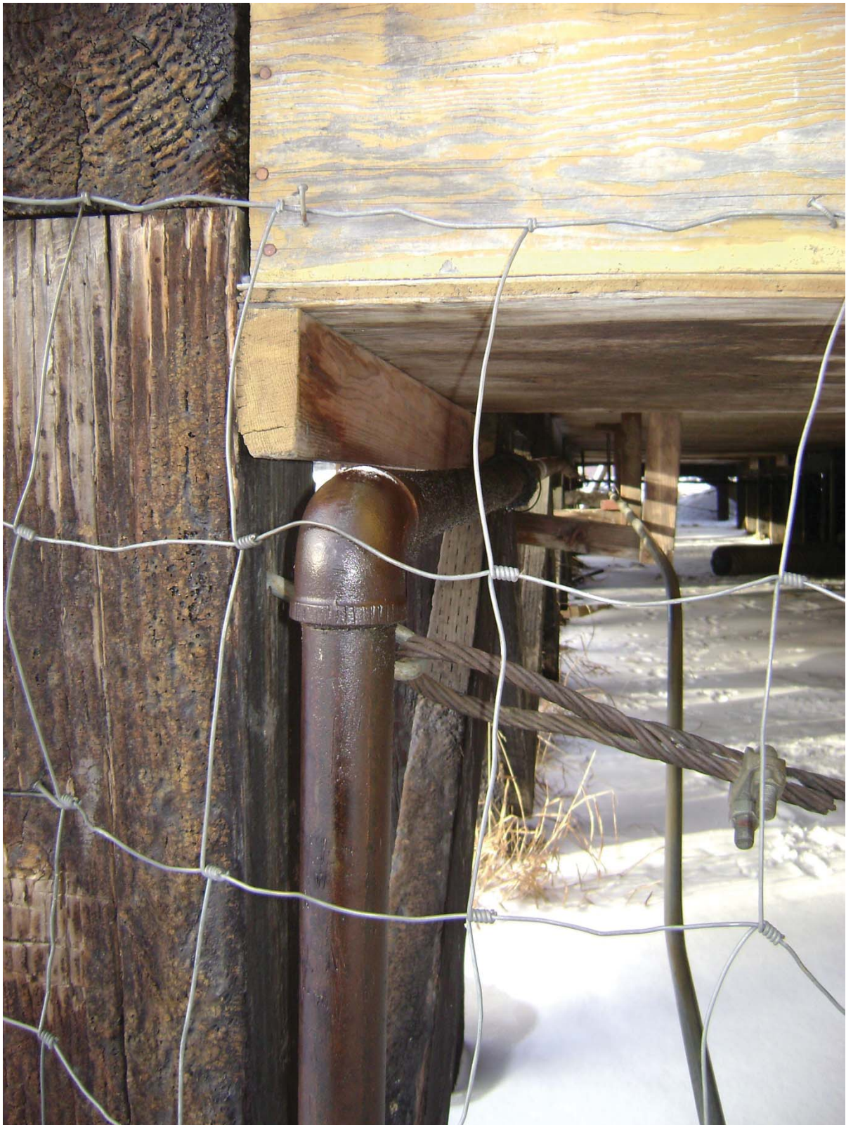
Photo of leaking fuel supply piping – Well pump is in the background to the left. Leak is at union about 4 ft from elbow.
