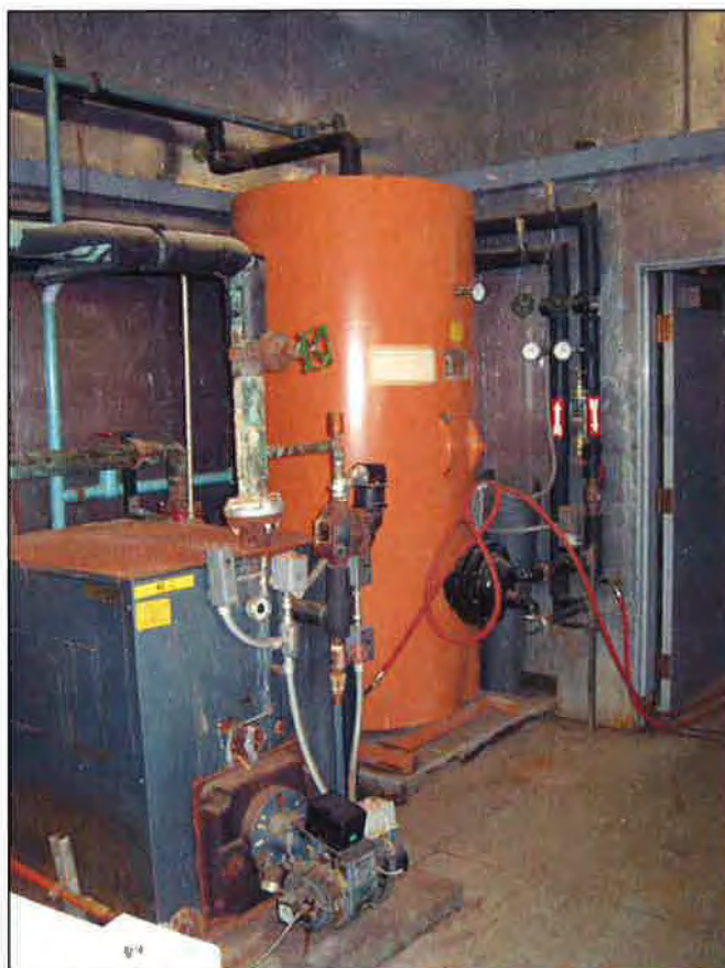
Photo No. 15: Boiler Room – Hot Water Generator
