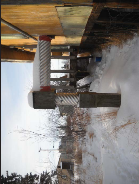
Insulated well head & piping
