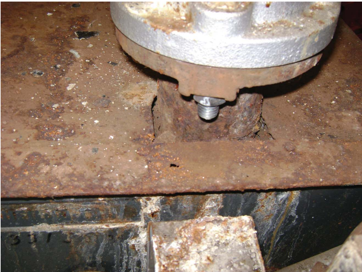
Close up of corroded boiler supply nipple.
