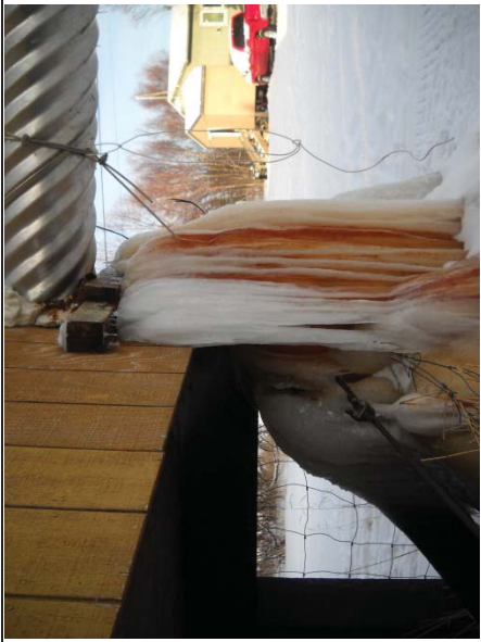
Leaky (glaciated) wastewater line from WTP/Washeteria (notice iron content in filter backwash water).
