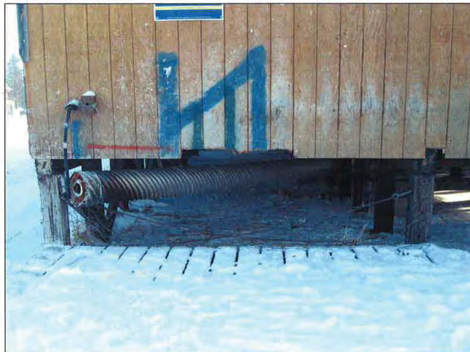
Photo No. 4: West Wall Note: 1. Missing trim from corner of building 2. Cable bracing not tight
