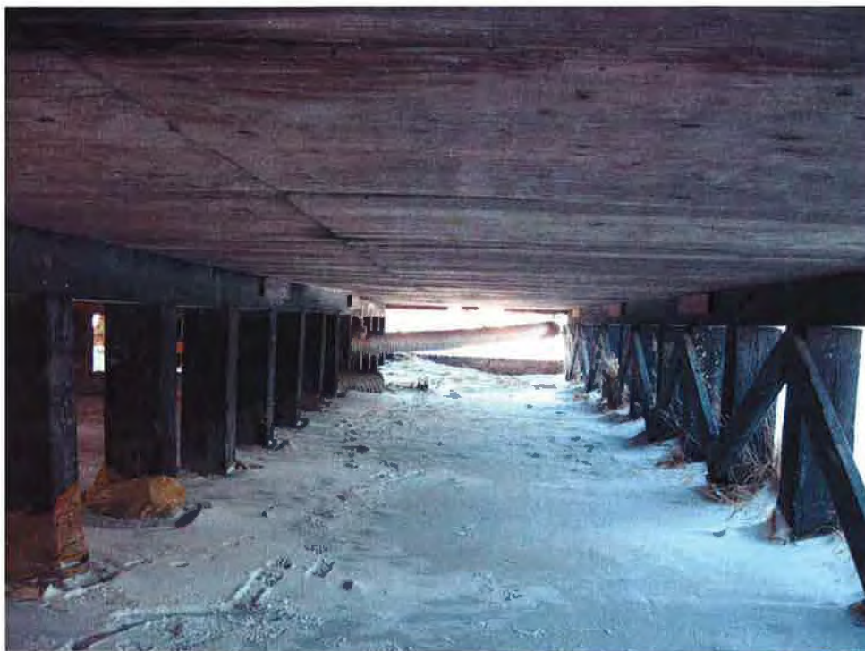
Photo No. 9: Post and Beam Foundation
