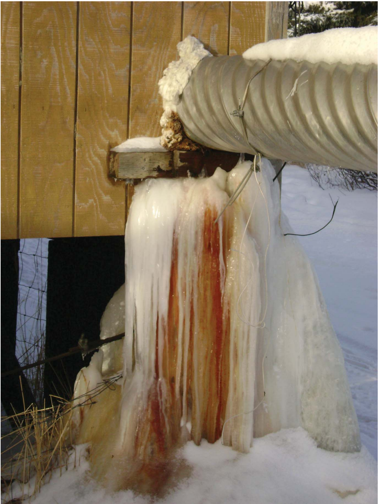
Leak at backwash drain piping from outside.
