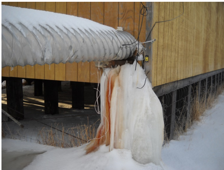
Photo 3 – Leaking WTP Backwash Line
