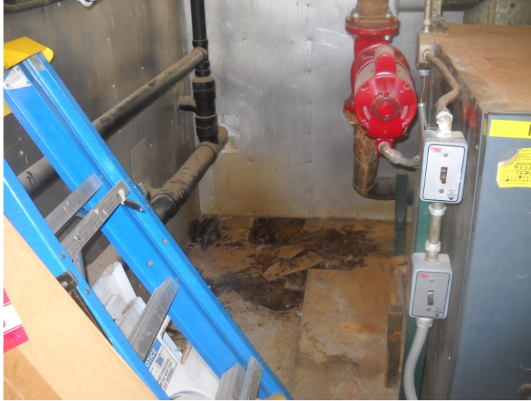
Photo 1 – Rotting Floor near Boilers
