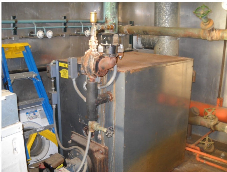
Photo 2 – Corrosion Damage on Boiler and Piping
