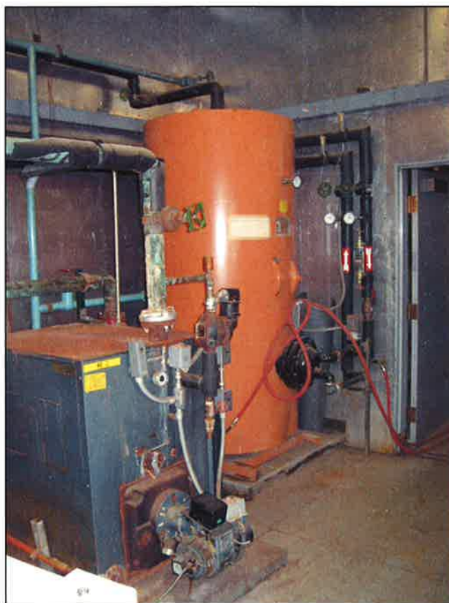
Photo No. 15: Boiler Room – Hot Water Generator
