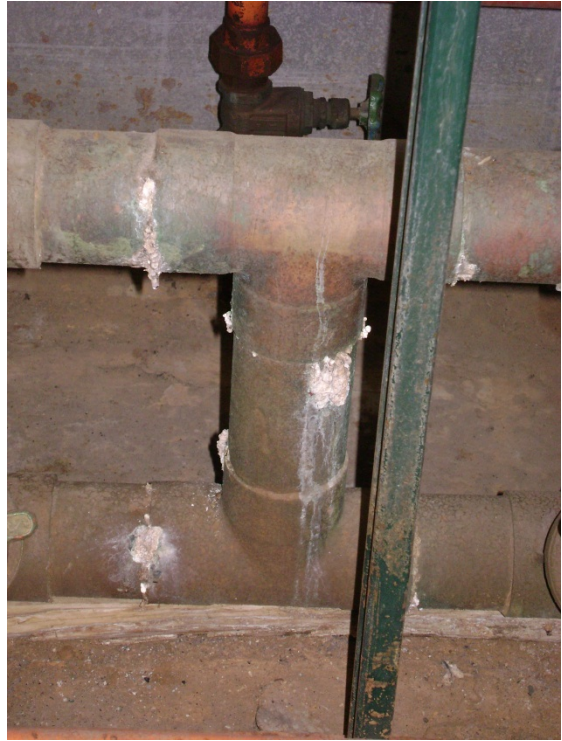
Close-ups of copper boiler piping with corroding, leaking joints
