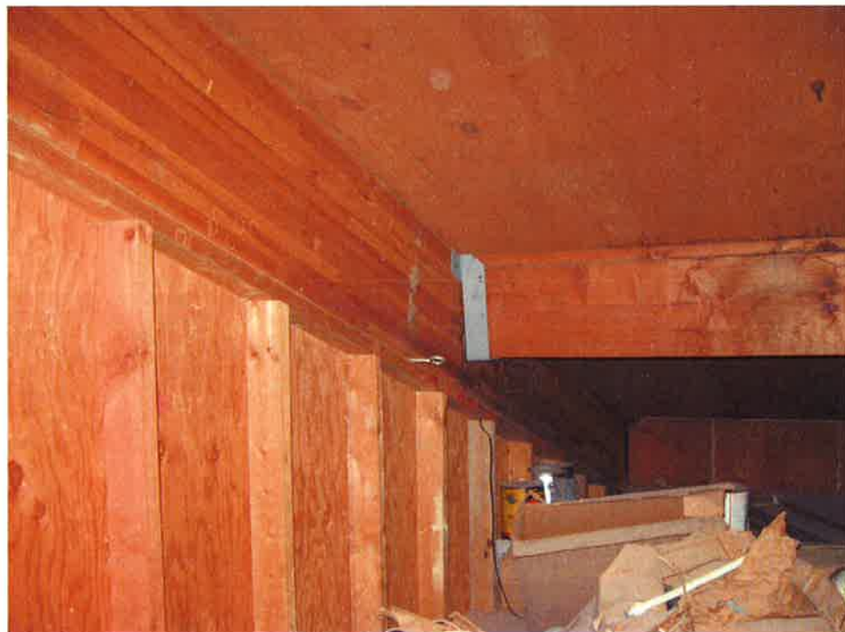
Photo No. 10: Typical Roof Framing
