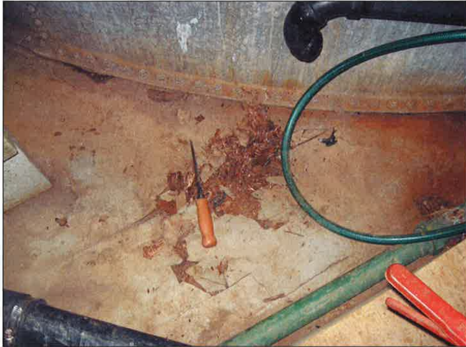
Photo No. 19: Water treatment tank – rotten plywood adjacent to tank
