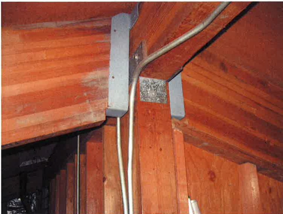
Photo No. 11: Roof Framing Note: Dapped GLB at connection
