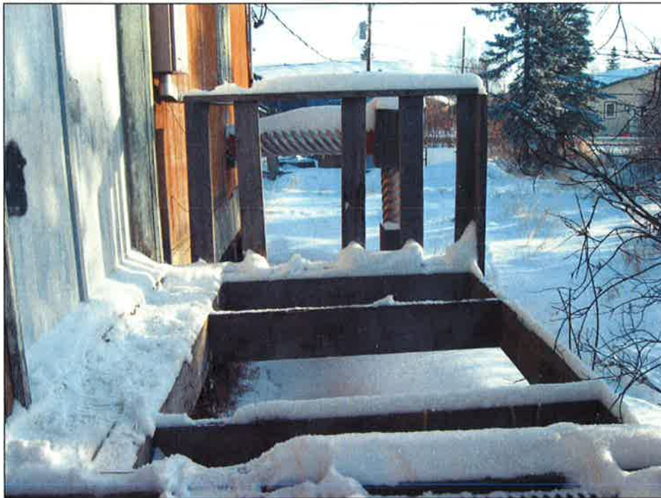
Photo No. 8: Landing on South Wall Note: No decking creates potential safety hazard
