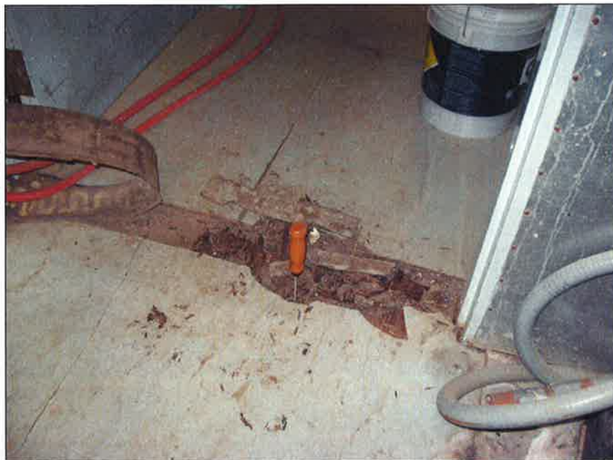
Photo No. 18: Boiler Room – Rotten sill at door between Boiler Room and Treatment Room
