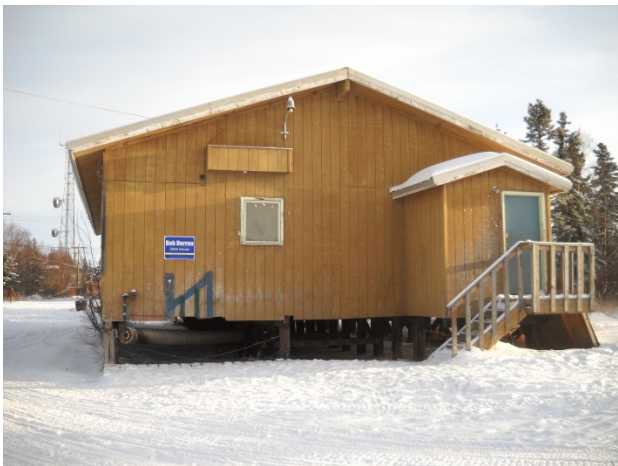
WTP/W Bldg (SE corner, notice insulated well head & piping)
