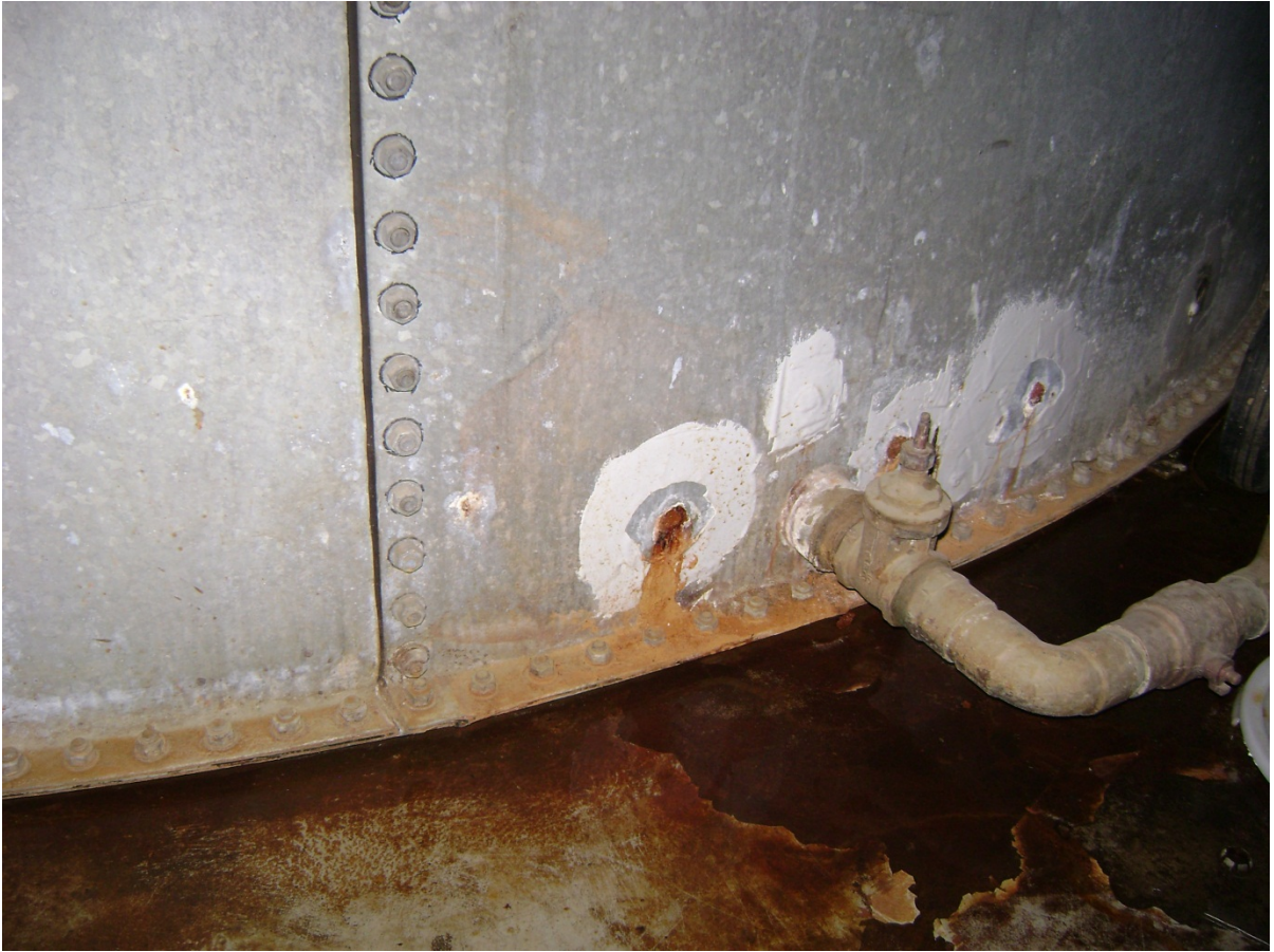
Treated water tank corrosion. Tank has been lined, but water still appears on floor underneath
