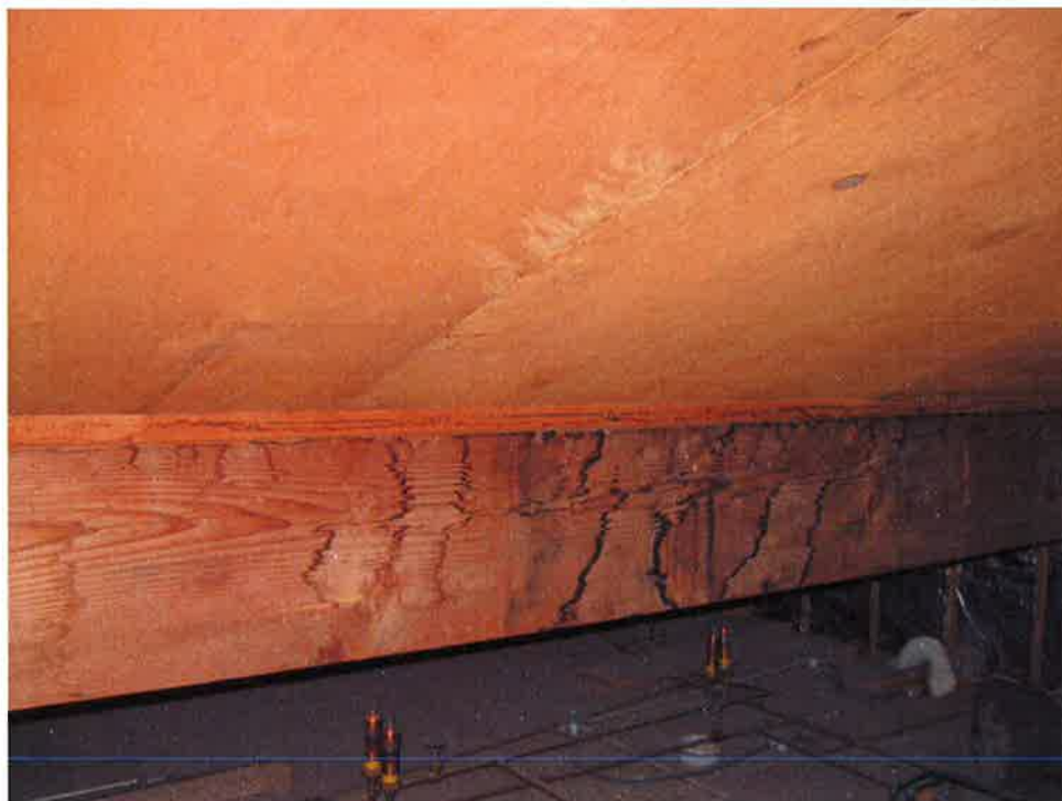
Photo No. 12: Roof Beam Note: Water stains on beam
