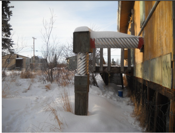
Insulated well head & piping
