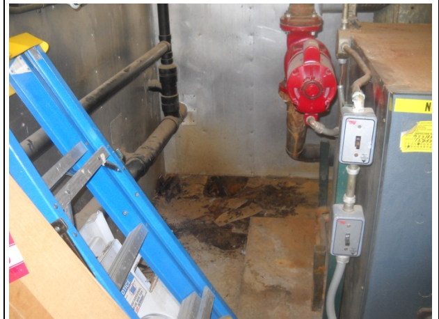
Leaky (glaciated) wastewater line from WTP/Washeteria (notice iron content in filter backwash water).
