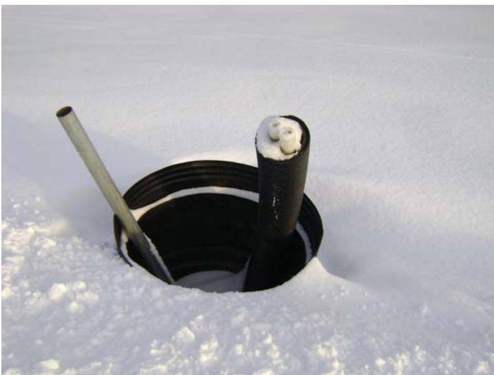
Waste Heat Piping conduit on opposite side of road from power plant.
