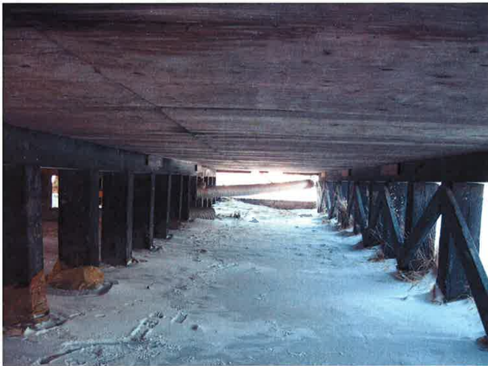
Photo No. 9: Post and Beam Foundation
