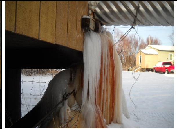
Leaky (glaciated) wastewater line from WTP/Washeteria (notice iron content in filter backwash water).
