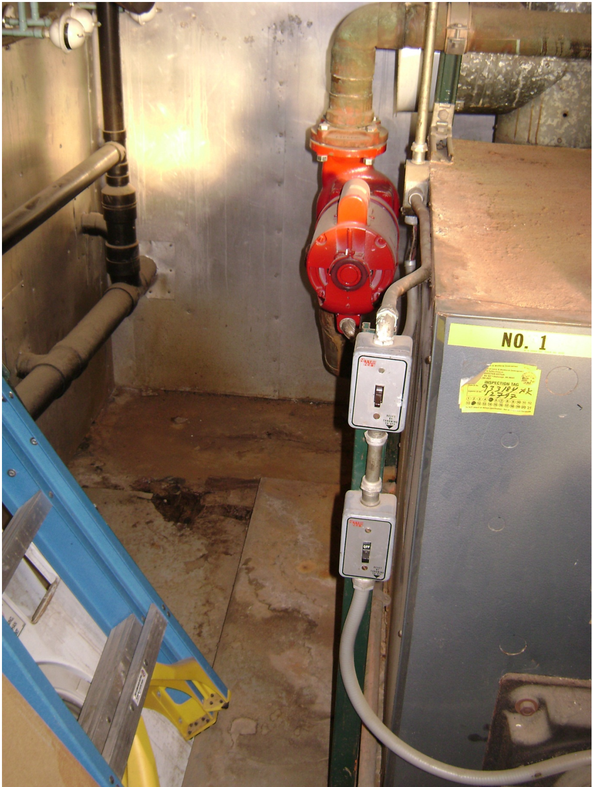
Boiler and Circulation Pump
