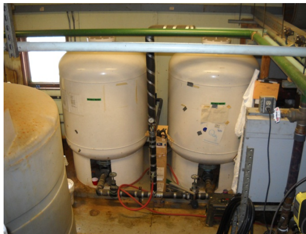
Pressure Tanks (backwash surge tank on left foreground)
