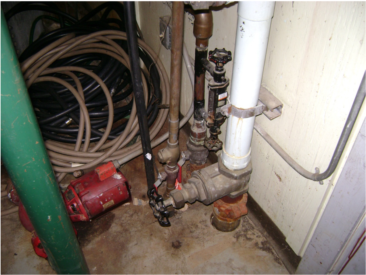
School and Work Camp (smaller) water lines thru floor. Raw water tank drain line pump at left.
