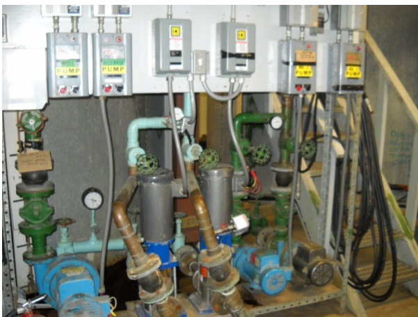
Treatment System Pump Manifold
