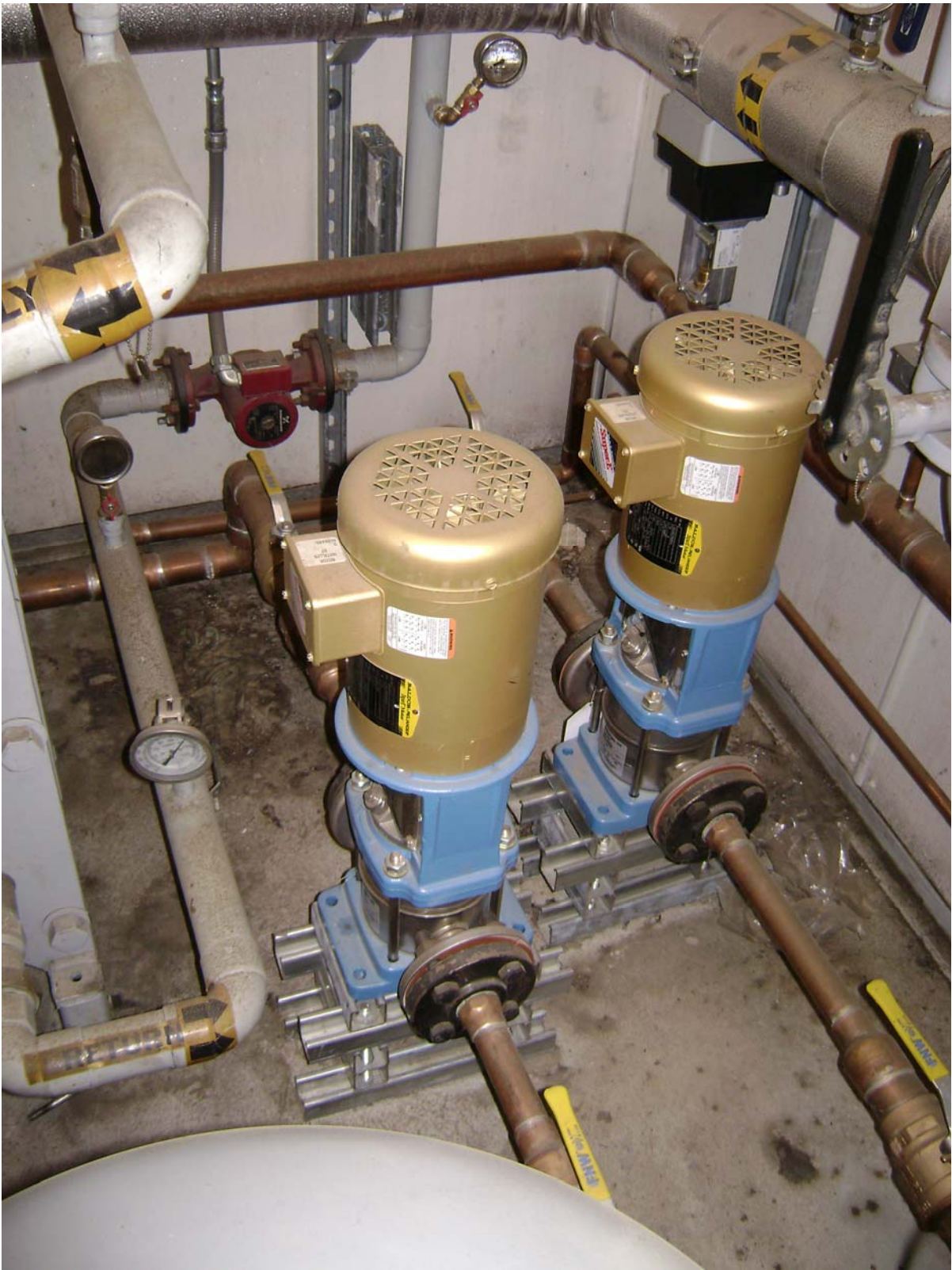
Circulation pumps for Waste Heat supply. Note pumps and control valve at upper right not connected to power. Pump in background is hot side circulator for heat exchanger.
