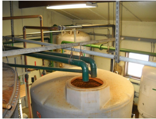
Treatment Room (cw from left, treated water tank, greensand filter, pressure tank, backwash water surge tank)
