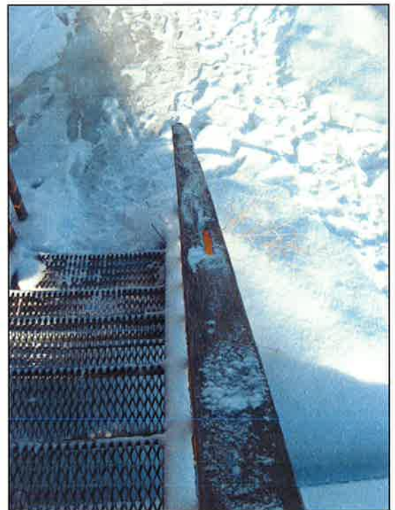
Photo No. 6: West Entry Stairs Note: Rotten stairrail
