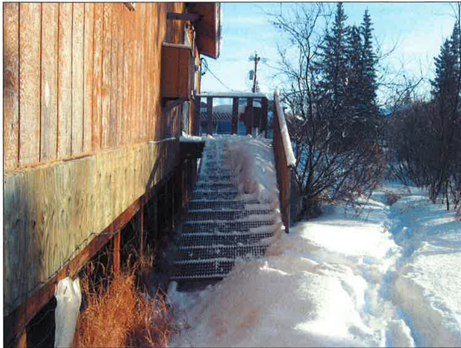
Photo No. 7: Ramp on South Wall Note: Non-compliant Railing
