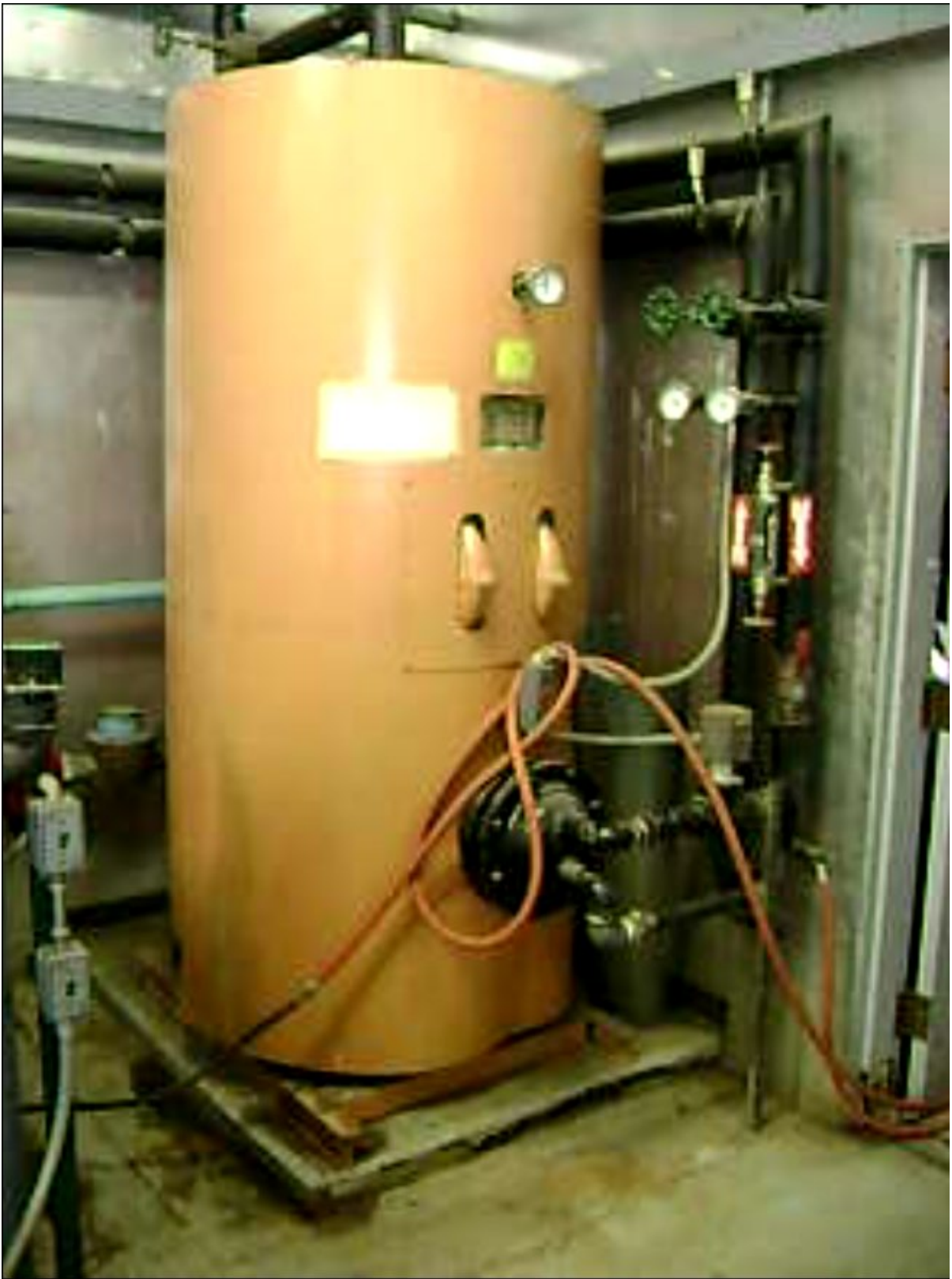
Domestic Water heater with original single wall heat exchanger bundle.
