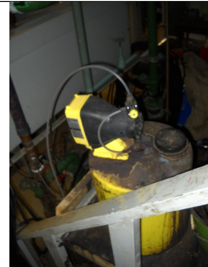
Potassium Permanganate Tank
