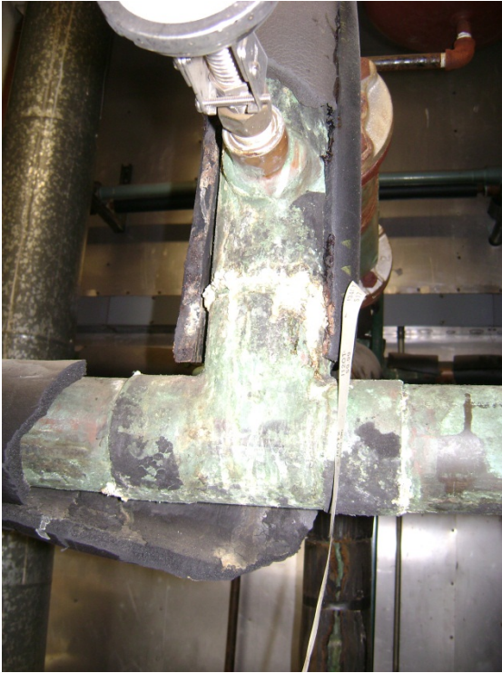
Close-ups of copper boiler piping with corroding, leaking joints
