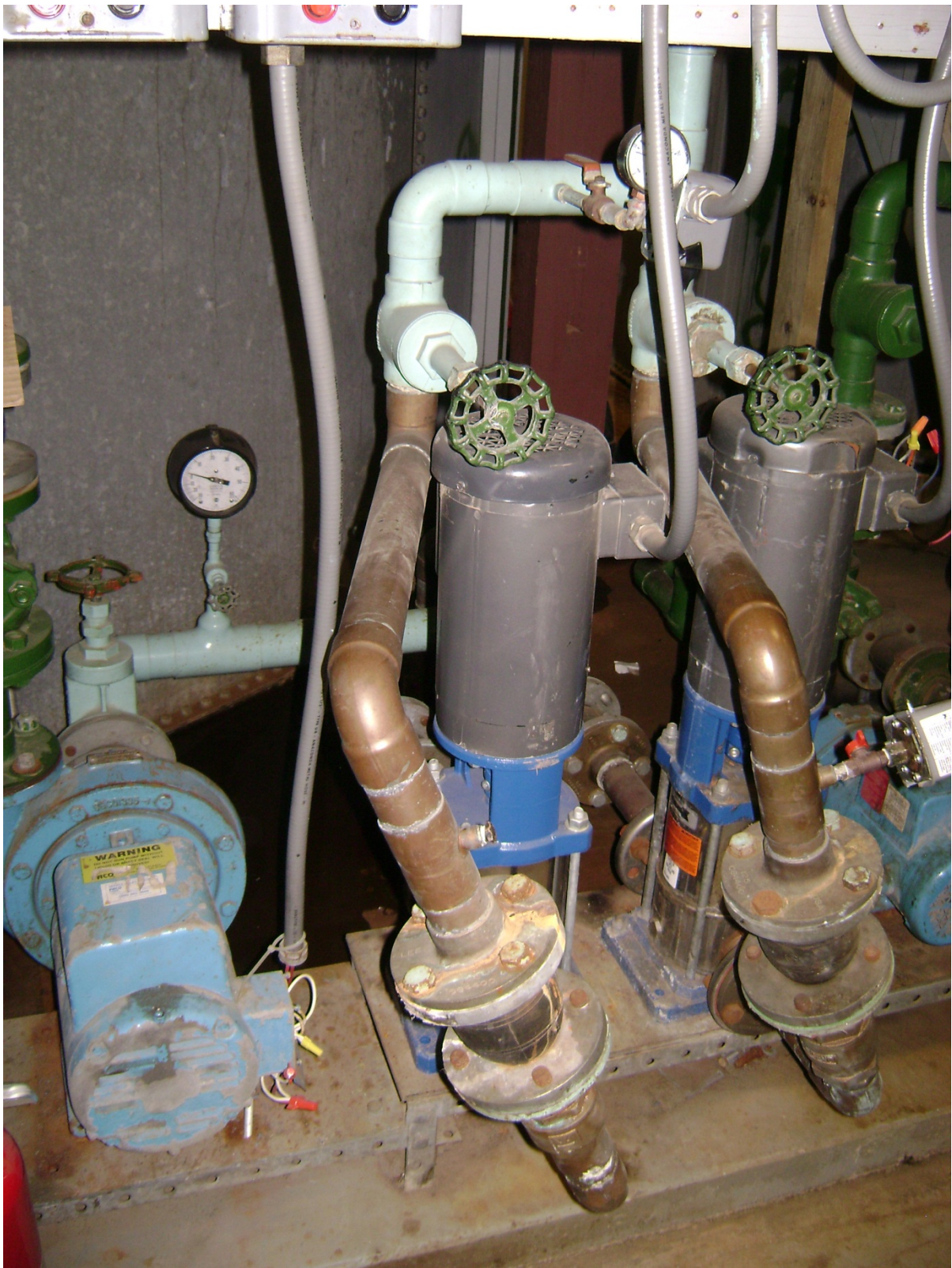
Pressure pumps (right two). One is not working. Note piping obstructing pump maintenance.
