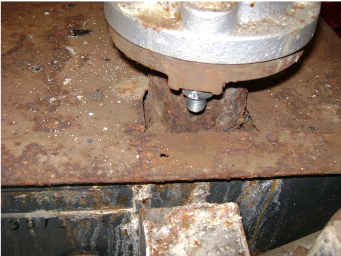
Close up of corroded boiler supply nipple.
