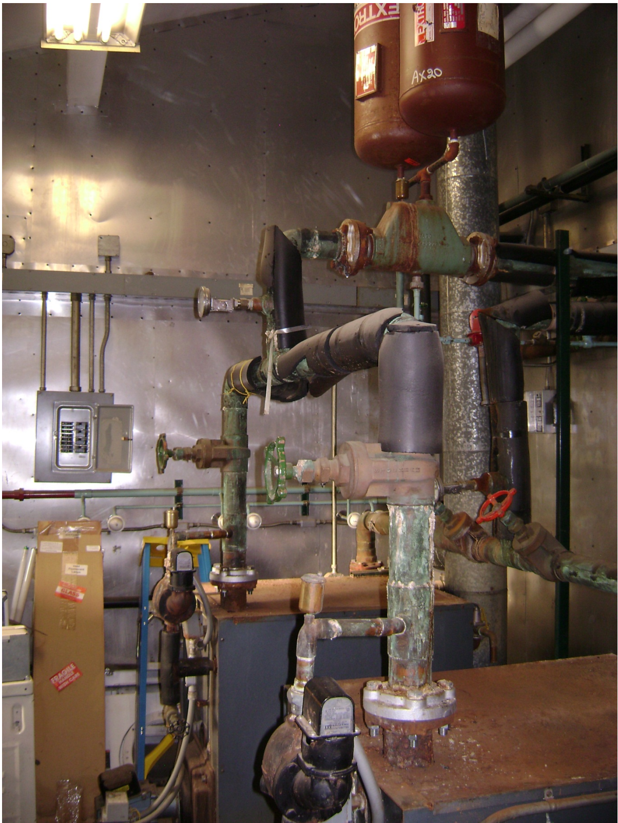
View of Boilers with leaking piping and deteriorated piping insulation
