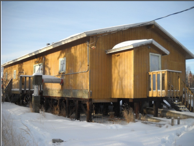
WTP/W Bldg (SE corner, notice insulated well head & piping)
