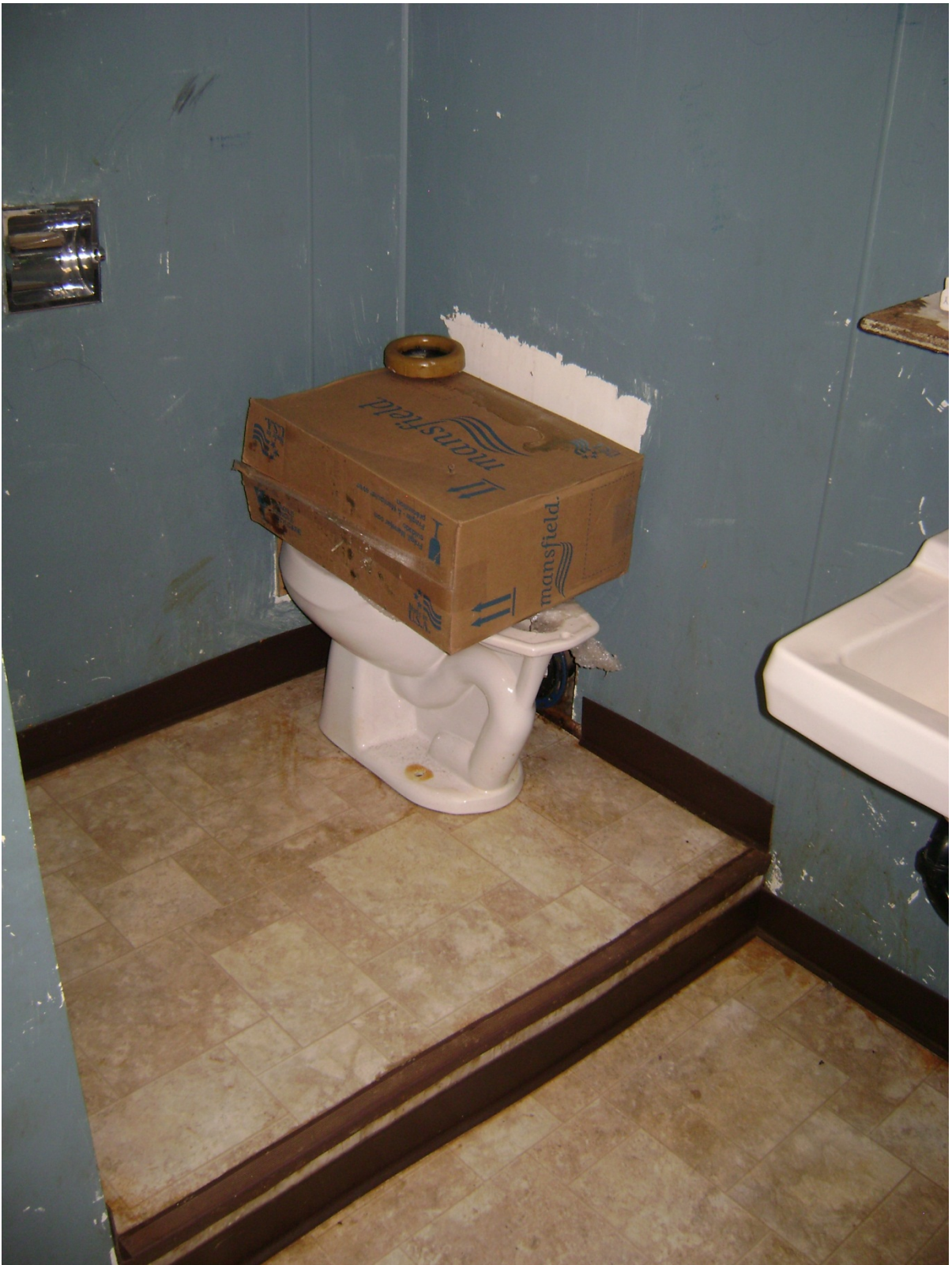
Typical Toilet/Shower room. Toilets not connected.
