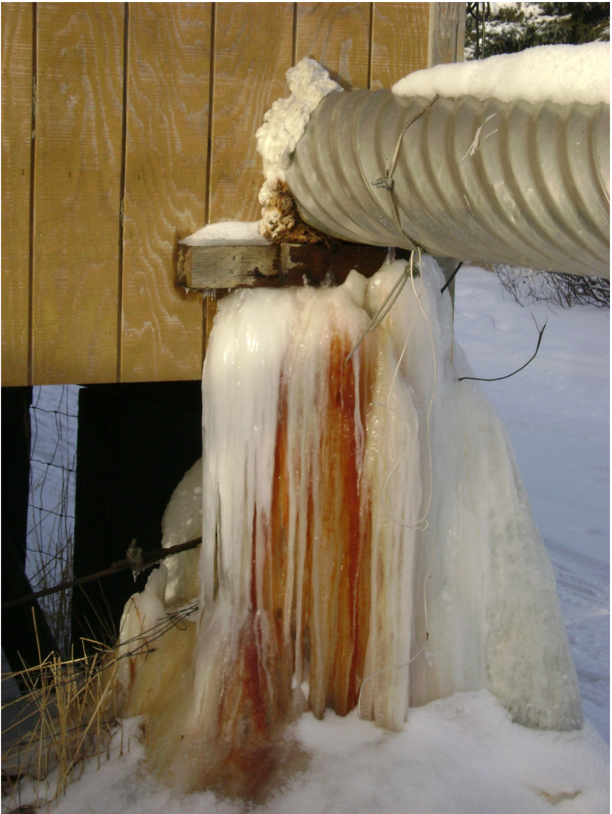
Leak at backwash drain piping from outside.
