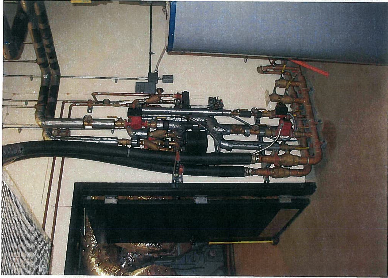
Fig 1 Distribution Manifold from Wood Heat Loop to Loads, in boiler room,
