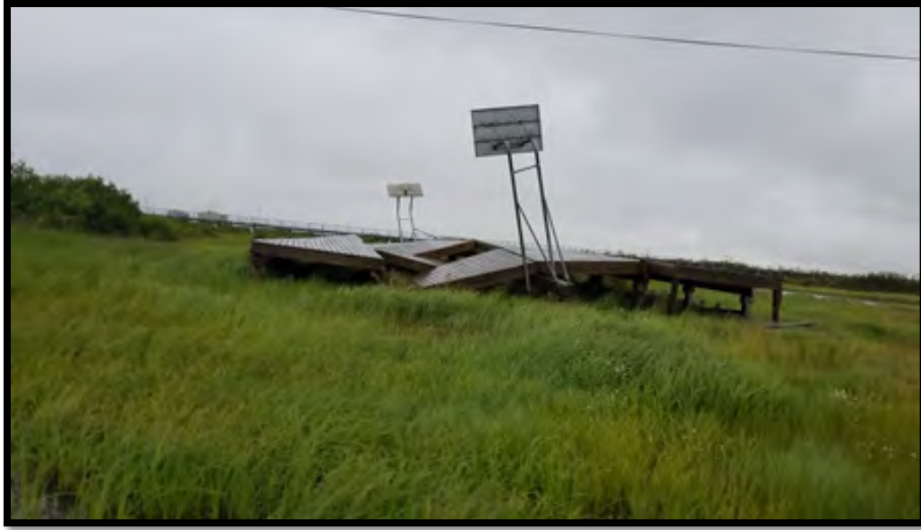
Figure 15: Basketball court, damaged from heavying and settling.
