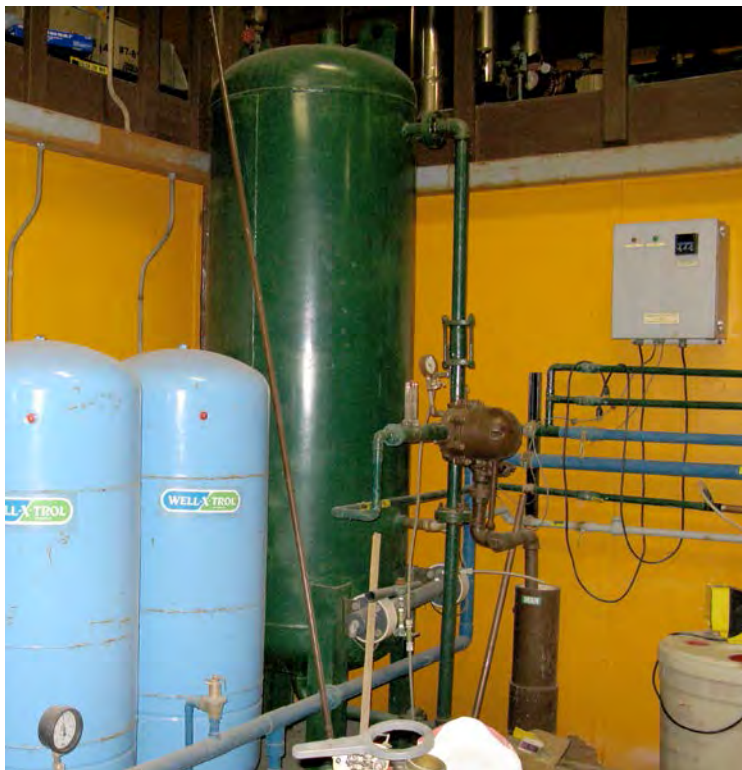
Figure 8 - Existing Greensand Filter and Piping
