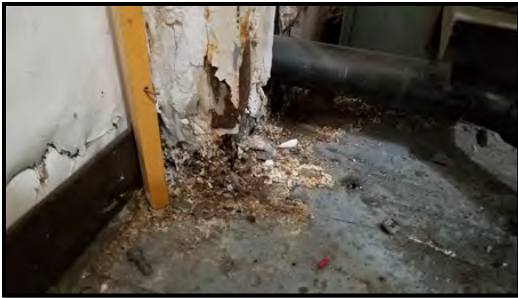
Figure 6: Water damage behind dryers in washeteria
