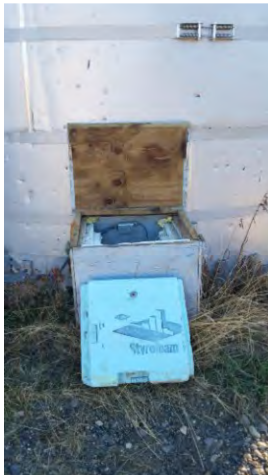
Figure 23: Typical Perimeter Pile, Beginning to Fail, Leans Towards Depression Figure 24: Water Storage Tank-Exterior Valve Box
