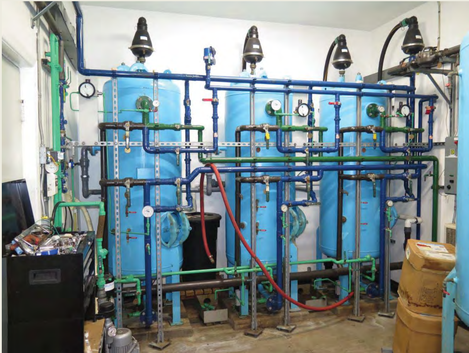
Photo 16: Greensand filters. Raw water piping in green; filter effluent in blue, backwash dark brown piping. Air scour piping in light green.
