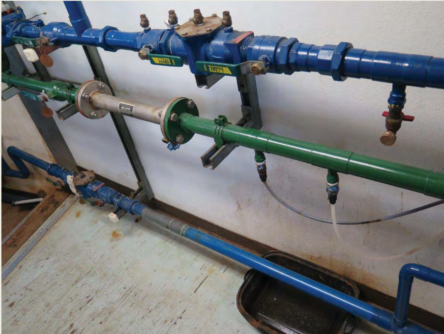
Photo 39: distribution system piping, showing backflow preventers on all lines (truck fill line backflow preventer on top; combined washeteria/school/multipurpose building lines at bottom)
