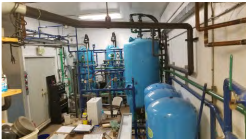
Figure 25: WTP Filters, Settling Tank, and Pressure Tanks
