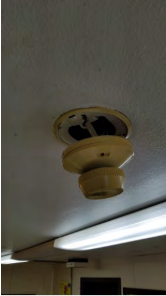
Figure 38: Laundry-Nonfunctioning Smoke Alarm
