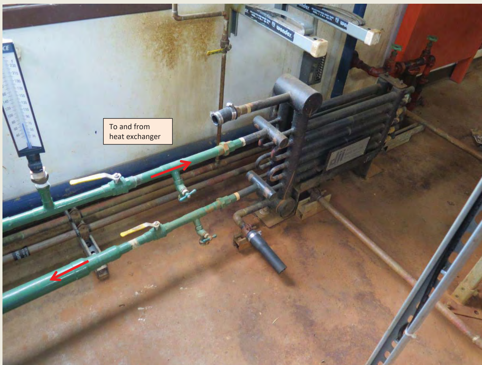
Photo 11: Raw water line heat exchanger (meant to raise temperature to improve oxidizer performance). No longer functional – disconnected from glycol supply.
