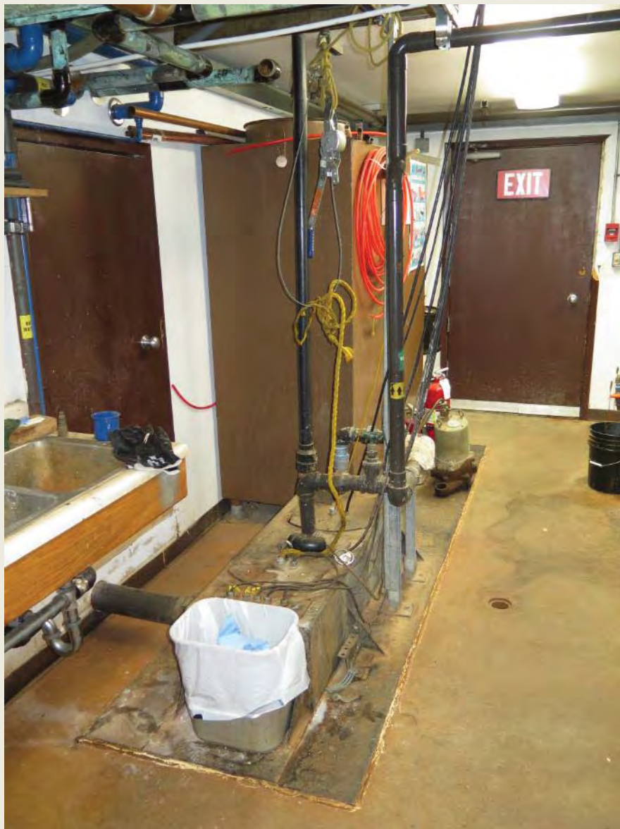
Photo 19: Washeteria lift station, with backwash detention tank in background..
