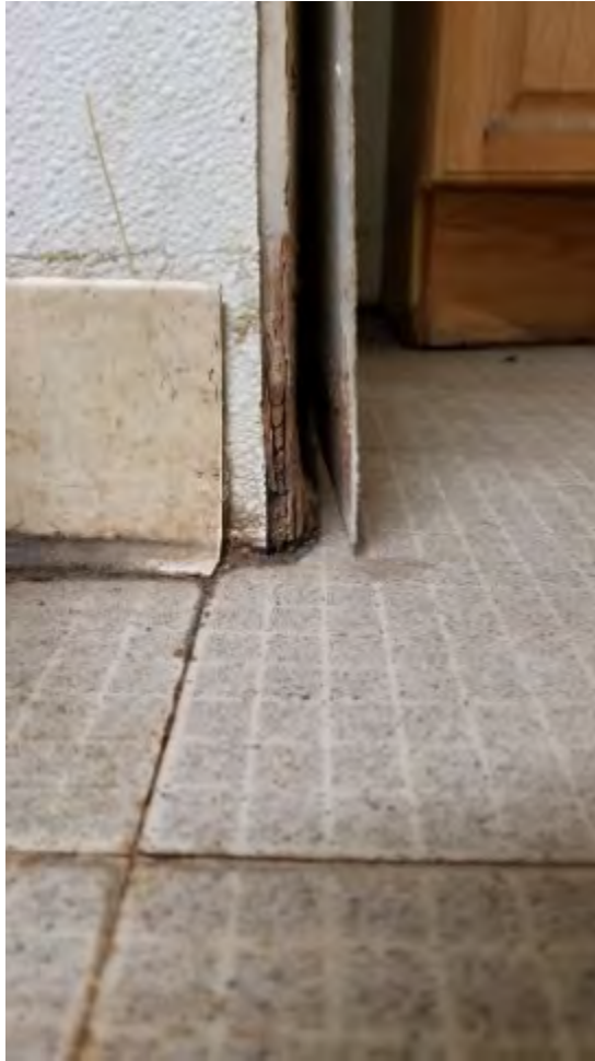
Figure 37: Bathroom-Wall Separation, Plywood Delamination
