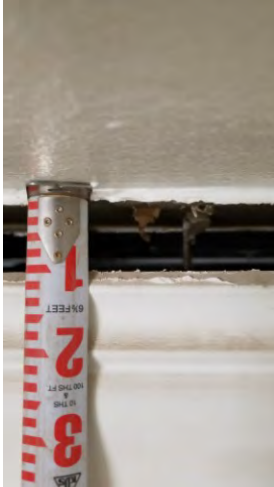
Figure 35: Bathroom-Wall and Ceiling Separation
