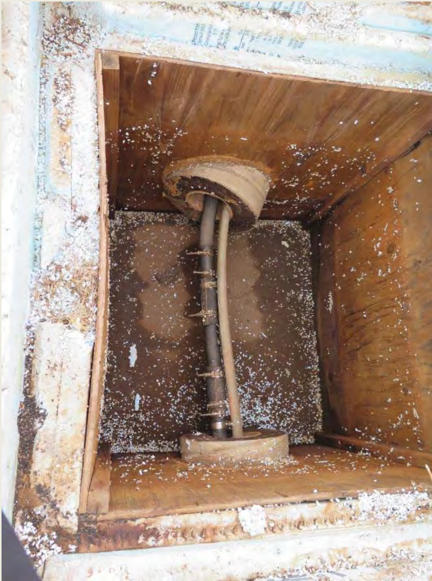
Photo 8: Raw water transmission piping (black) and glycol heat trace inside first manhole from well. Note repair couplings from previous leaks.
