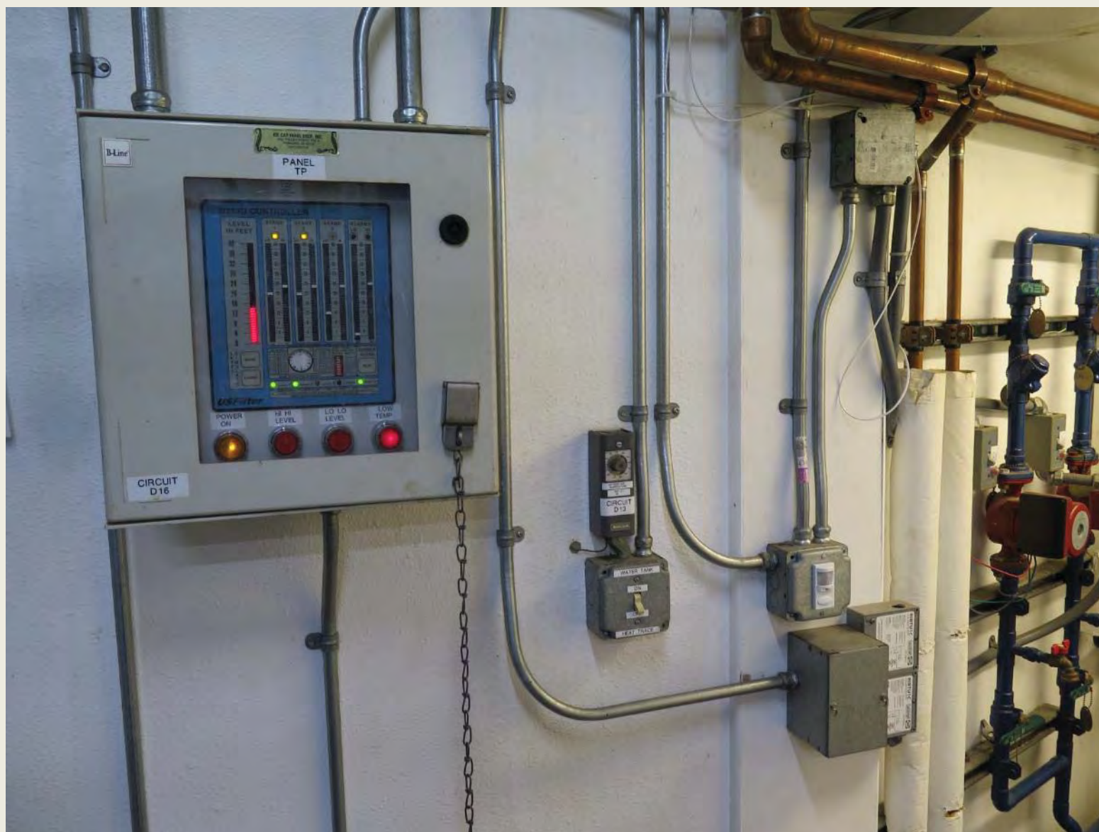
Photo 23: Digital tank level display – not functional because the suspended electrodes used for the high and low level conditions are not working and have been removed. This failure has caused the well/filtration system to only operate in hand mode. In addition, it appears the pressure transducer is not working properly, as the depth display is inaccurate.
