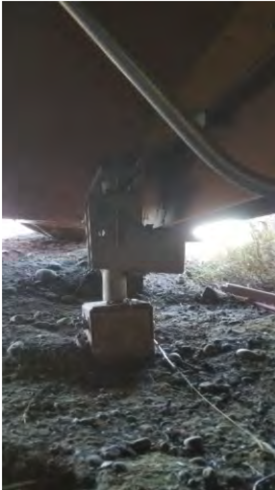
Figure 23: Typical Perimeter Pile, Beginning to Fail, Leans Towards Depression Figure 24: Water Storage Tank-Exterior Valve Box
