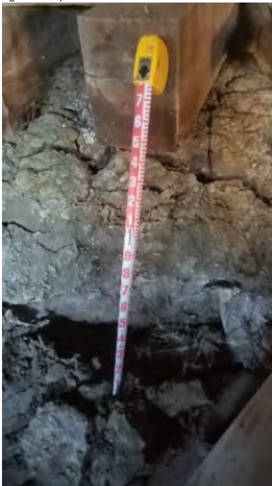
Figure 20: Soil Subsidence Under Cutting Foundation
