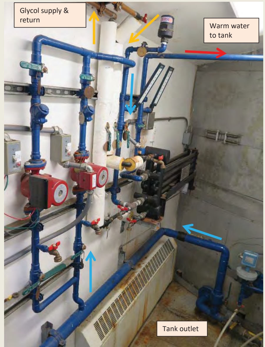
Photo 22: Storage tank finished water outlet & tank add heat system (heat exchanger not functional)
