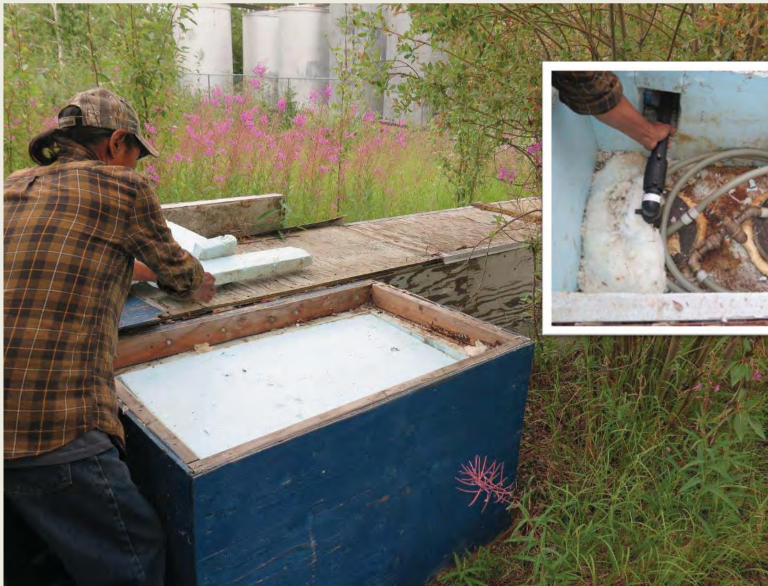
Photo 49: Point of connection to the old school utilitdor. Water main (left) and sewer force main in black HDPE; glycol heat trace piping shown coiled in box.
