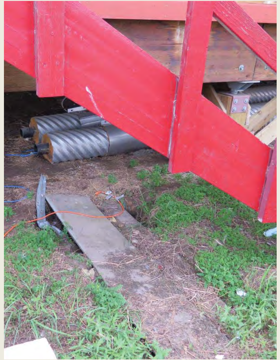
Photo 60: Another sinkhole which has appeared directly adjacent to the Beaver Multi-Purpose Building.
