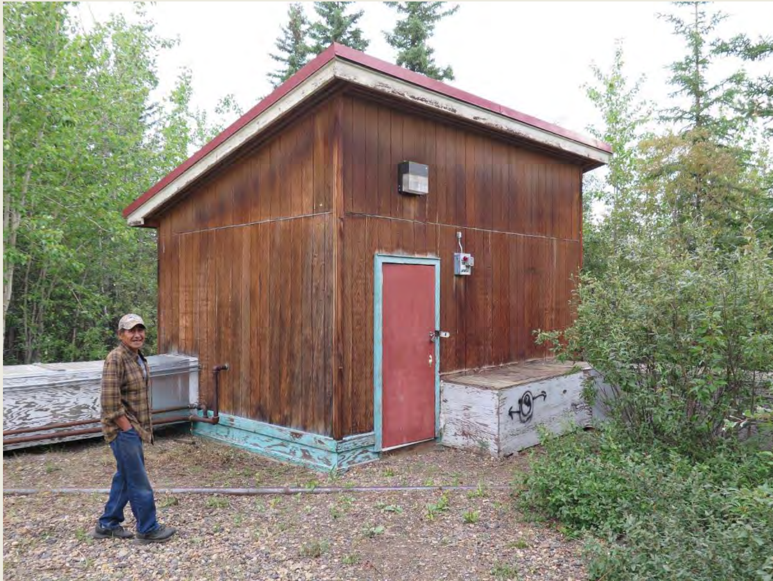
Photo 50: Point of connection to the old school utilitdor. Circulating water main in black HDPE; glycol heat trace piping shown coiled in box.
