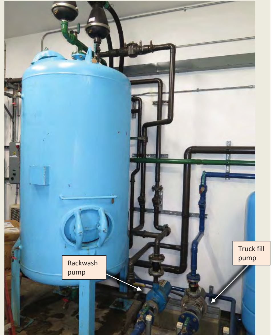
Photo 35: Truck fill & backwash pumps
