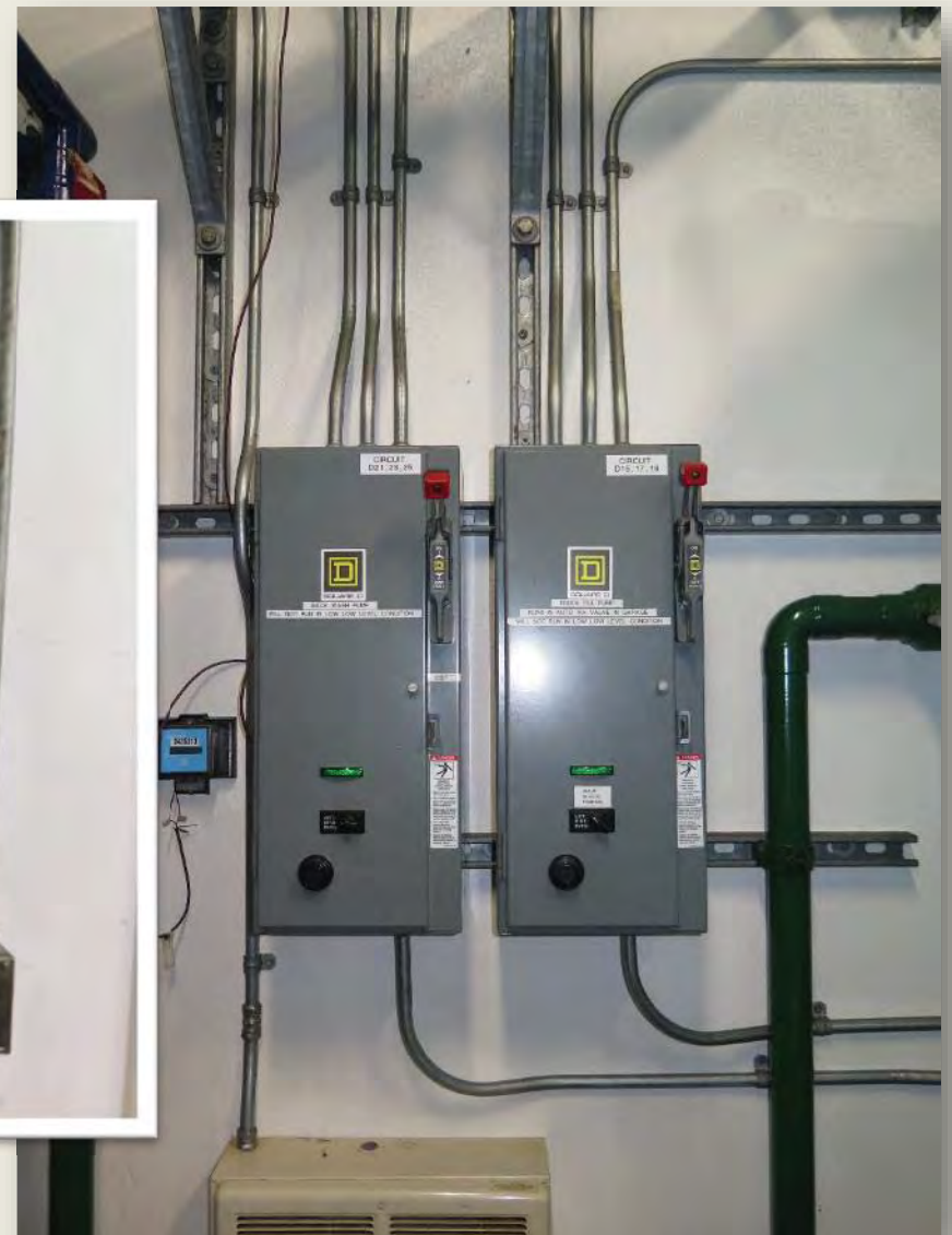
Photo 56: Backwash and Truck Fill pump control panels
