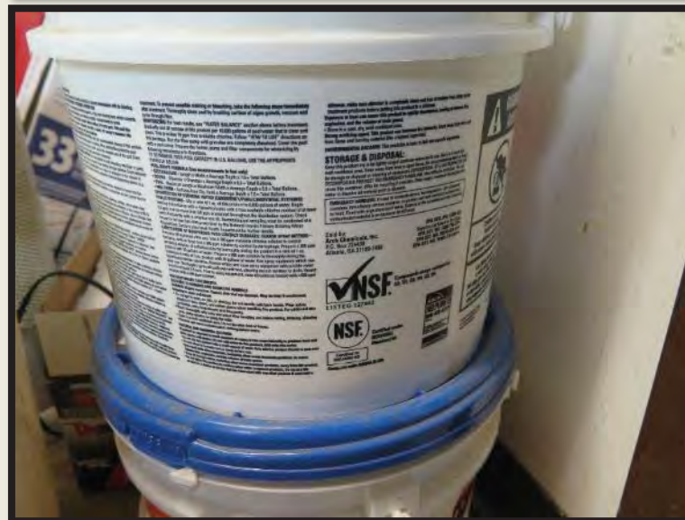
Photo 33: Potassium permanganate (2 manufacturers) and calcium hypochlorite storage.
