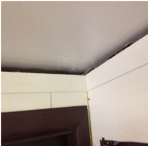
Walls separating from ceiling.
