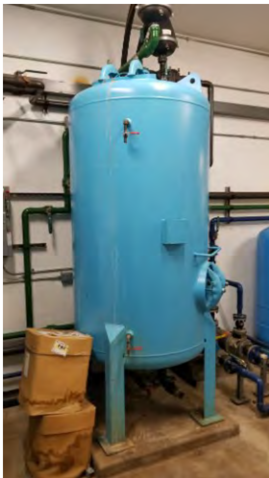
Figure 26: WTP-Settling Tank
