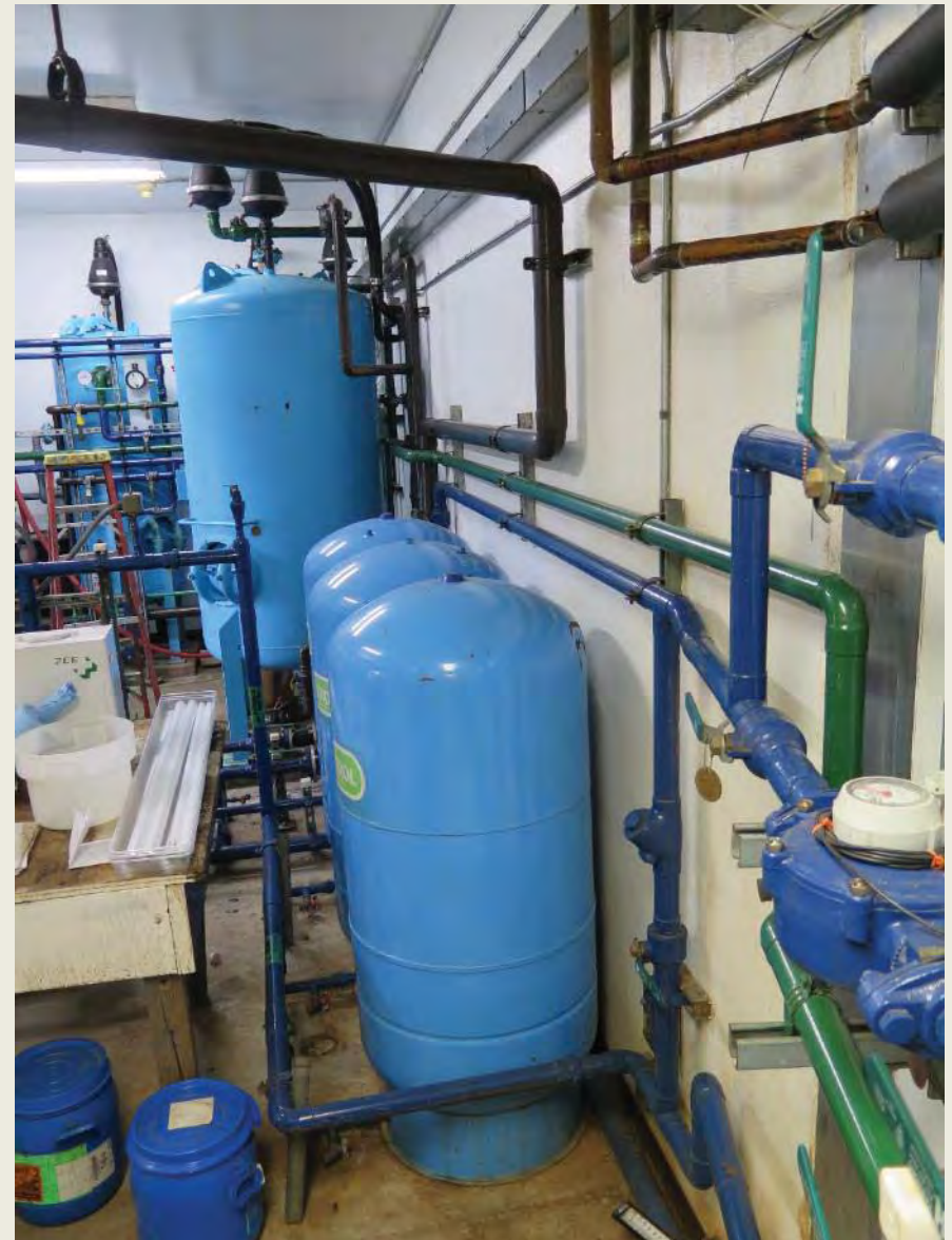
Photo 41: Pressure tanks, showing dent called out in previous sanitary survey.
