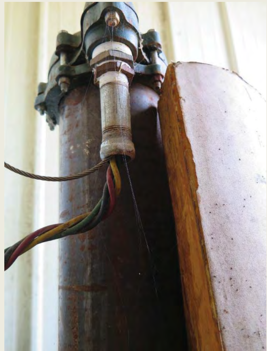
Photo 3: Well WL001, electrical power cables and conduit
