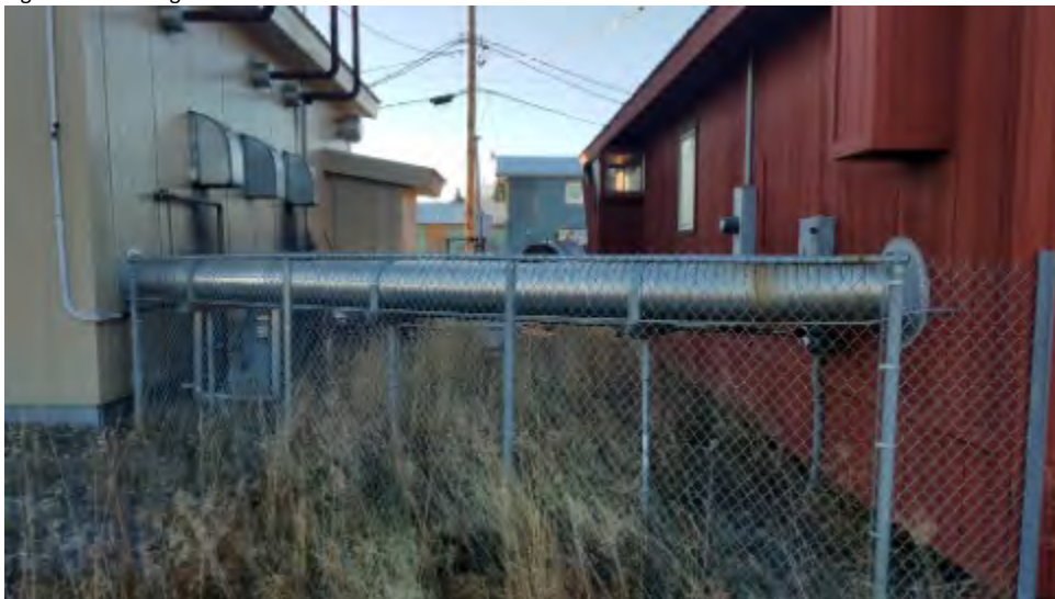
Figure 5: Power Plant Heating Pipe
