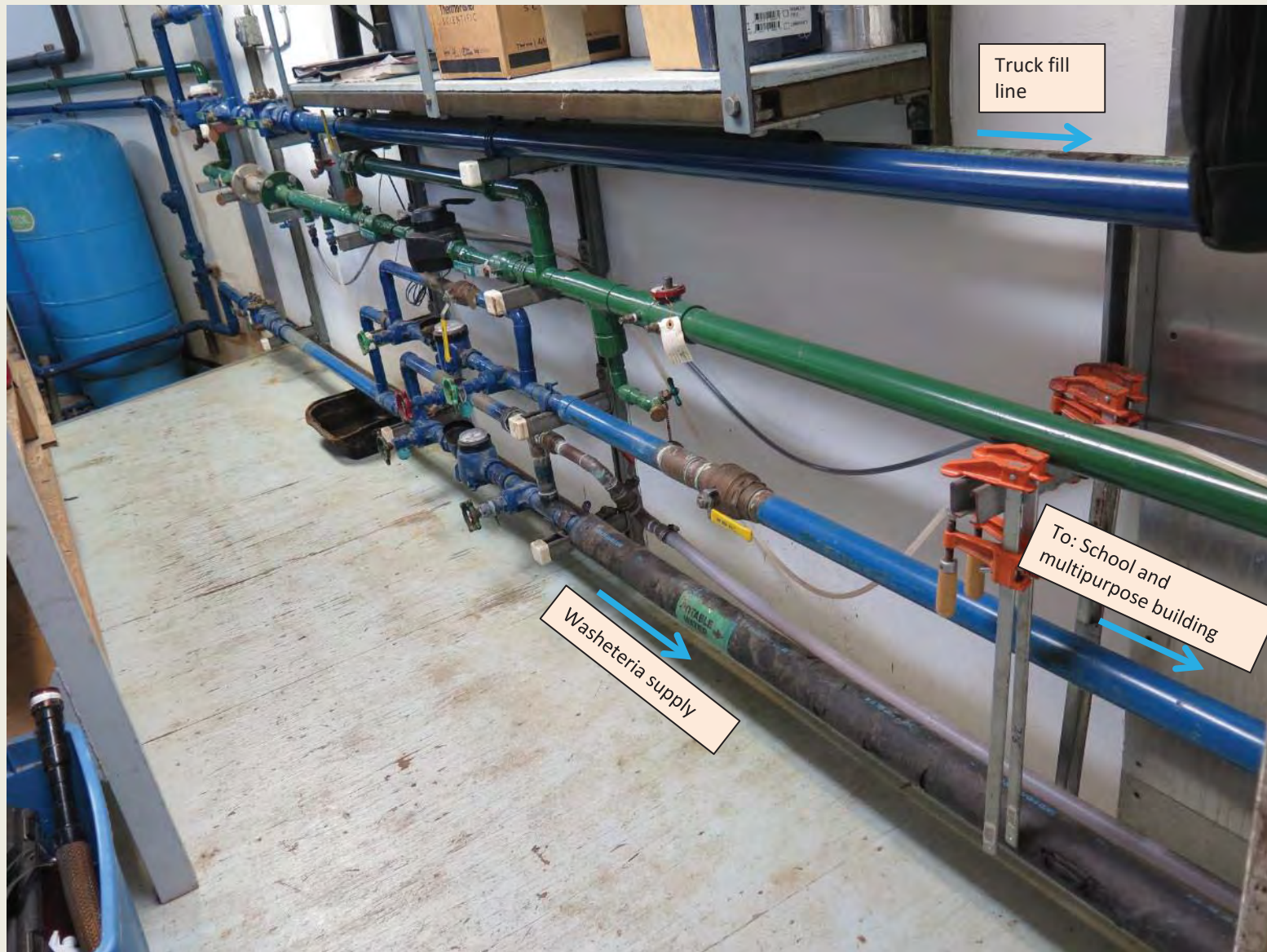
Photo 38: distribution system piping, with separate metering of individual service lines
