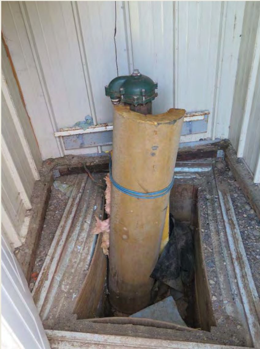
Photo 2: Well WL001, showing pit left when gravel fill was removed to install glycol heat trace piping
