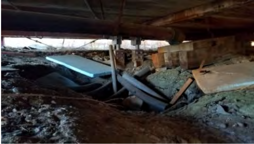
Figure 19: Depression Under Washeteria
