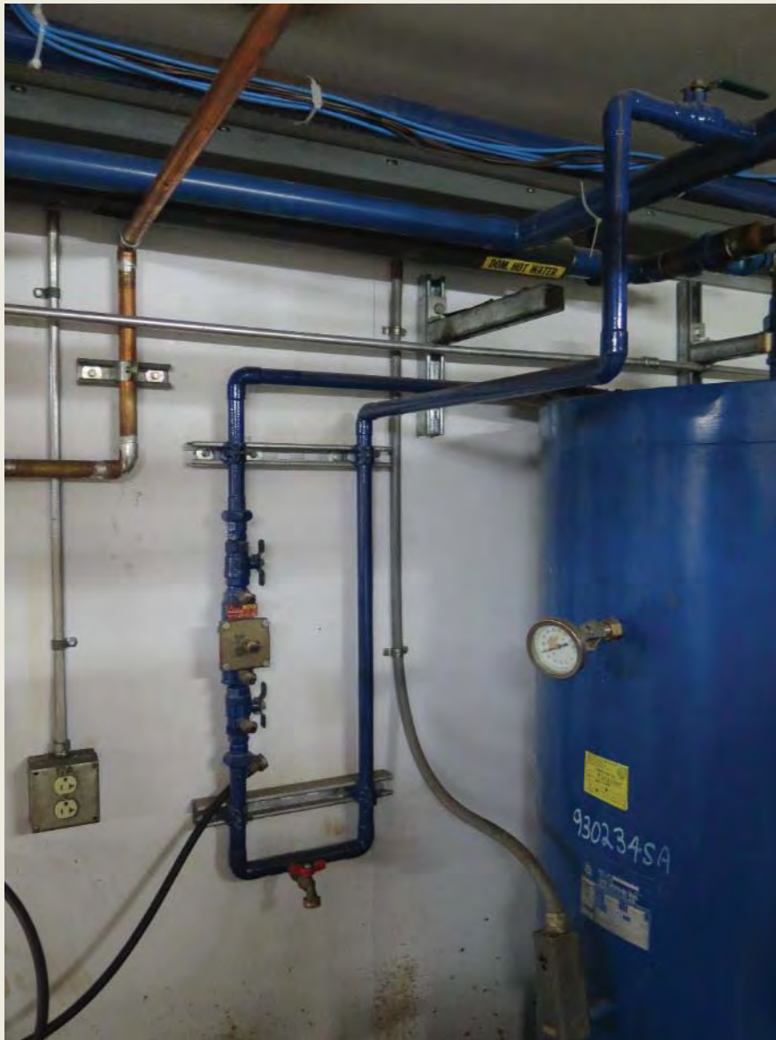
Photo 40: Backflow preventer on potable water supply to hot water generator.
