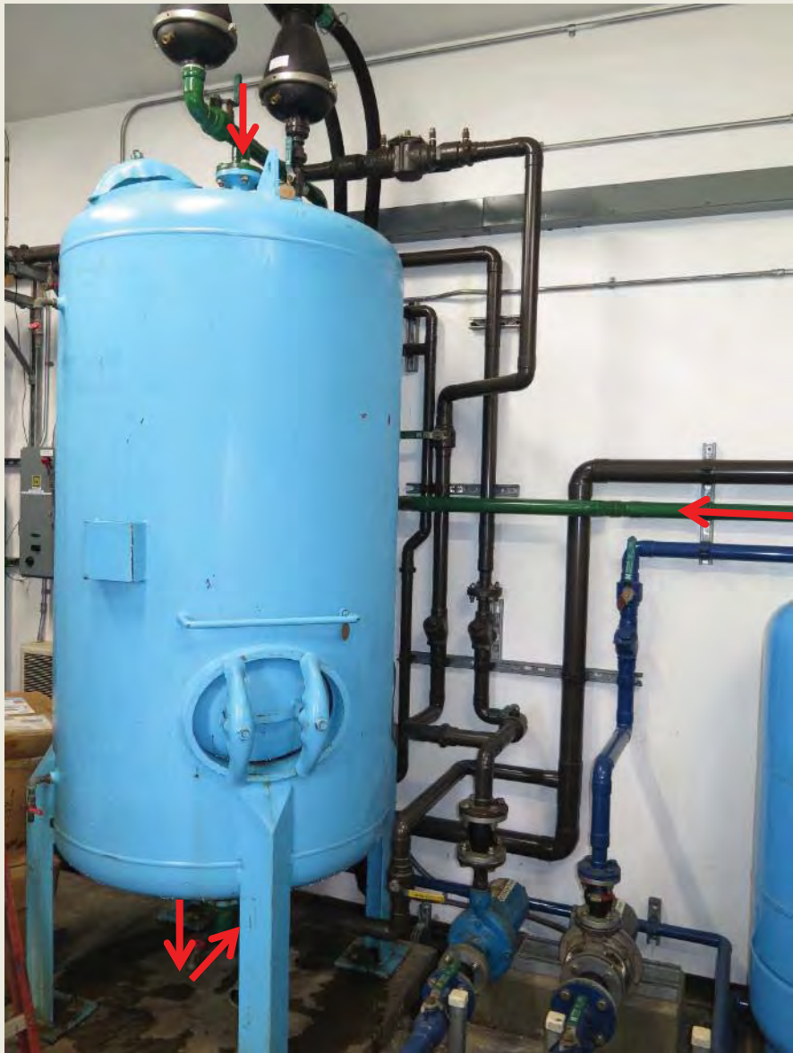
Photo 14: Raw water detention tank, intended to provide contact/reaction time for oxidation of iron and manganese.
