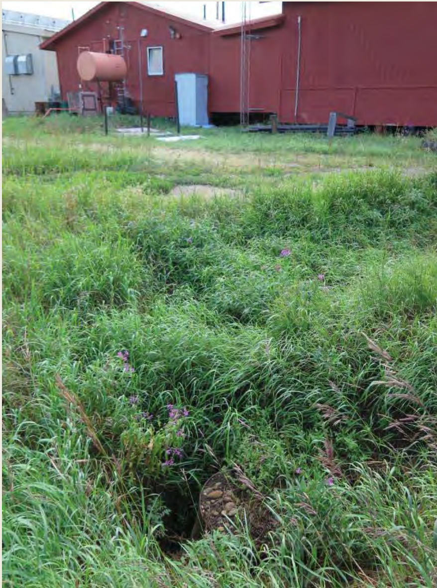
Photo 59: Another shot of the sinkhole(s) behind the washeteria, showing gravel-filled drum placed into center.
