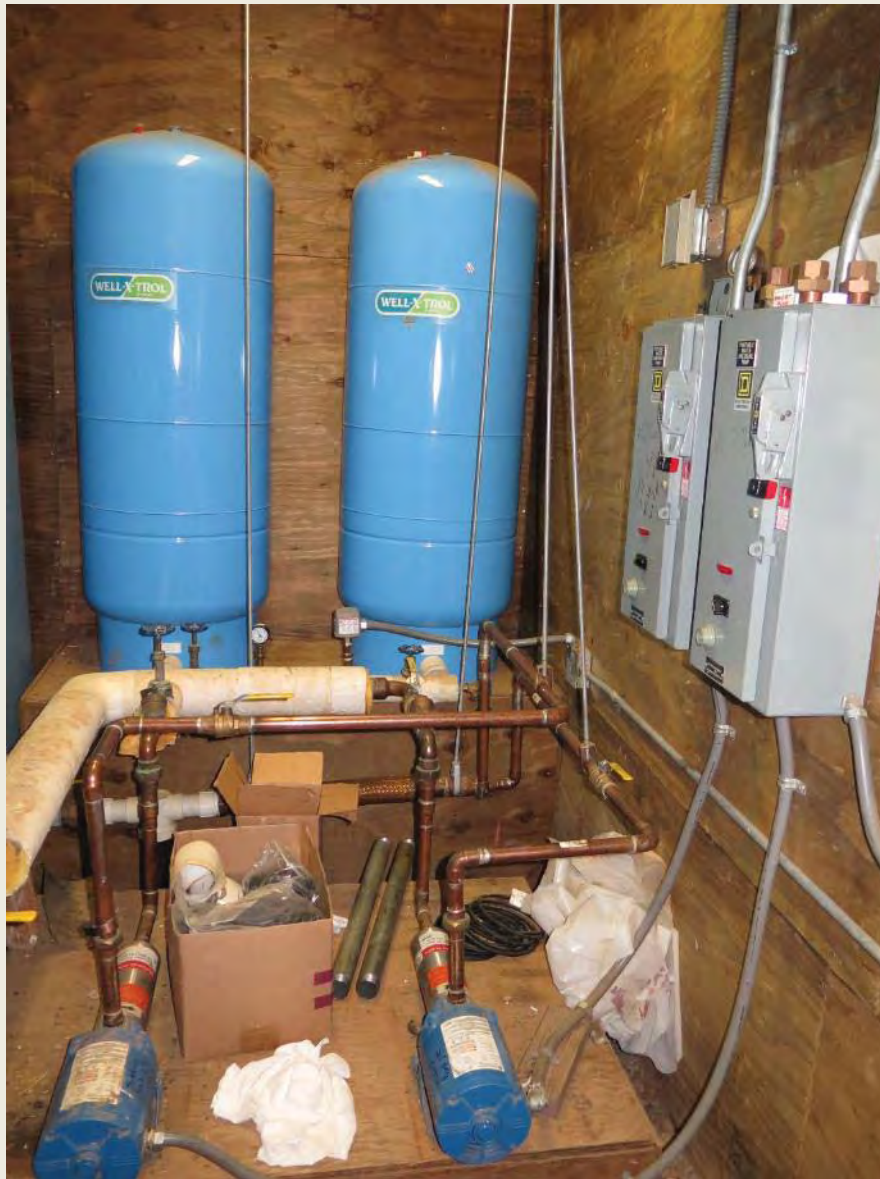
Photo 51: School's pressure pumps and pressure tanks, piped from indoor storage tank to school. This system is valved "off" but still hard-piped to the water distribution system.
