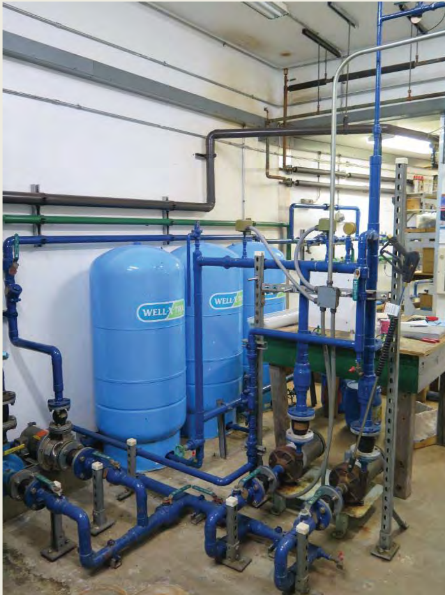
Photo 34: Distribution system pressure pumps & pressure tanks
