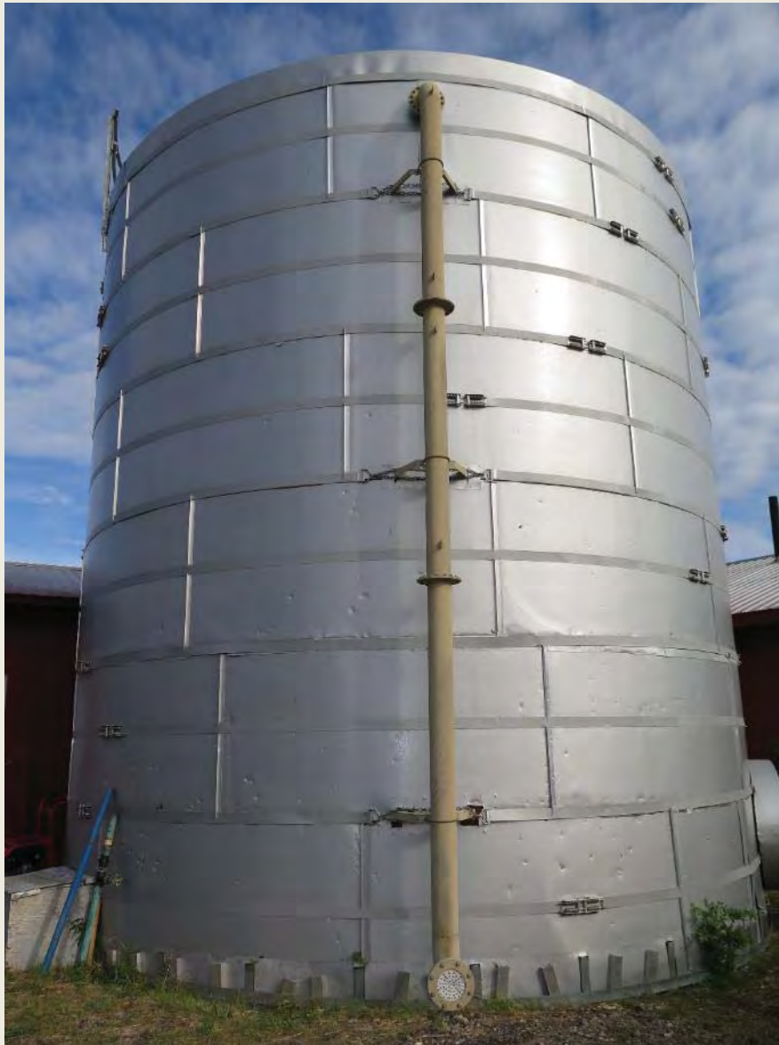
Photo 25: Water storage tank, showing overflow pipe with perforated screen.
