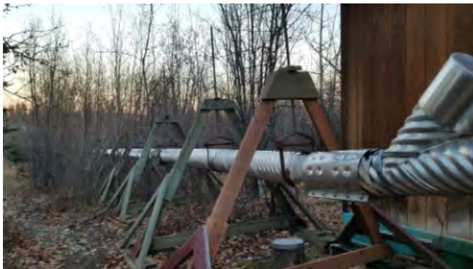
Figure 10: Outfall from Lift Station to Lagoon
