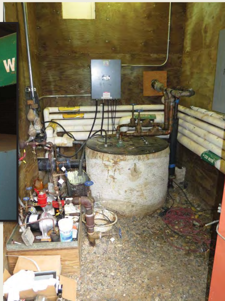
Photo 54: The school lift station, located in room adjacent to school water tank and pressure distribution pump system. The sewer main is located in the same utilidor as the water lines.
