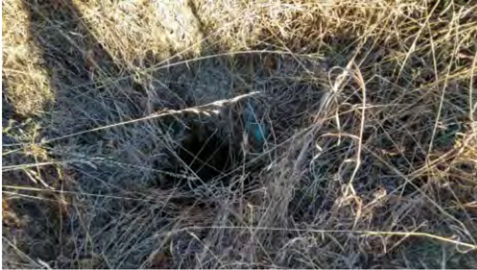
Figure 16: Depression, East Hole, Insulation Board Exposed
