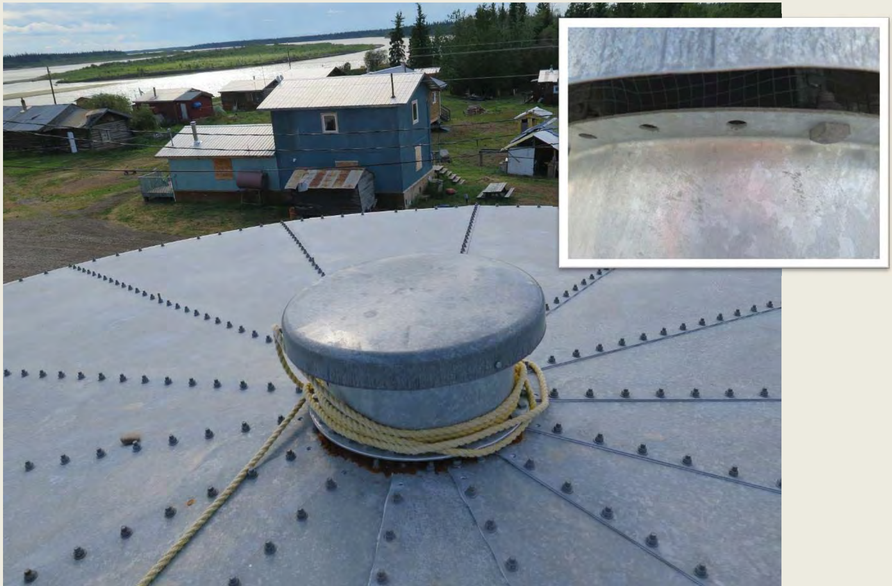
Photo 28: Tank vent & screened opening
