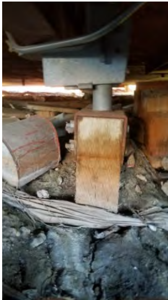
Figure 21: Washeteria Foundation Pile Failing
