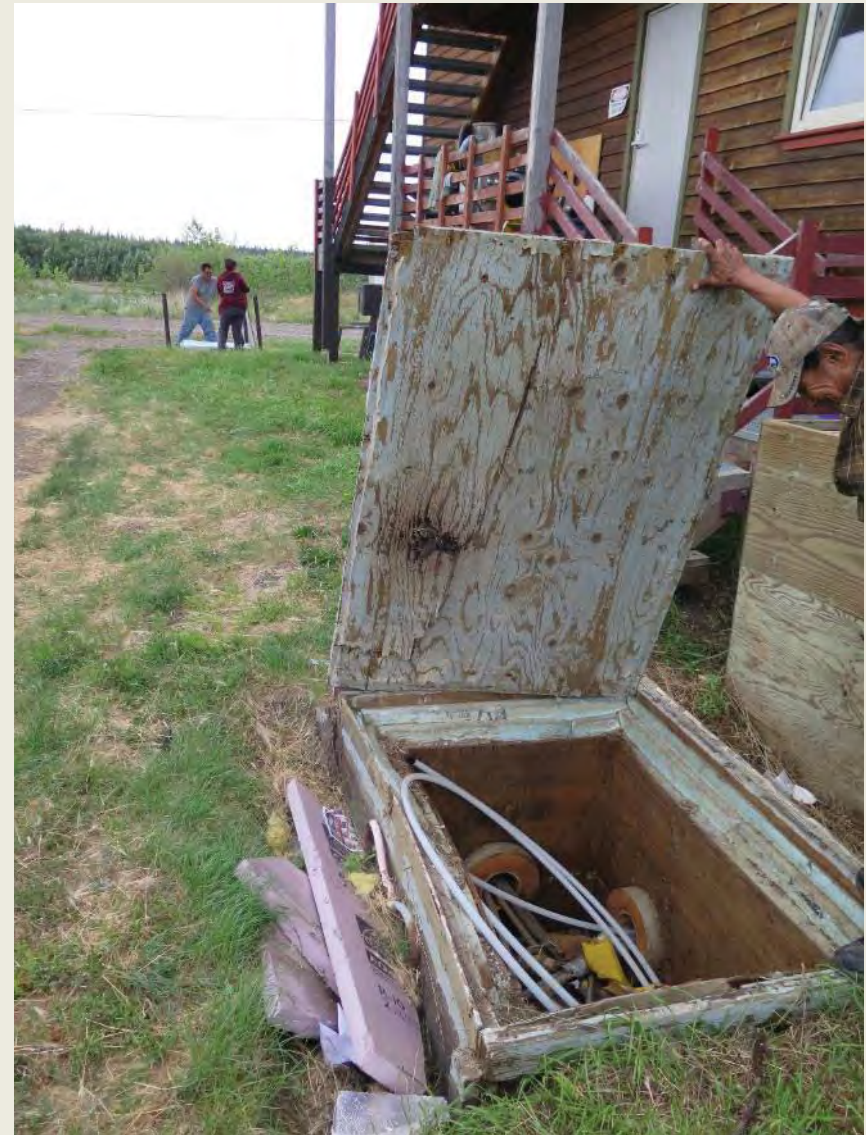
Photo 9: Second manhole on raw water transmission line, where it joins treated water and sewer utilidor behind multi-purpose building (first manhole in background). New PEX tubing (white) for in-progress service line project visible.
