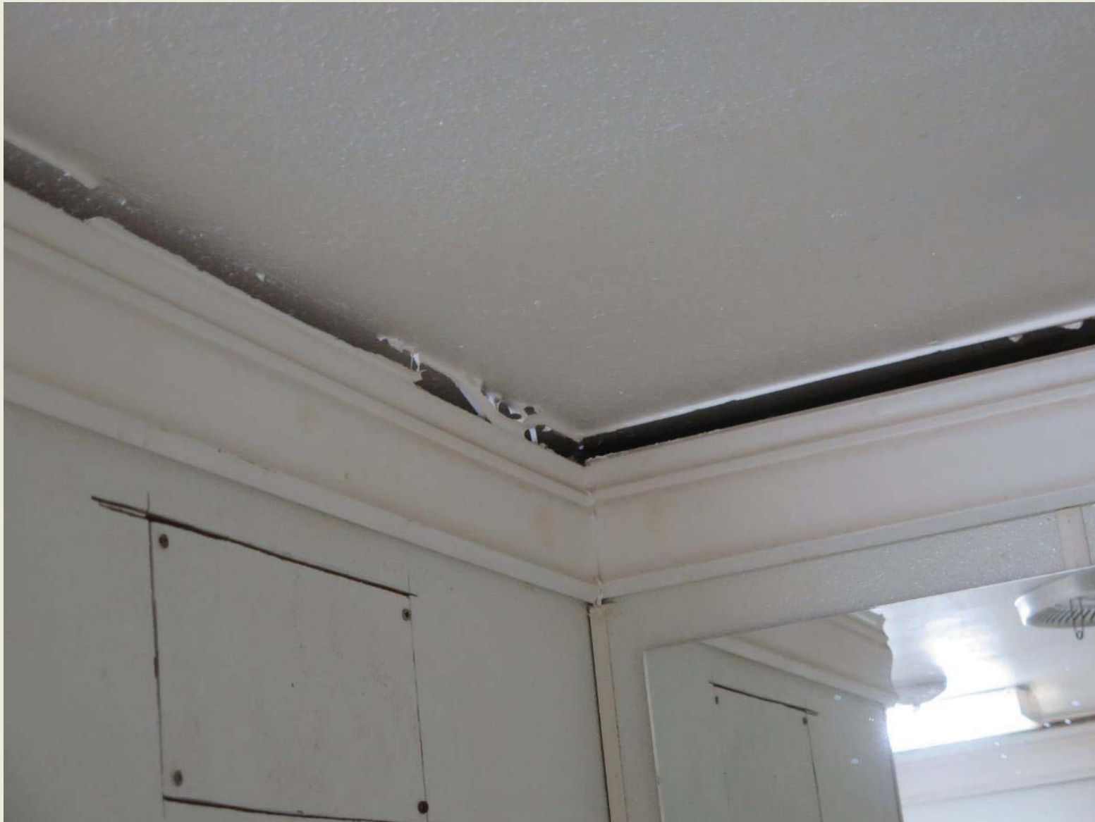
Photo 57: Evidence of the building suffering differential settlement: the ceiling in the washeteria area has separated from the walls by more than one inch. This extends into the office/chemical storage room, but was not observed in the water plant area.
