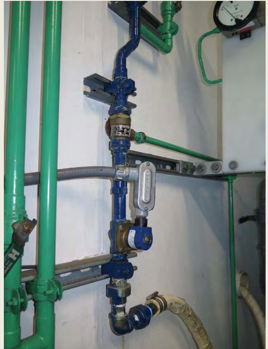
Photo 37: Watering point interior plumbing showing Watts 9D-M2 dual check valve with intermediate atmospheric vent (drains to green pipe). This model check valve is not rated for potable water use, and not certified lead-free.
