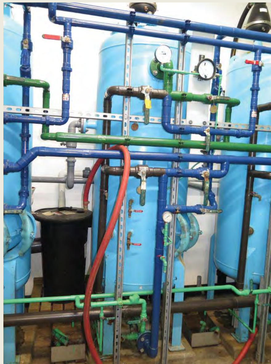
Photo 18: Filter vessel piping and sump tank, used to collect and pump freeboard drain effluent to backwash tank.
