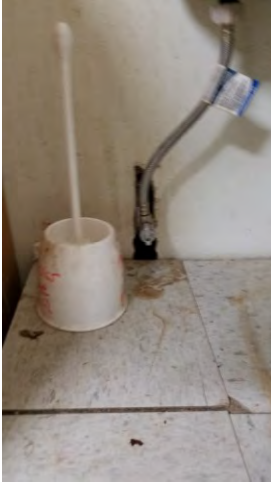
Figure 36: Bathroom-Toilet Repair Due to Settling
