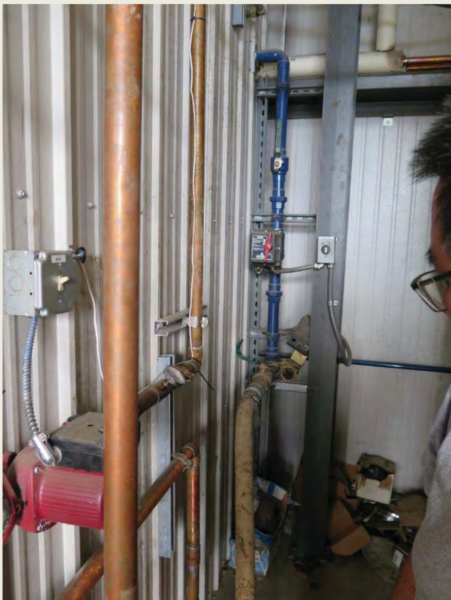
Photo 42: Truck fill piping (blue) and hose, in haul truck garage.
