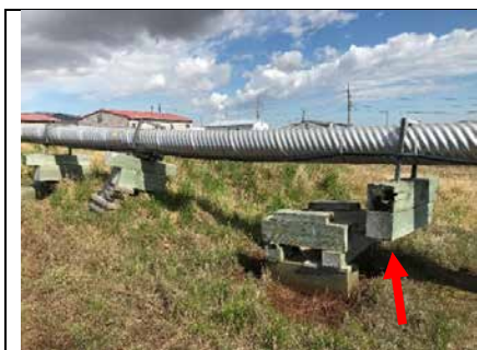
Photo 11 Failed Waterline Supports Support has failed and is pulling waterline down. (Stantec 6/2018)
