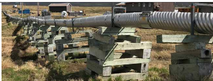
Photo 12 Waterline Sagging on Failing Supports Supports are unstable and falling over, line has visible sagging. (Stantec 6/2018)
