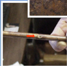
Fuel line corrosion caused by electrolysis
