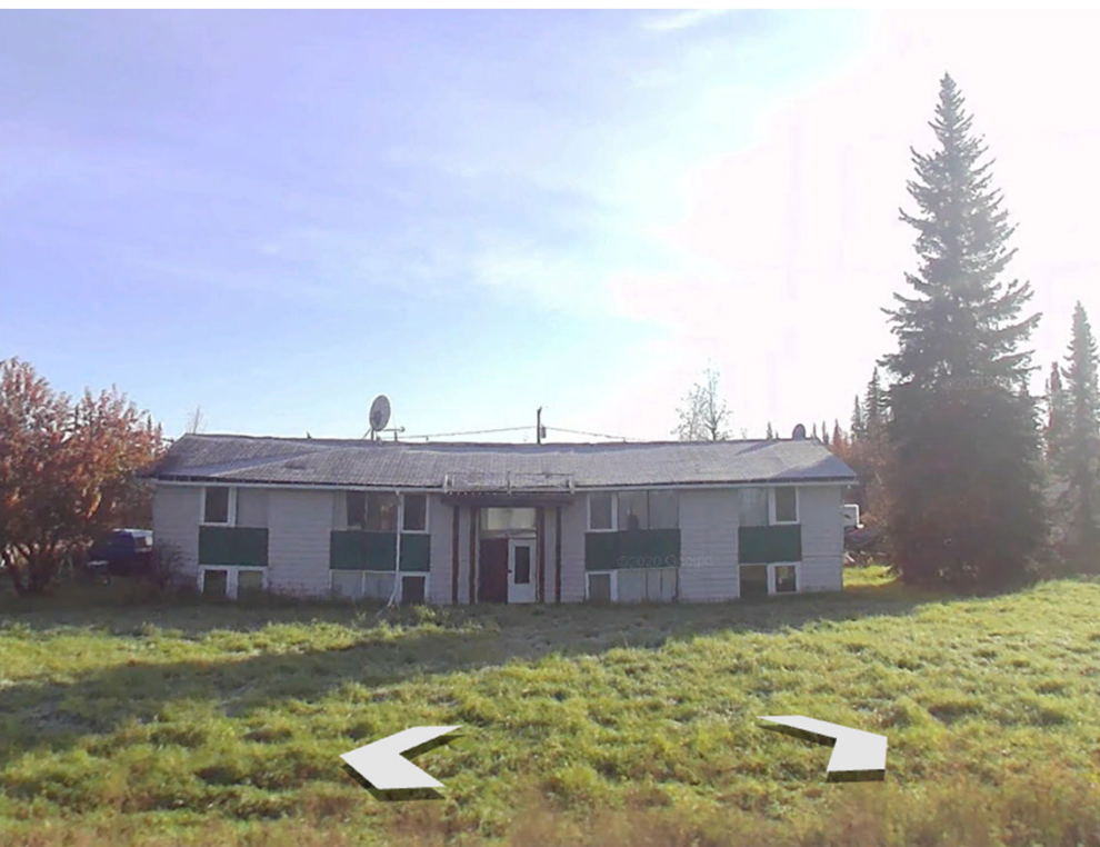
West side of the house near Farmer's Loop Road
