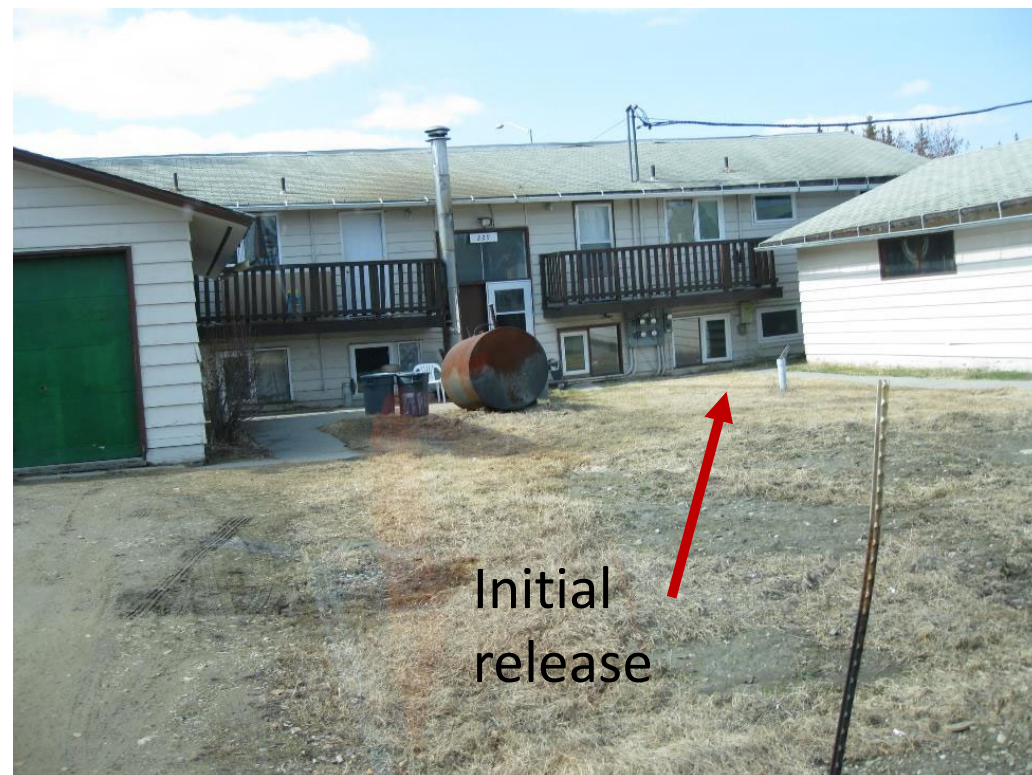
East side of the house near Madcap Lane
