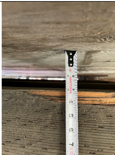
22 - Temp. Support under vessels – 3 inches low
