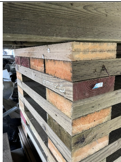
23, Dunnage Support for temporary support under vessel
