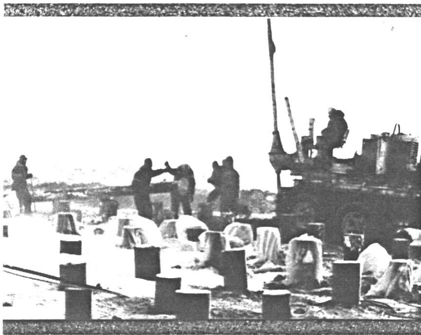
KEEPING SNOW OUT OF THE BORE HOLES
