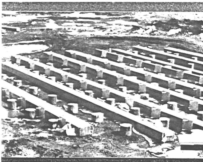
GLUE-LAM BEAMS WILL SPAN THE PILES
