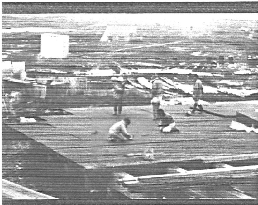
INSTALLING CUSHION FOR TANK
