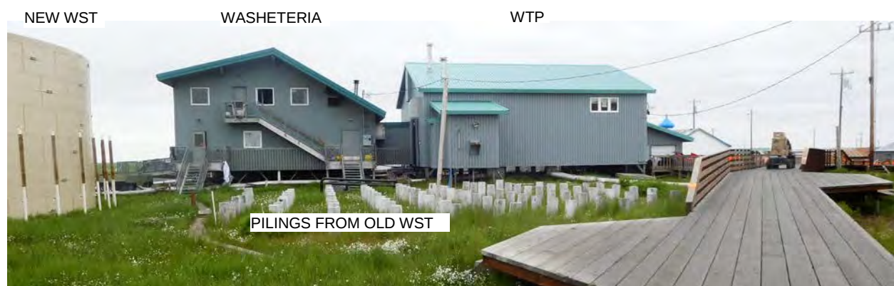
Exhibit 2-1: Kongiganak WST, WTP/Washeteria, and old WST pilings (2019).
