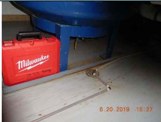
Photo 20 – Vertical Supports for Vessels on 2 nd floor. Channel is under legs on middle vessel only.
