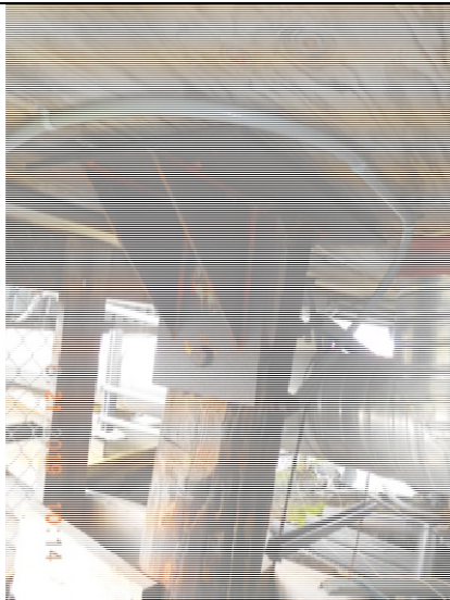
Photo 2 – Typical WTP Piling Bracket
