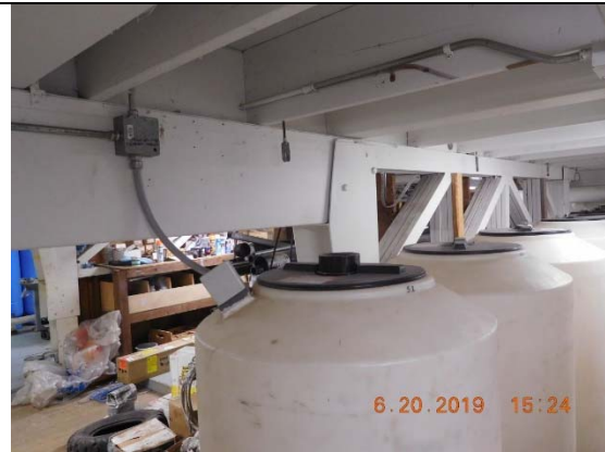
Photo 30 – Typical header connection to column at walkways.
