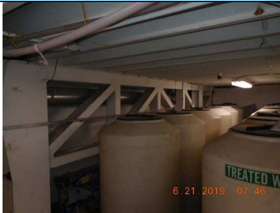
Photo 16 – 165 Gallon Tank Loading, WTP First Floor
