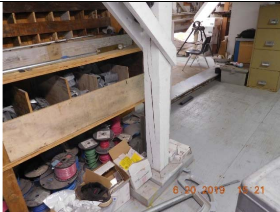
Photo 29 – Frame Column showing cracks
