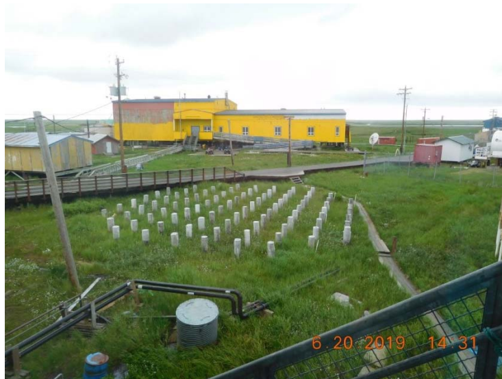
Photo of wooden piling for previous water storage tank.
