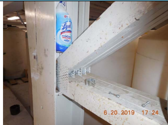
Photo 13 – Typical truss connection at column
