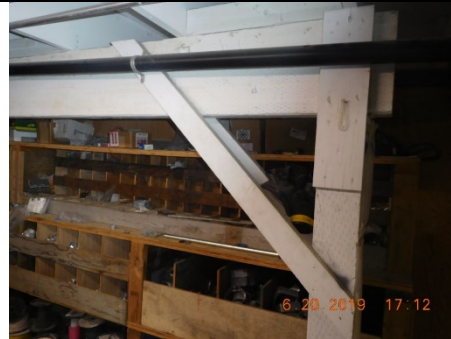
Photo 7 – Existing frame bent showing top connection and diagonal supports
