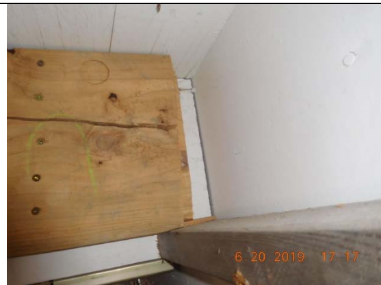
Photo 26, Sistered joists in vicinity of vessels above. Note lack of bearing distance.
