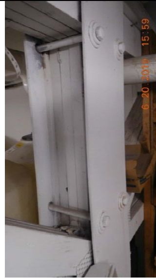
Photo 9 – Typical wall truss support for second floor at column.
