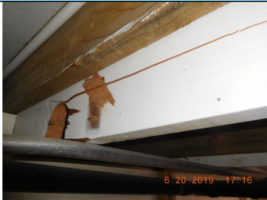
Photo 12 – Second floor joists above support bent. Note longitudinal crack at top of utility cutout. Also, not sister joist.
