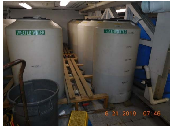
Photo 15 – Typical Tank Loading in Bay 1 (West side only, Bay 4 both sides).
