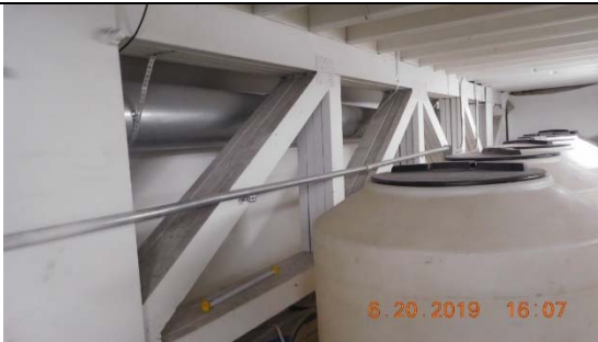
Photo 10 – Typical Wall Truss at each bay. Trusses run east-west. Also note floor joists for second floor.
