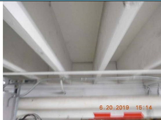
Photo 28 – Typical 2" x 12" Framing. Bay 1, 3, 4. Not Bay 2.
