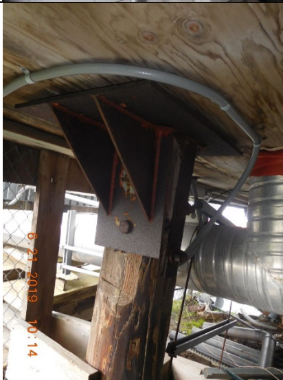
Photo 2 – Typical pile support bracket and pile under WTP
