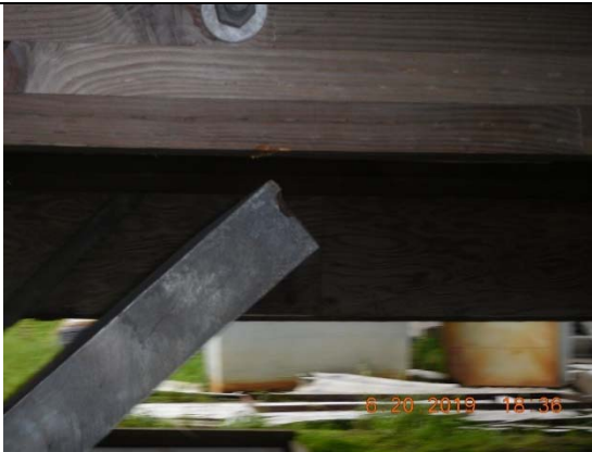
Photo 45 - Under Washeteria. Note broken angle
