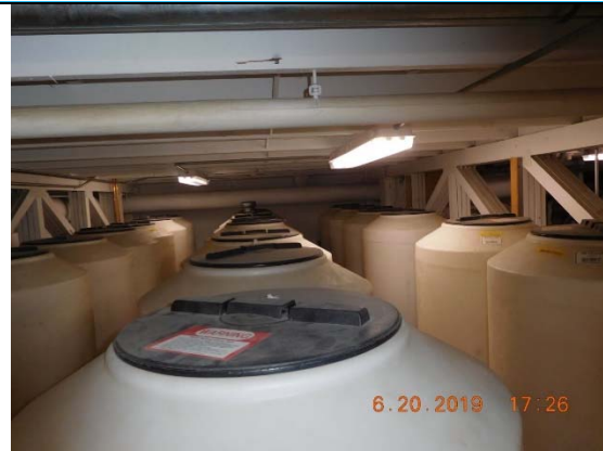
Photo 17 – Typical 165 Gallon Tank Layout
