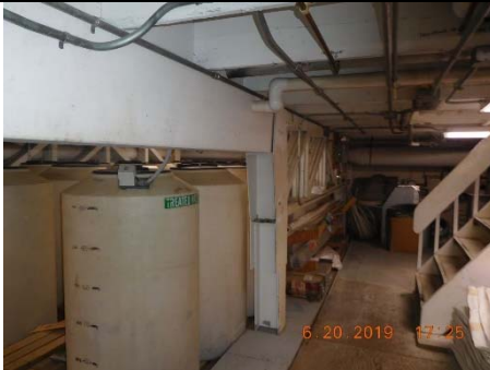
Photo 6 – Header at walkway, first floor WTP. Also showing staircase to second floor
