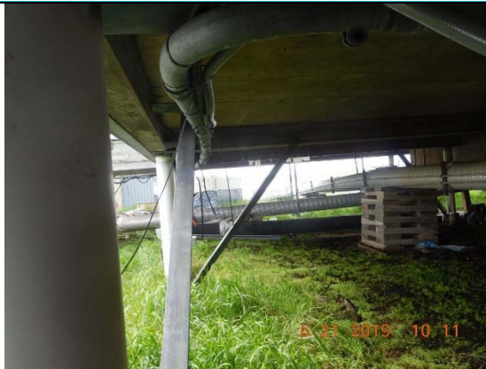
Photo 43 – Under Washeteria. Note bent angles
