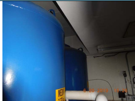
Photo 32- Raised Ceiling at Vessels on Second Floor. Head Room = 10'-1", Typical Second Floor Head Room = 7'-11"
