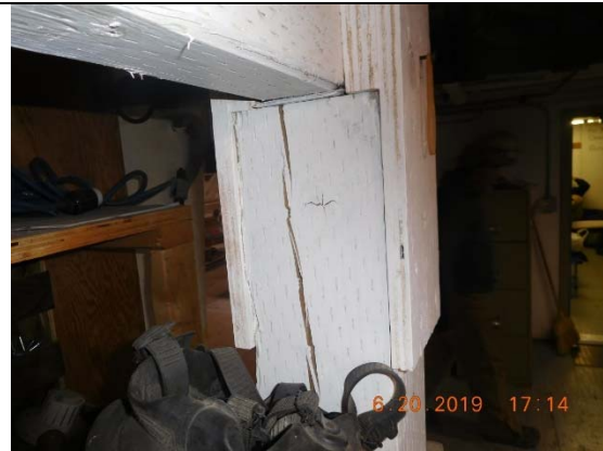
Photo 23 – Cracks in east column on frame for vessel supports.
