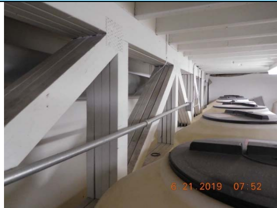
Photo 48 - Multiple ply trusses at each wall section on first floor.
