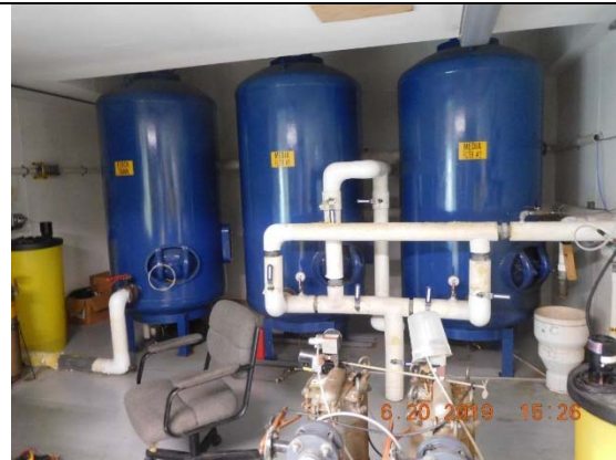
Photo 19 – Three Filter Vessels on Second Floor.
