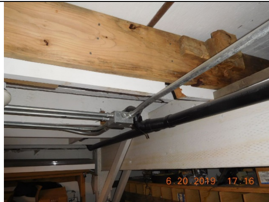
Photo 11 – Joist framing above support frame for second floor. Note sistering of existing joists.
