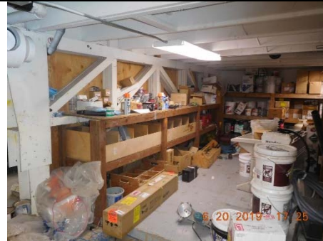
Photo 7 - First Floor WTP, Bay 3. Showing typical truss layout for support of second floor joists.
