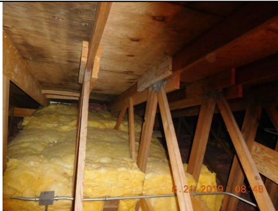
Photo 35 - Roof Trusses over raised ceiling area. Note Blocking and craming.
