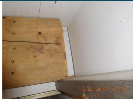
Photo 13 – Sister joists on south end from photo 12. Not minimal bearing distance and longitudinal crack.
