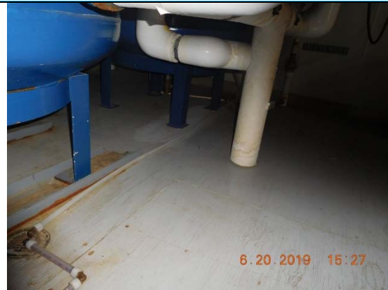
Photo 21 – Vertical Supports for Vessels on 2 nd floor. Channel is under legs on middle vessel only.
