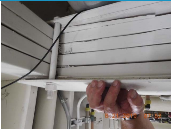
Photo 47 – Multiple ply trusses at each wall section on first floor.
