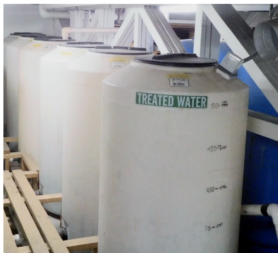
Exhibit 3-3: Current Treated Water Storage
