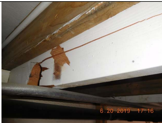
Photo 25 – longitudinal crack on second floor, floor joists – directly under vessels.
