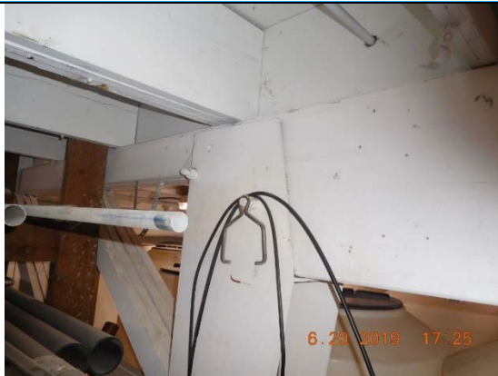
Photo 12 – Typical header beam and truss connecting to column.
