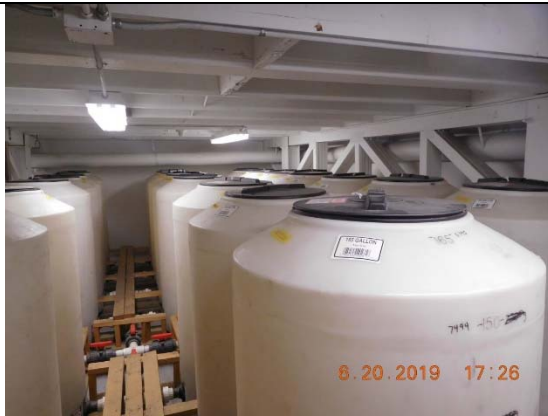
Photo 18 – Typical 165 Gallon Tank Layout, First Floor WTP
