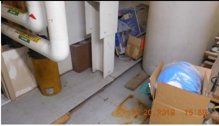
Photo 8 – Support Column, First Floor. Columns extend vertically at each pile to second floor
