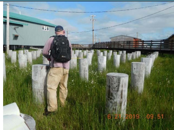
Photo 40 – Previous Water Storage Tank, 88 piles.
