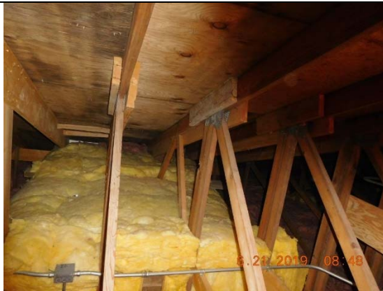
Photo 33 – Roof Trusses over raised ceiling area. Note trusses – 2x6 top and bottom chords. Tursses Spliced – 3 piece trusses.
