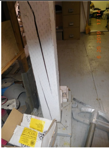
Photo 8 – Support Column, east side of support bent on first floor. Note cracking
