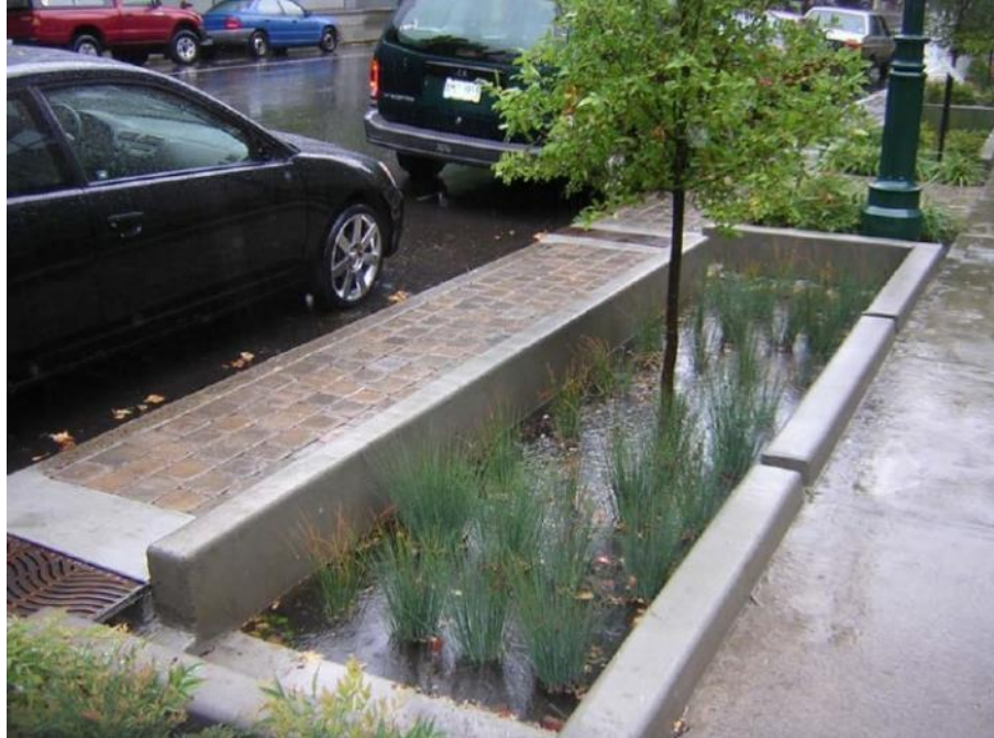
Figure 17. A bioretention planter in Portland, Oregon. Trench drains serve as inlets and outlets for street runoff; curb notches are inlets for sidewalk runoff. (Washington Stormwater Center Training Manual)
