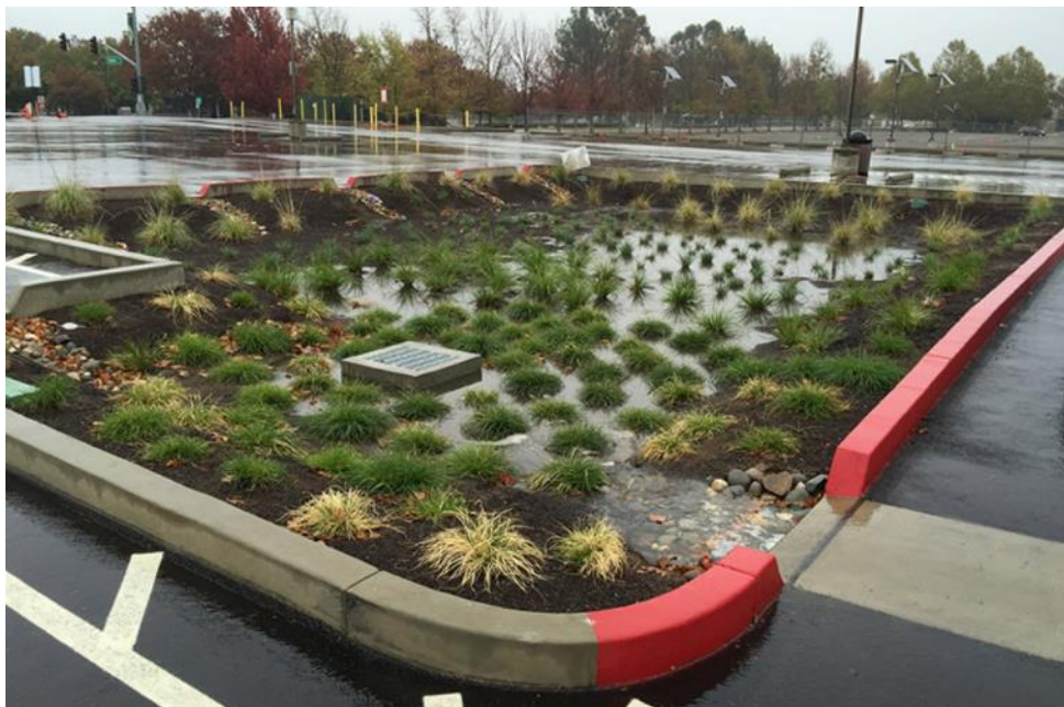
Figure 281. Bioretention planters in parking lots can treat and infiltrate runoff from large contributing areas and provide attractive landscaping for retail properties. An overflow drain (center left) can convey excess runoff to grey stormwater infrastructure or to another stormwater BMP. (credit: https://www.owp.csus.edu/lid/site/lot-7-bioretention-planter.html )
