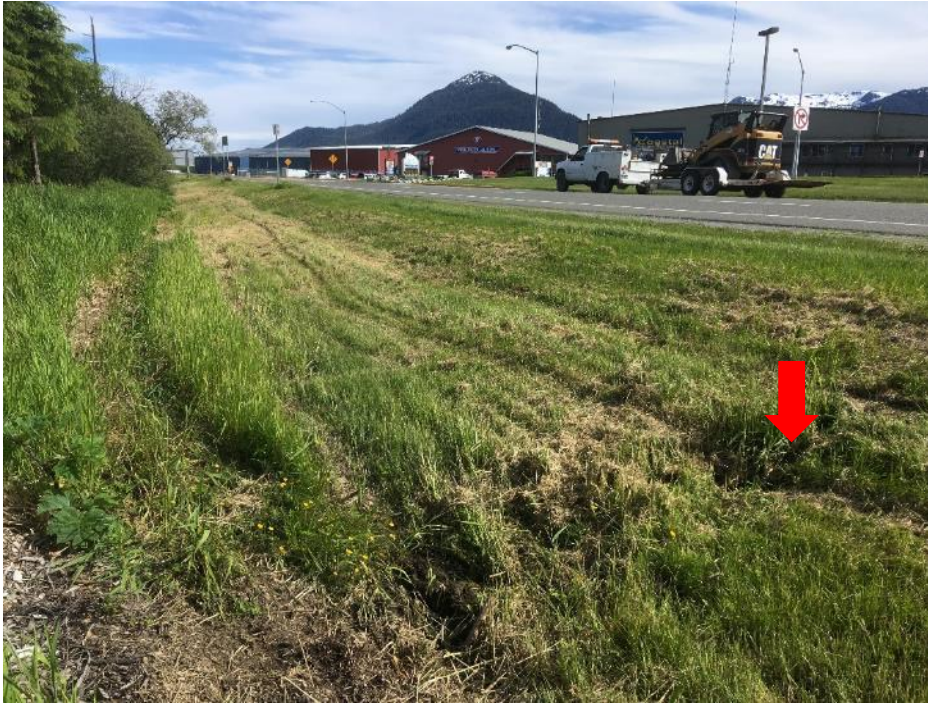
Figure 52. The Yandukin Drive Middle stormwater system discharges runoff from a pipe (indicated by red arrow) into a grass swale next to Jordan Creek (left of photo). View looking southeast from the north side of Yandukin Drive in June 2020.
