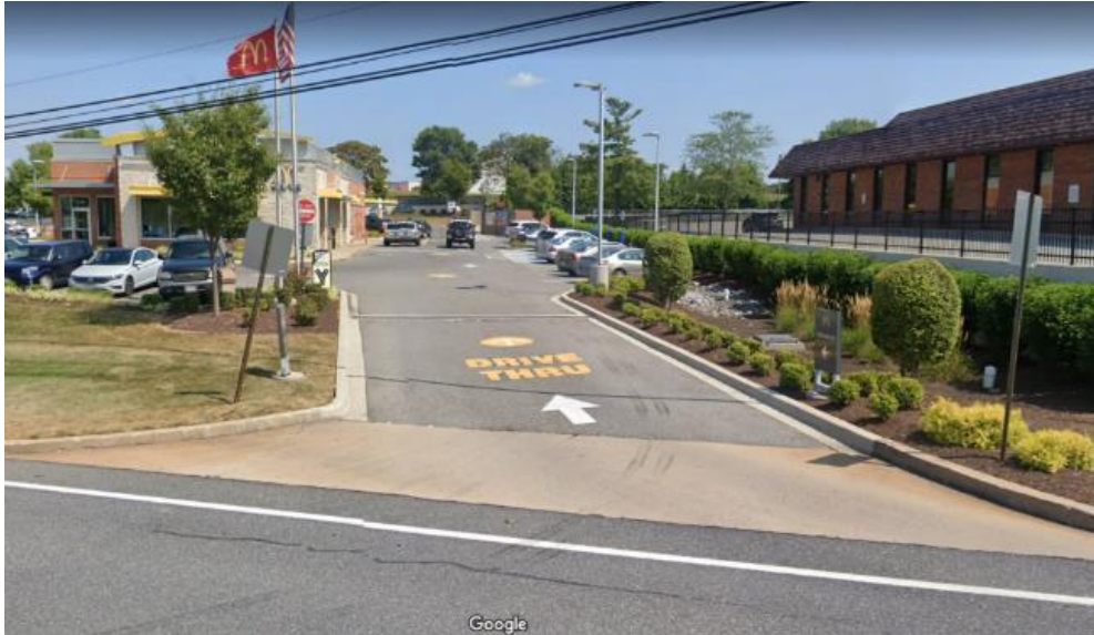
Figure 11. Stormwater runoff from a McDonald's restaurant in Westminster, MD is collected in a trench drain (center) at the drive-through entrance and conveyed to a landscaped infiltration BMP (right). Note the square-shaped raised overflow drain. Google Street View.
