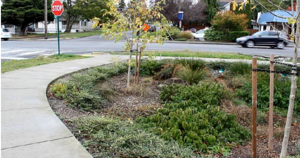
Figure 14. Bioretention cell. Note the overflow drain with beehive grate (center) and the two blue inlet pipes (center right) that convey runoff from the street into the cell (Washington Stormwater Center Training Manual).
