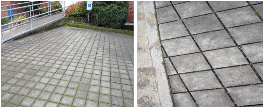
Figure 4. Left: a parking lot paved with PICP. Right: PICP closeup (Washington Stormwater Center LID Training Manual).
