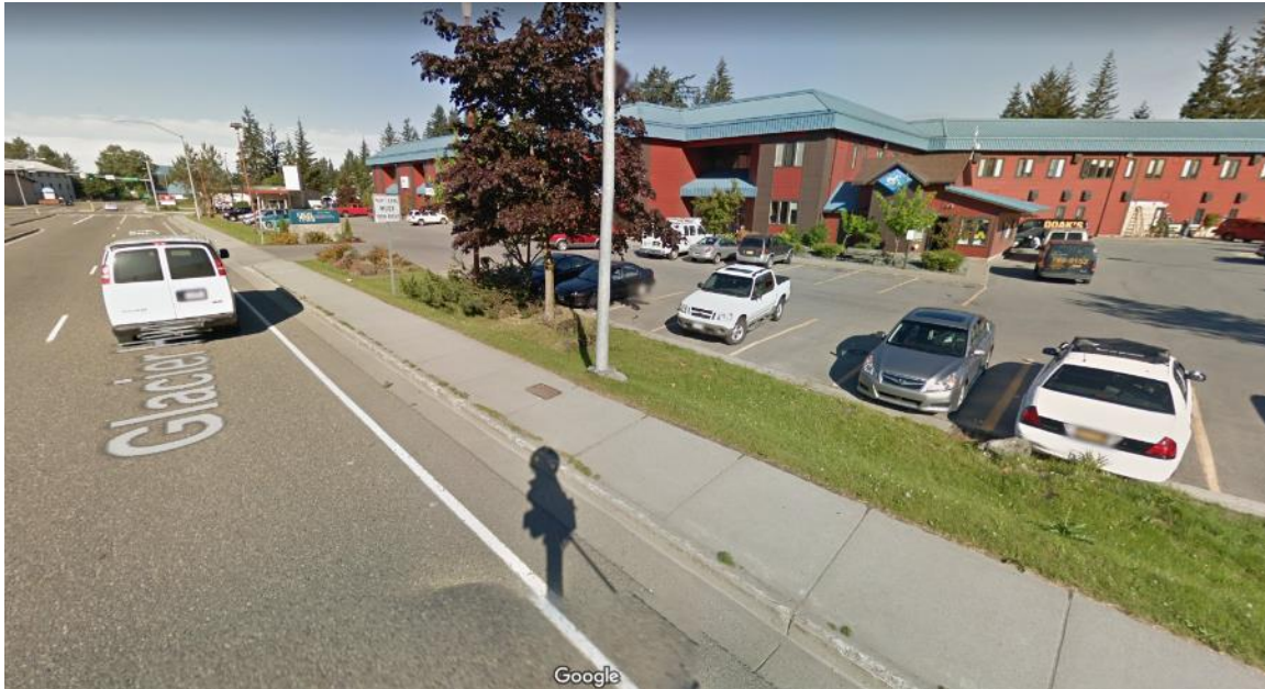
Figure 19. Two grass swales border an entrance drive connecting Jordan Creek Center to Glacier Hwy. Converting the swales into bioretention BMPs would provide treatment and infiltration of runoff from Glacier Highway and the parking area. Google Street View looking southwest in July 2011.
