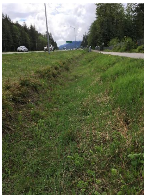
Figure 5. Left: An existing infiltration basin near the downstream end of stormwater system 1. View looking towards inlet pipe (upper right) in May 2020. Right: Runoff from stormwater system 1 flows through a pipe into this ditch on the west side of Egan Drive. The ditch connects to Jordan Creek in the distance. View looking southeast from the pipe outlet. May 2020.
