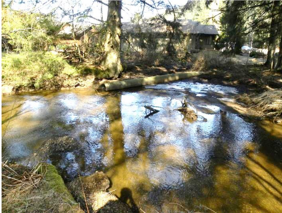
Figure 14. Stormwater outfall 5. Stream flow is from right to left. View looking north in March 2020.
