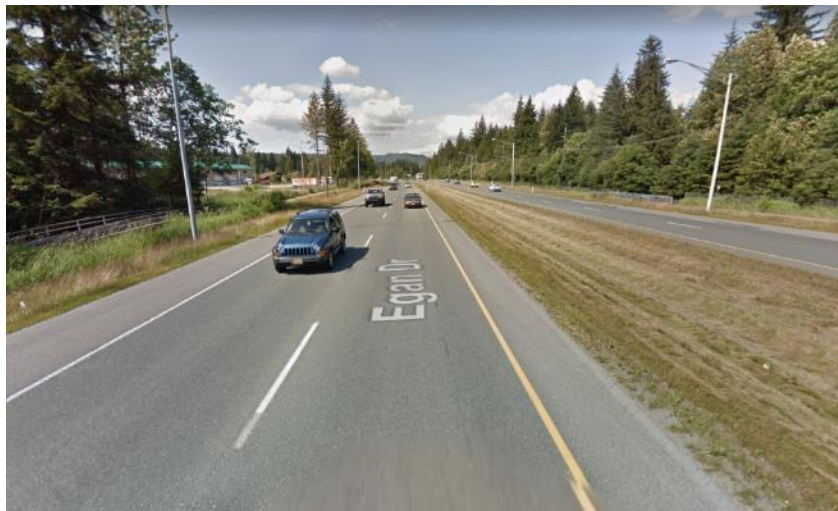
Figure 24. The median and outer margins of Egan Drive function as vegetative filter strips. View looking northwest where the highway crosses Jordan Creek (Google Earth Street View).
