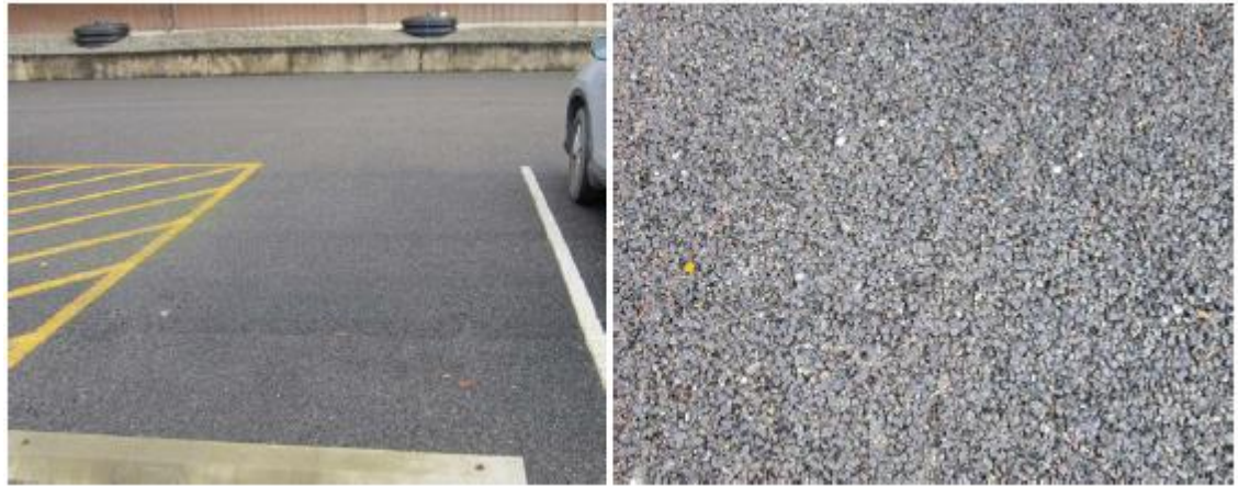
Figure 2. Left: A parking lot paved with porous asphalt. Right: porous asphalt closeup (Washington Stormwater Center LID Training Manual)
