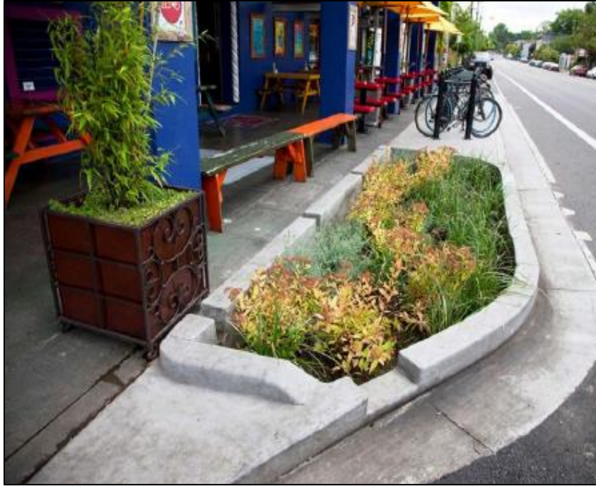
Figure 19. A bioretention planter in a curb extension designed to receive runoff from the sidewalk and street in Portland, Oregon. Curb extensions provide space for stormwater BMPs where right-of-way space is limited and improve auto, pedestrian, and bicycle safety by shortening the crossing distance for pedestrians, improving sight lines, and providing a visual presence in the roadway to slow vehicles approaching intersections (Washington Stormwater Center Training Manual).
