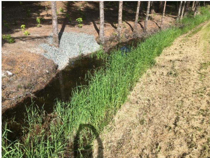
Figure 9. The inlet end of a 150-foot long infiltration trench that receives runoff from the west end of Yandukin Drive near Jordan Creek.
