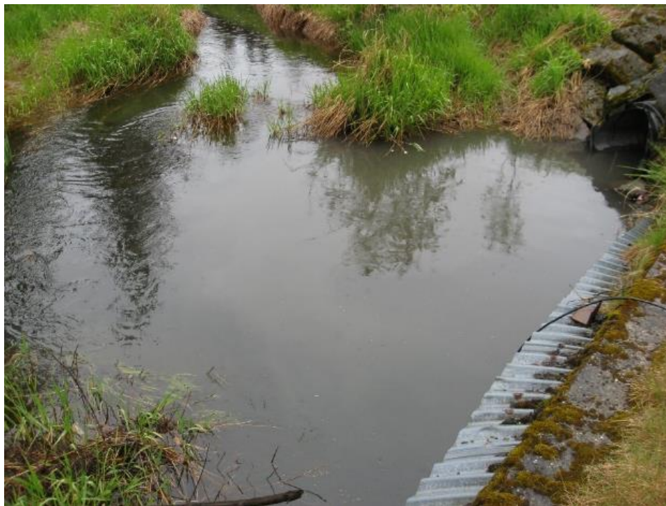
Figure 17. Stormwater runoff containing suspended sediment flows into Jordan Creek from the stormwater system 6 outfall pipe (upper right) and mixes with clear water in Jordan Creek upstream of Glacier Highway in May 2020.
