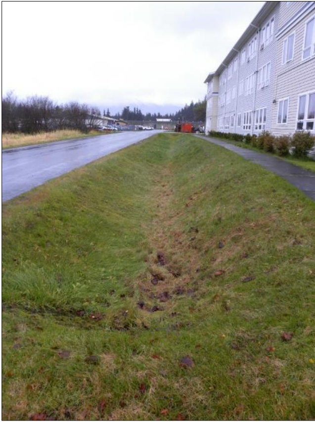
Figure 56. A grass-lined swale on the east side of Alpine Ave. South. View looking north towards Teal Street in October 2014.
