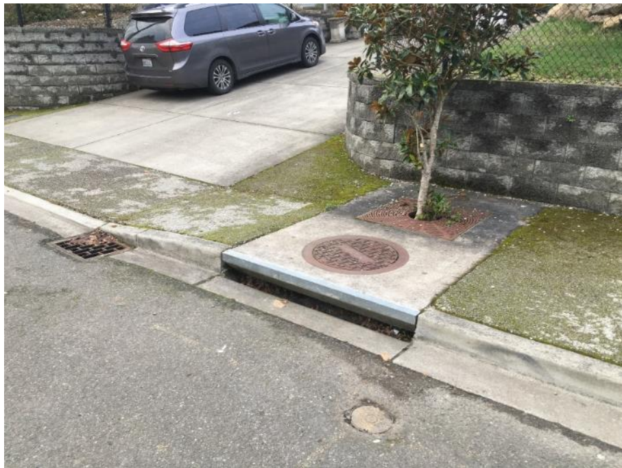
Figure 18. This bioretention planter containing a single tree intercepts runoff from curb and gutter immediately upstream of a catch basin (center left) in Seatac, WA. Note the sidewalk is constructed with pervious concrete.
