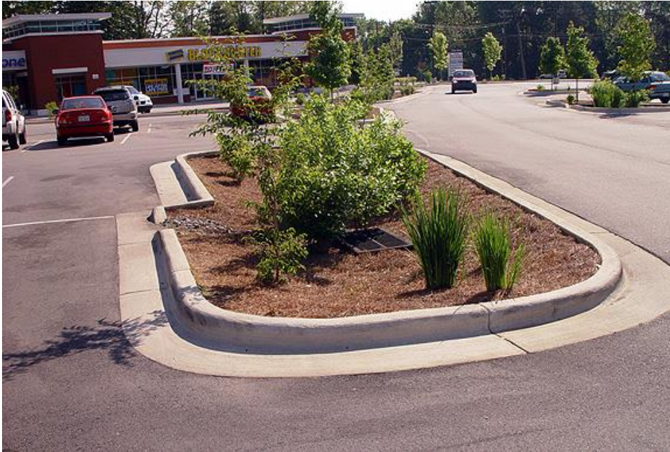
Figure 35. A bioretention planter between a parking area and an access drive (credit: https://www.hazenandsawyer.com/publications/urban-green-infrastructure-solutions/ )
