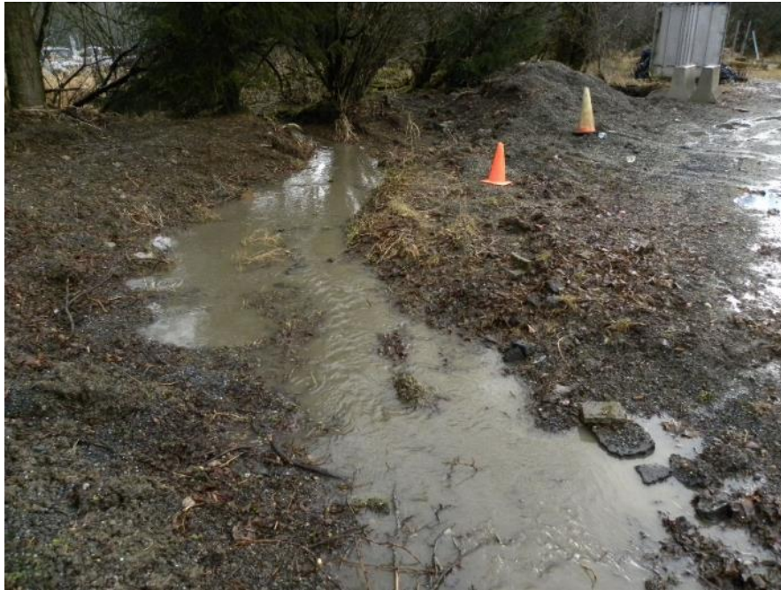
Figure 48. Stormwater runoff from gravel and paved parking areas near the Edward K. Thomas building flows towards Jordan Creek prior to construction of the infiltration trench. View looking southeast in February 2016.
