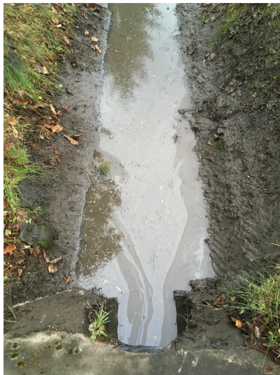
Trout Street Ditch in the Lower Jordan Creek watershed.
