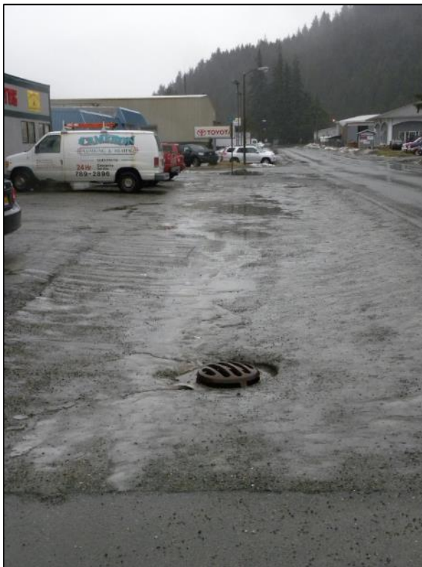
Figure 30. A stormwater catch basin in a gravel-surfaced area in the Crest Street right-of-way. View looking north towards Teal Street in January 2013.
