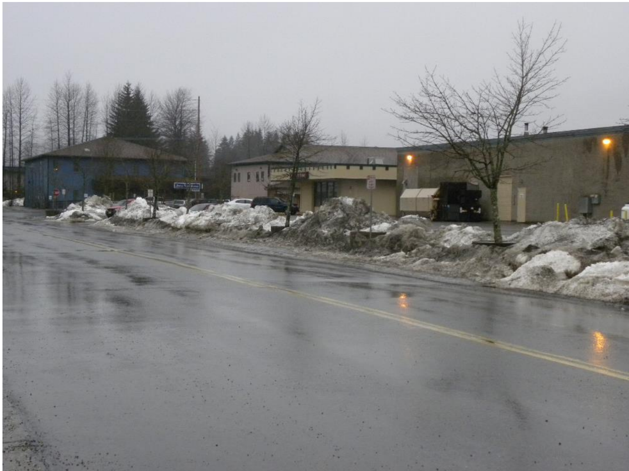
Stormwater from the west end of Mallard Street drains to stormwater system 9 in the Lower Jordan Creek watershed.
