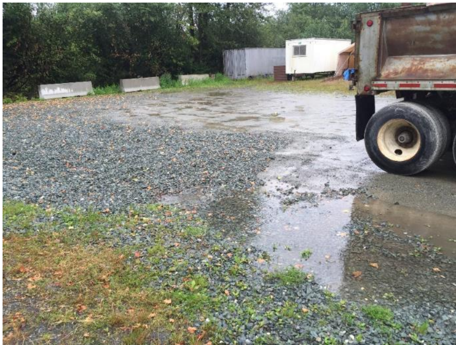
Figure 49. Stormwater runoff enters an infiltration trench (photo center) on the south side of the Edward K. Thomas building. The vegetated portion of the trench is behind the concrete barriers. View looking southeast in August 2016.
