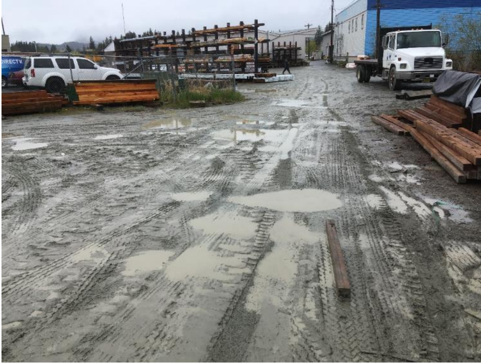
Figure 36. The Valley Lumber lumberyard produce large quantities of sediment-laden stormwater, some of which enters stormwater system 10. May 2019.
