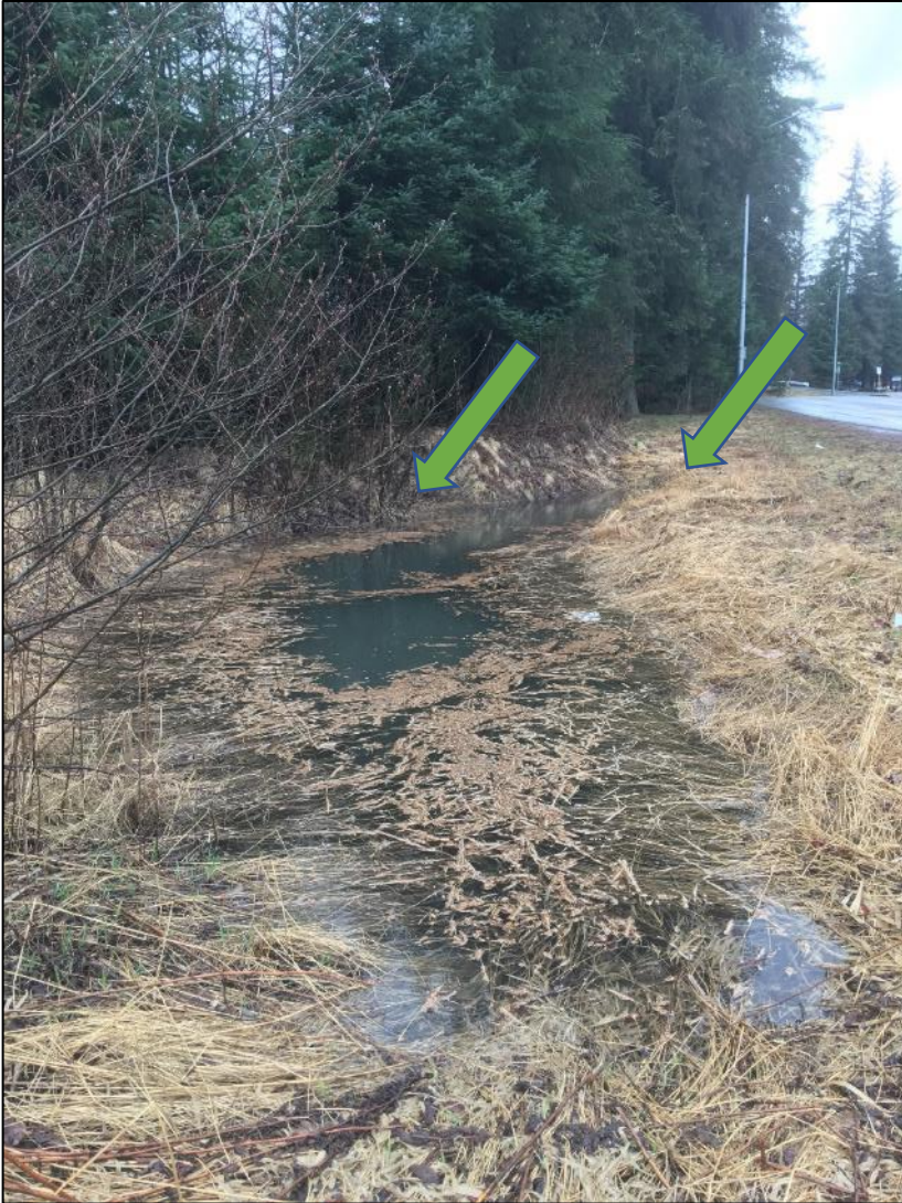
Figure 7. An infiltration basin at the downstream end of stormwater system 2 in April 2020. Arrows indicate the inlet pipe (right) and outlet trench (left). View from north end of basin looking south in April 2020.
