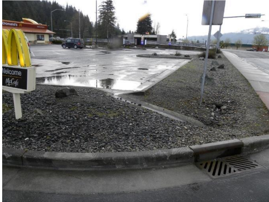
Figure 9. Stormwater runoff from the west side of the McDonald's parcel enters stormwater system 3 at the entrance driveway. Runoff from the driveway and Trout Street flows into the catch basin. View looking southeast along Trout Street in May 2010.
