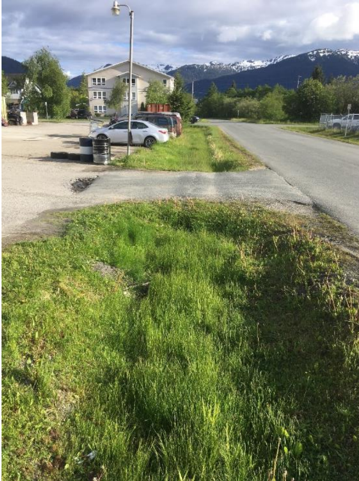
Figure 32. Stormwater swales on the east side of Alpine Ave. North. View looking south towards the Teal Street intersection in June 2020.
