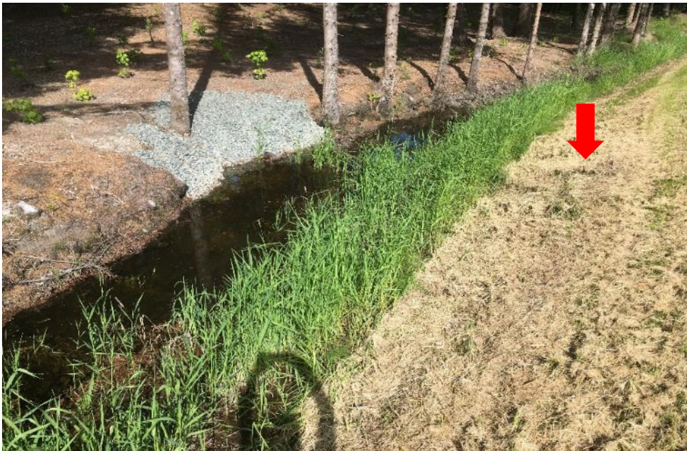
Figure 51. The outfall area of a small stormwater system at the west end of Yandukin Drive. Runoff from a stormwater outfall pipe (red arrow) collects in the ditch and enters a trench drain. The inlet of the drain is indicated by the gravel-faced embankment above. View looking east in June 2020.
