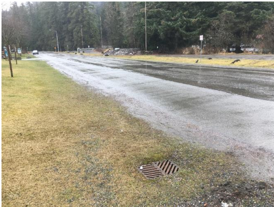
Figure 15. A catch basin near the intersection of Jordan Ave. and the south entrance to Jordan Creek Condos Loop drive. Biofiltration BMPs that encompass this and 4 other basins in the right-of-way can be constructed to provide flow control and runoff treatment. View looking north along Jordan Ave. in April 2020.
