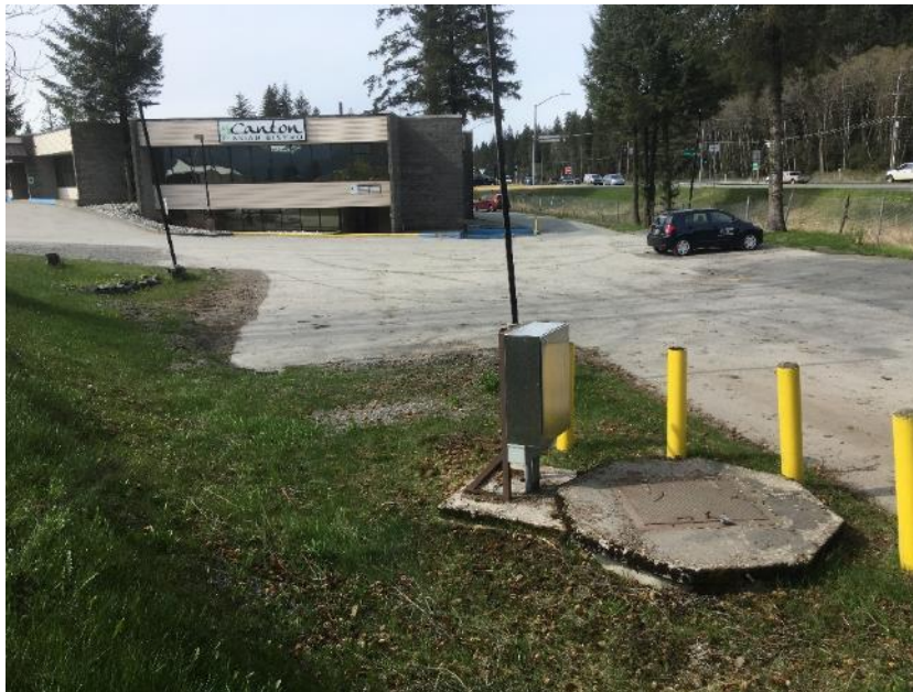
Figure 35. The Kootznoowoo parcel and building at 8585 Old Dairy Road. Stormwater runoff collected in 5 catch basins on the parcel flows to a sump (lower right of photo) and is then pumped into stormwater system 10.
