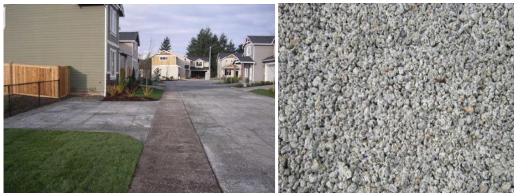
Figure 3. Left: pervious concrete sidewalk, driveways, and a street in a residential setting. Right: pervious concrete closeup. (Washington Stormwater Center LID Training Manual)
