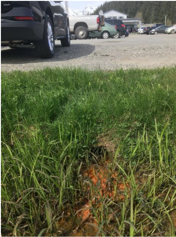
Figure 31. The outlet of a pipe connected to two catch basins in a parking area on the west side of the Toyota-Honda dealership. The Teal Street ditch is in the foreground and flows to the right. View looking north in June 2020.
