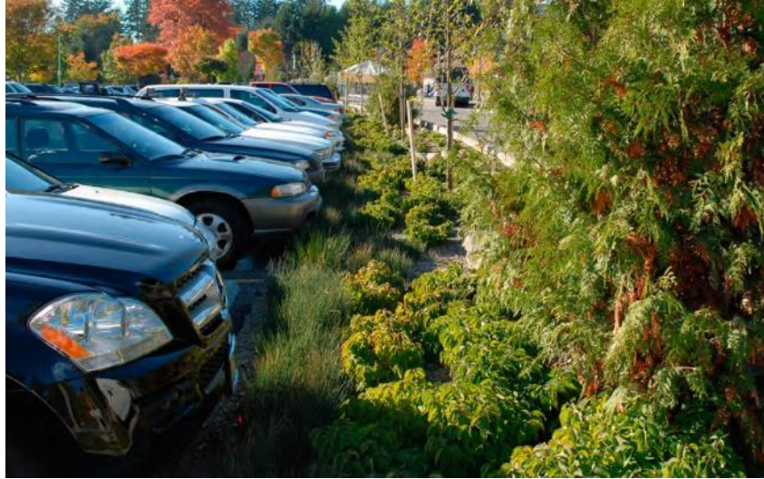
Figure 25. A vegetated filter strip in a parking lot at the Oregon Zoo.
