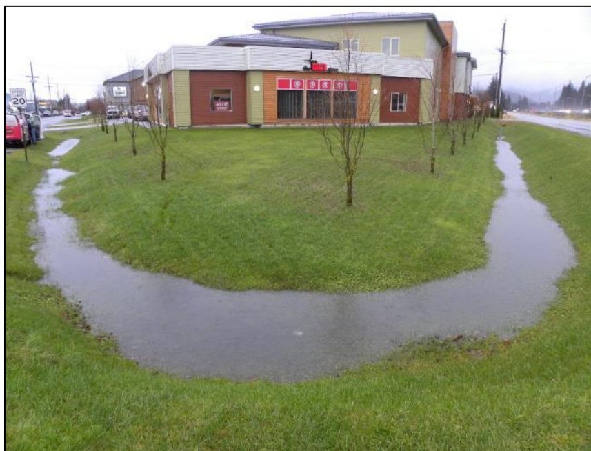
Figure 21. Panoramic photo of a biofiltration swale at the intersection of Airport Blvd. and Old Dairy Road in October 2014. Swale inlet pipes are at top of photo; the outlet pipe is at left edge of photo.
