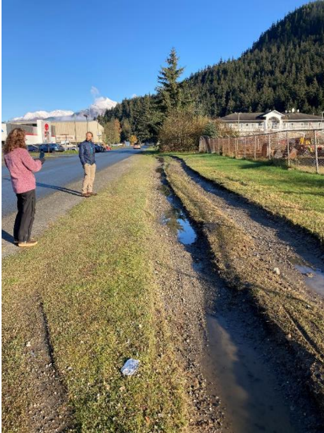
Figure 34. Ruts left by vehicles driving in the Crest Street right-of-way. View looking north between Teal Street and Airport Blvd. in October 2020.
