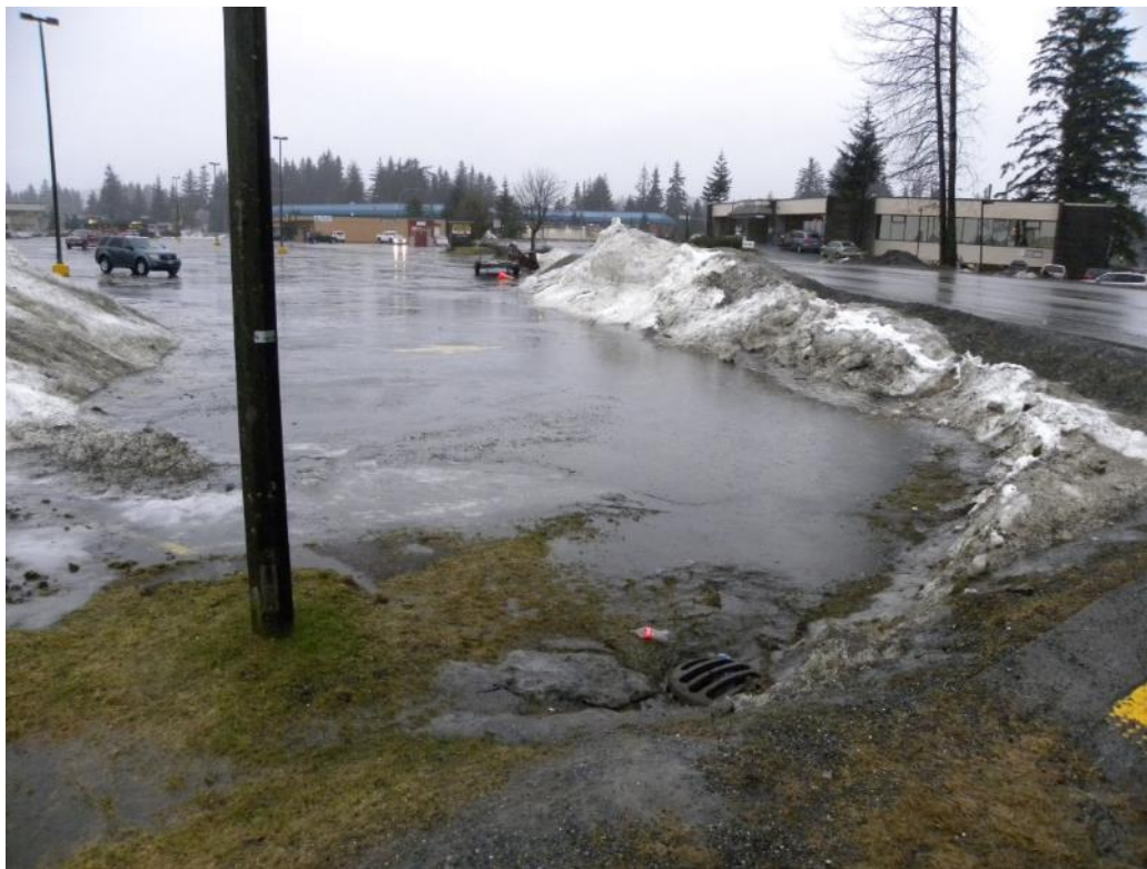
Figure 1. Rain and melted snow from a parking lot flow into a catch basin at the intersection of Old Dairy Road and Crest Street in the Lower Jordan Creek watershed. January 2013.
