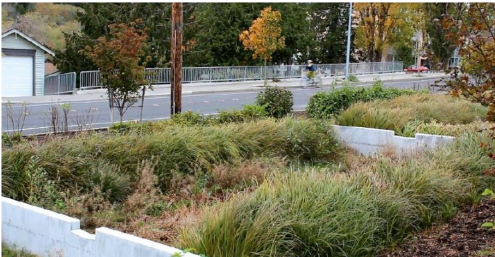
Figure 15. A series of bioretention swales. Check dams between cells impound and convey water to the downstream cell. (Washington Stormwater Center Training Manual)
