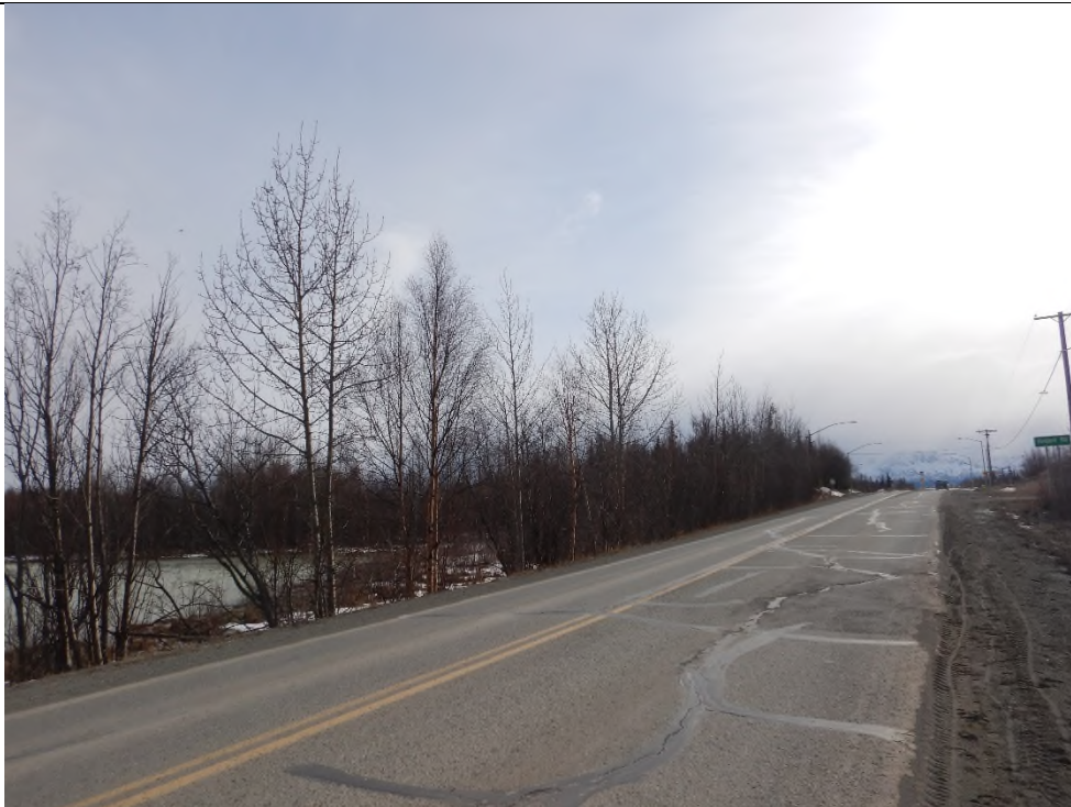
Shallow ditches along North 49th State Street.
