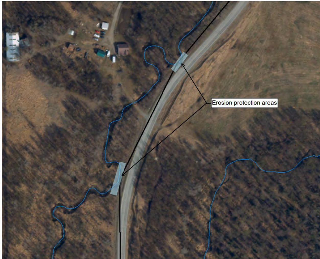
Figure 9: Wasilla Creek embankment erosion at Stringfield Road
