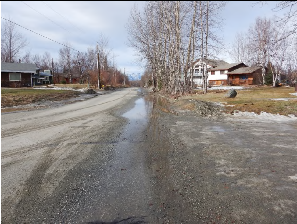
Standing water in roadway at Tern Drive.
