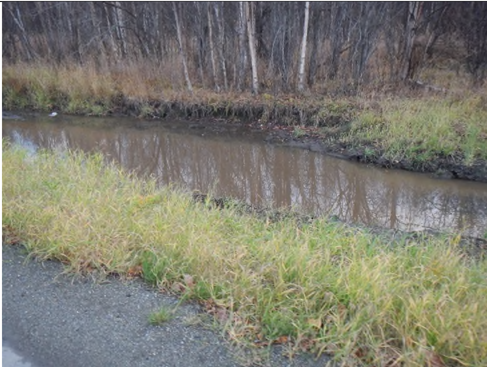
Ponding in ditches/ATV trails along Stringfield Road.
