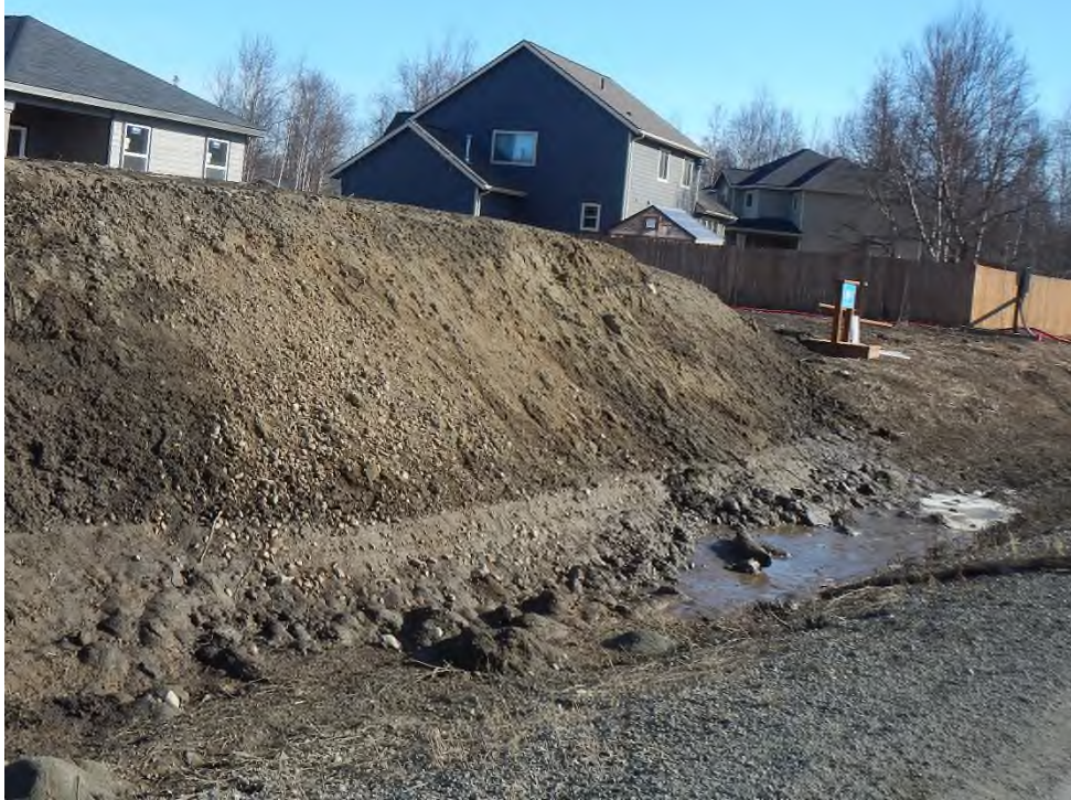
Corner of Commons and Tributary Avenue – looking east. Residential storage of large amount of material without BMPs.
