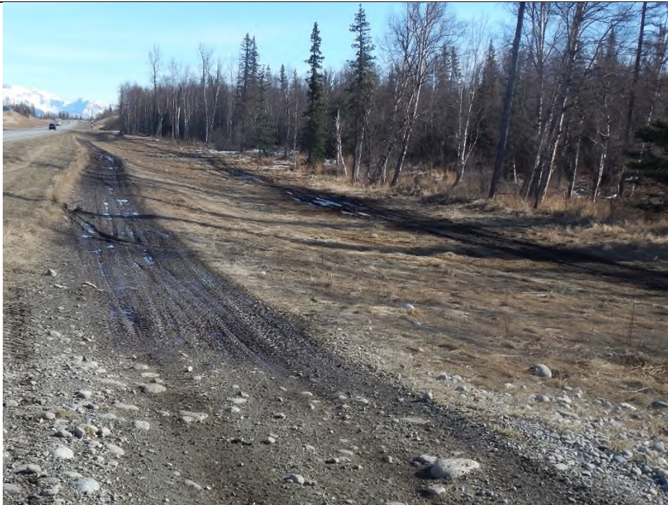
Ponding in ATV trail on east side of Trunk Road looking north.
