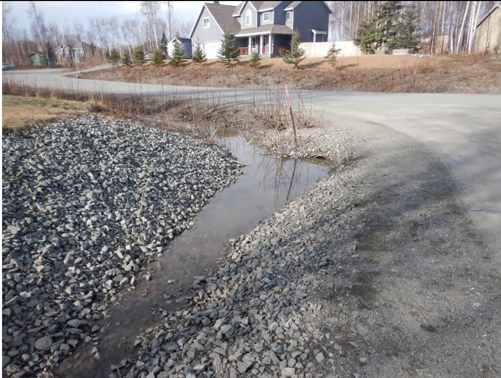
Submerged culvert at Bit Circle.
