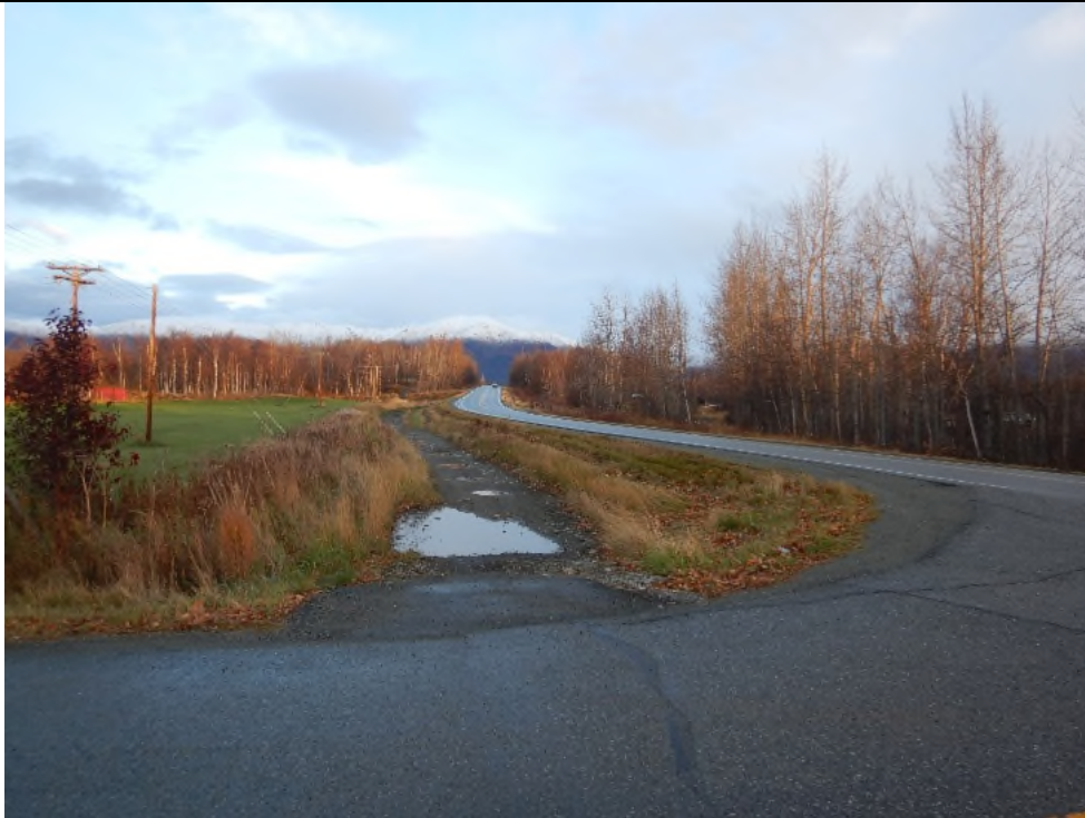
Ponding in ATV trail.
