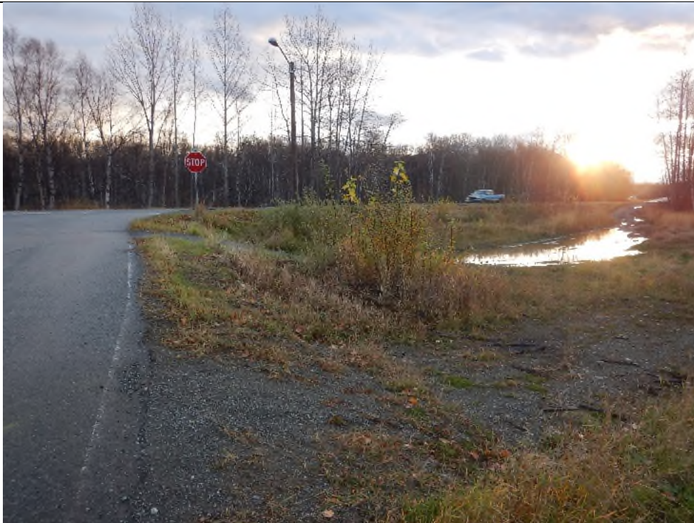
Ponding in ATV trail.
