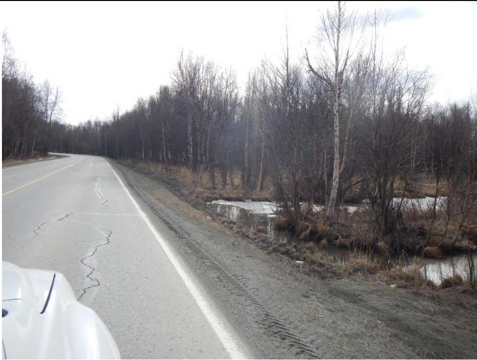
Wasilla Creek encroachment at Stringfield Road.
