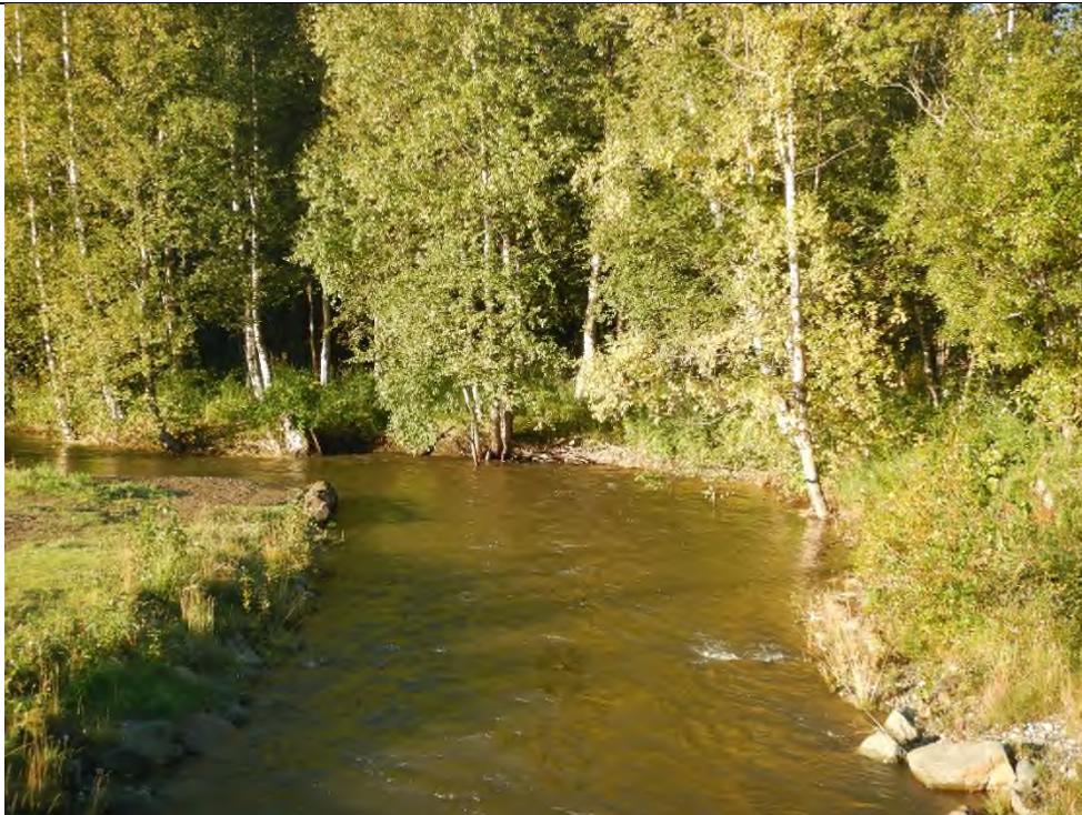
Wasilla Creek downstream streambank erosion at bend.
