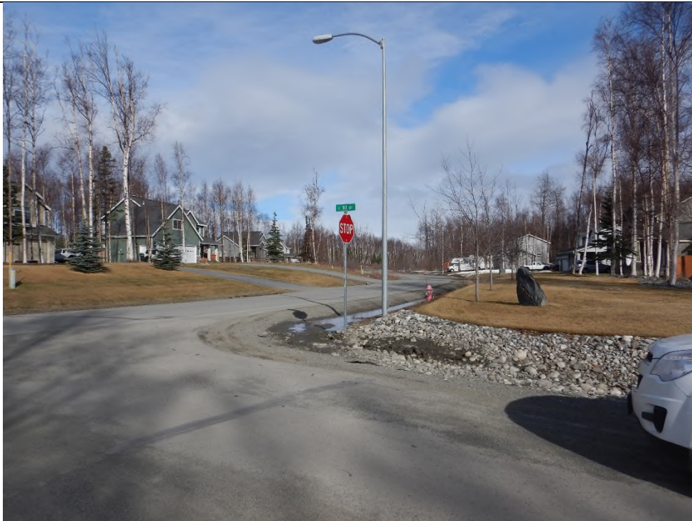
Submerged culvert at Bit Circle.
