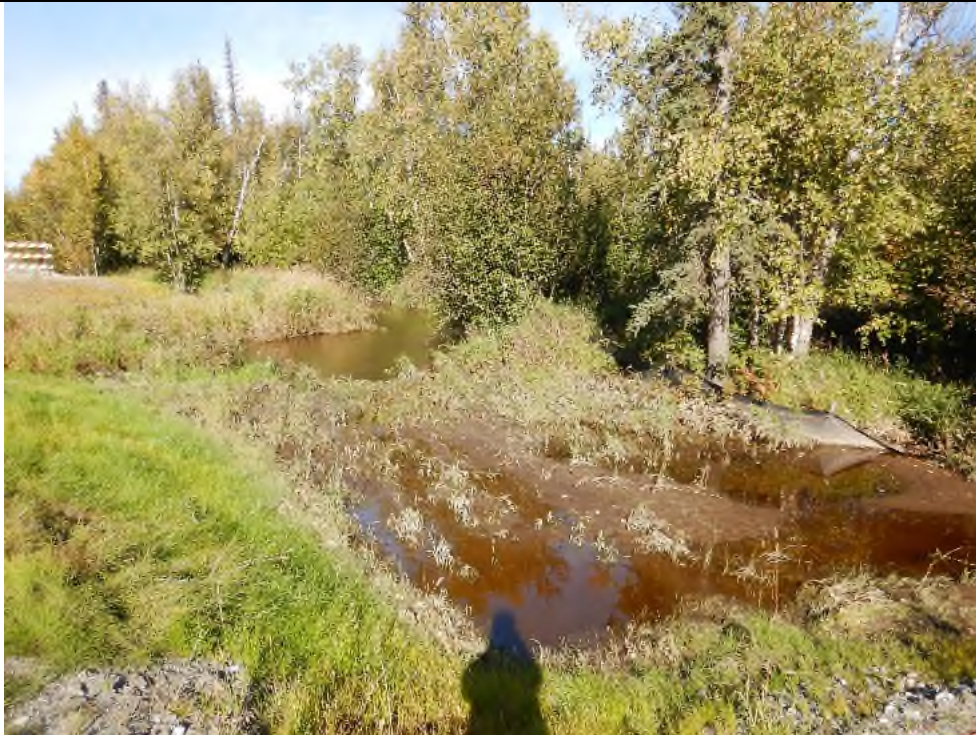
Ineffective BMPs at Nelson Drive.
