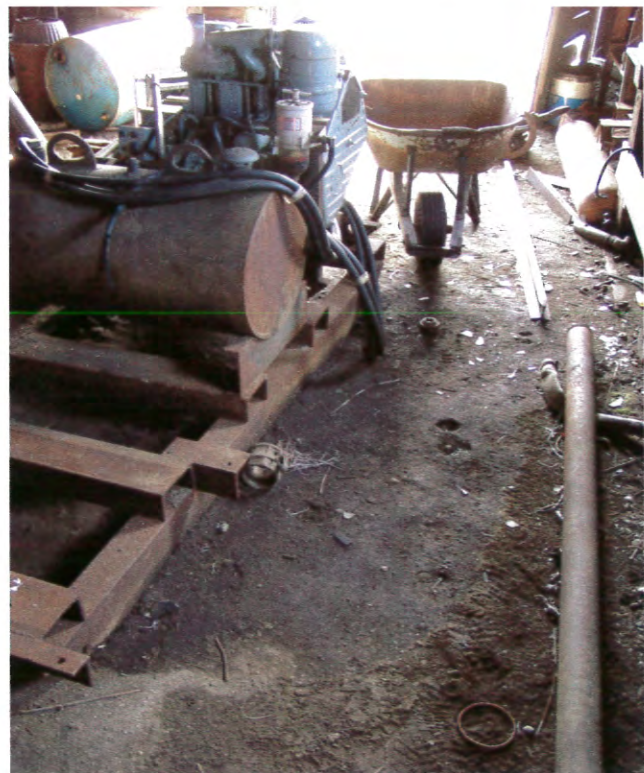
37. Building 19, south end service area.
