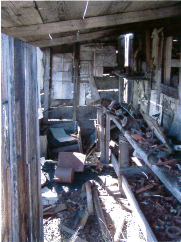
29. Building 16, coal storage and parts.
