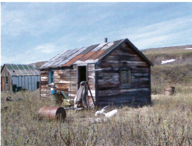
3. Building 2 (owned by Mr. Gil Barr).
