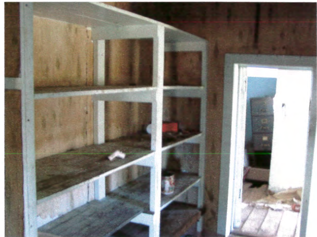
23. Building 13, kitchen pantry.
