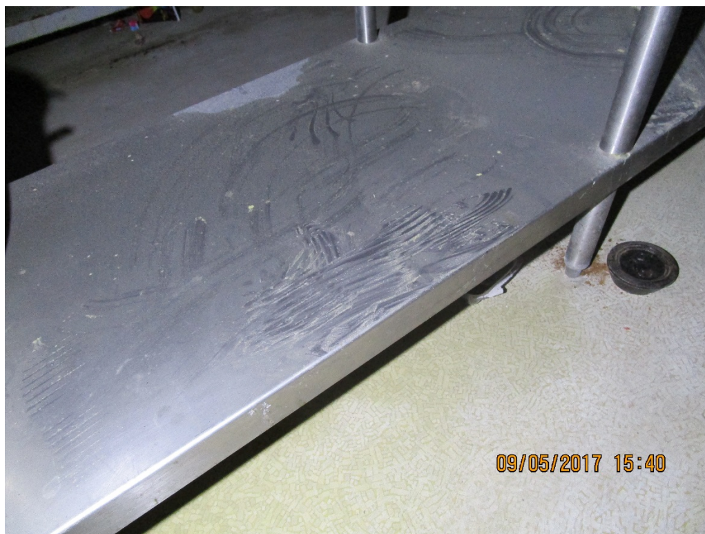
Photo 6: Another pattern of asbestos-containing sheet vinyl.
