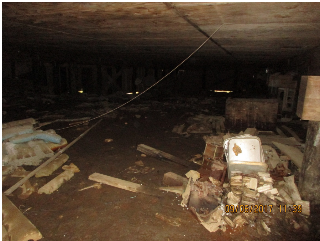
Photo 3: View under "Classroom Wing" showing typical condition of the underside of the building.
