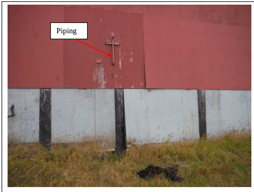
Photograph 5: Piping associated with a potential former AST located on the northern wall of the western portion of Building S1. (September 5, 2017)
