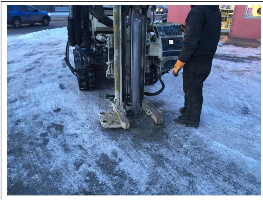
Photograph 1: Looking southwest at advancing Boring PB10. (December 8, 2016)
