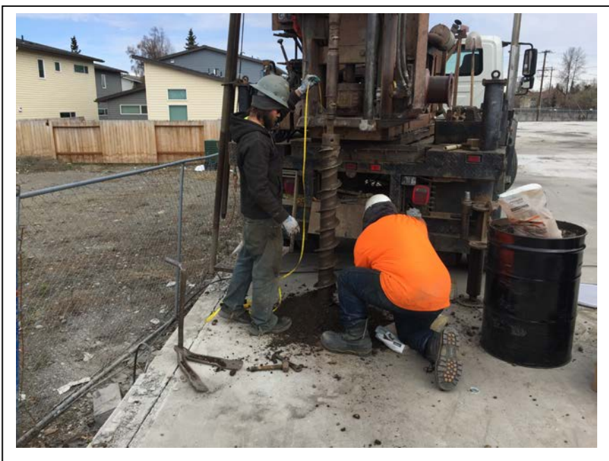
Photograph 6: Looking north at advancing Boring SW-2. (May 4, 2017)
