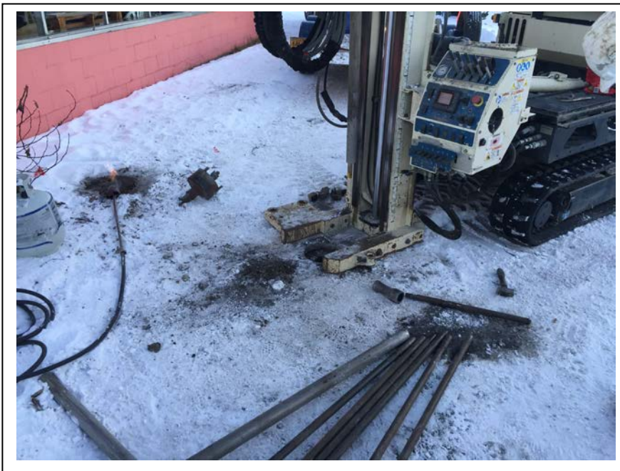
Photograph 3: Looking northeast at advancing Boring PB12. (December 9, 2016)
