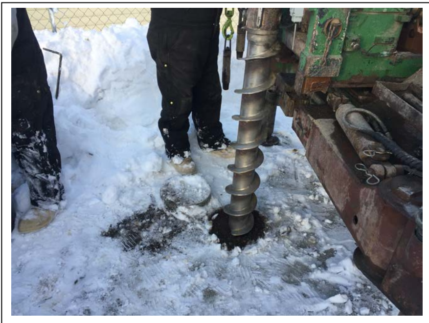
Photograph 5: Looking west at advancing Boring SW-1. (January 26, 2017)
