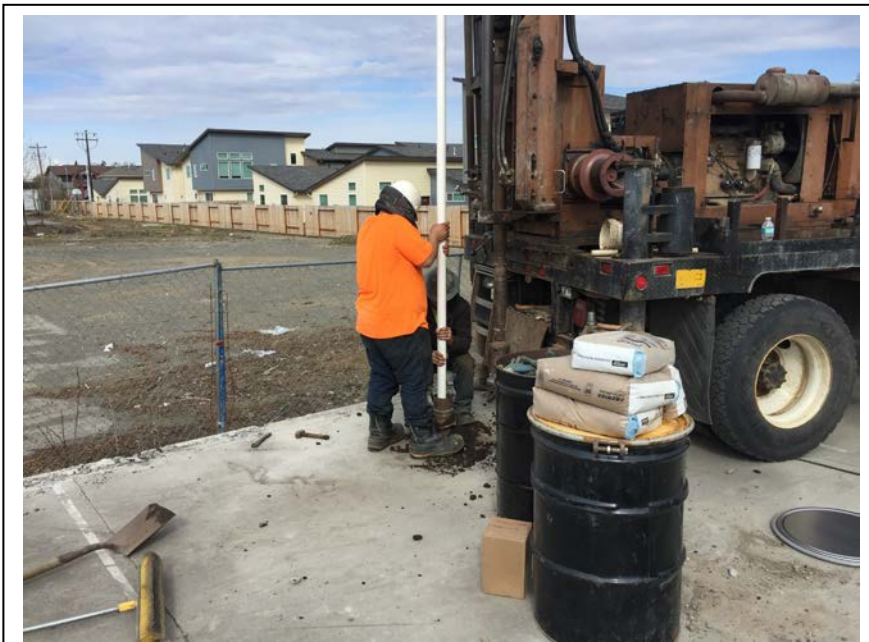
Photograph 8: Looking northwest at installing Monitoring Well SW-2. (May 4, 2017)
