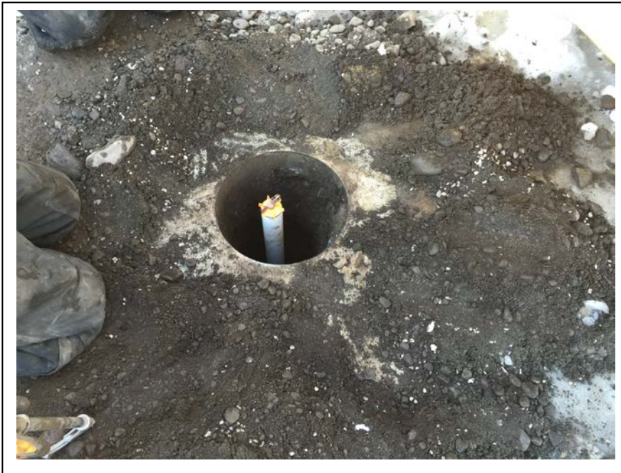
Photograph 7: Looking down at Monitoring Well SW-1. (January 26, 2017)
