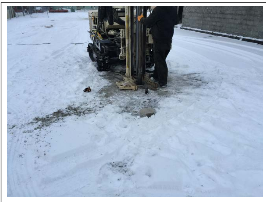
Photograph 4: Looking north at advancing Boring PB4. (December 9, 2016)
