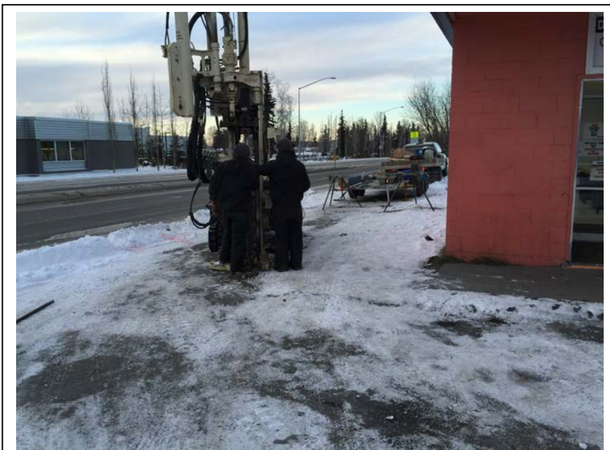
Photograph 2: Looking southwest at advancing Boring PB11. (December 8, 2016)
