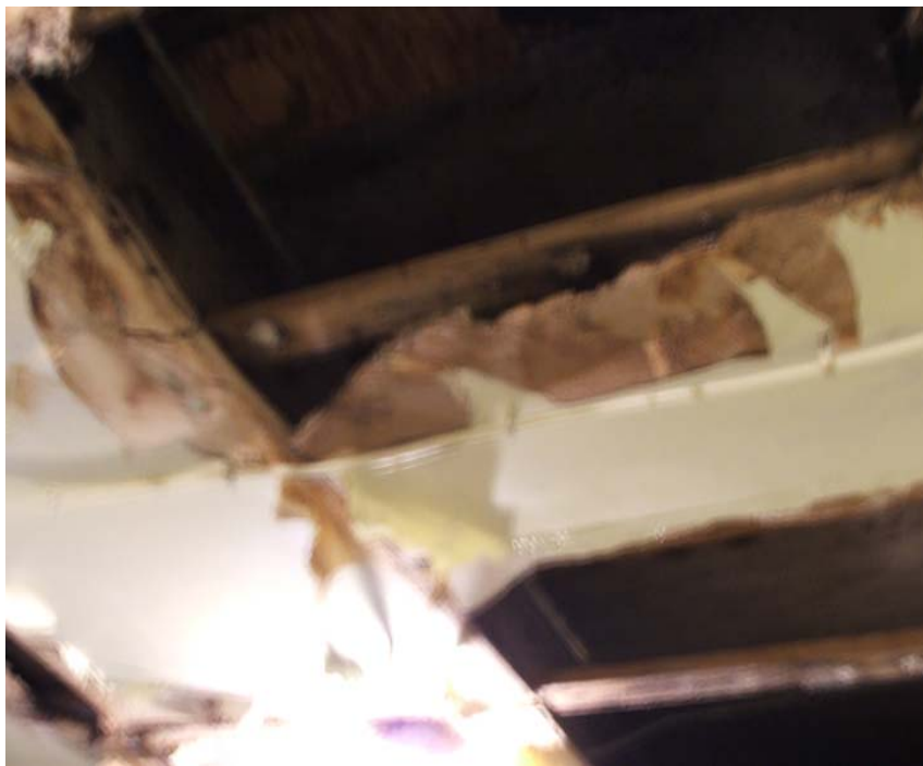
Missing ceiling panels in backroom along the east side of the building
