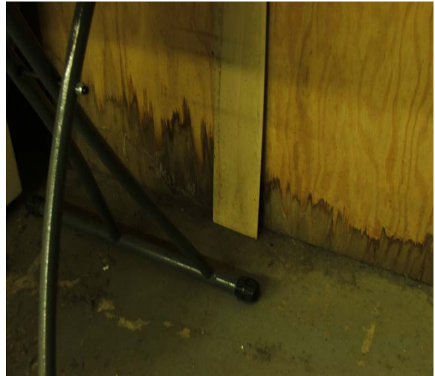
Interior wall (east side) of LFJ Manufacturing, note staining at base of wall.
