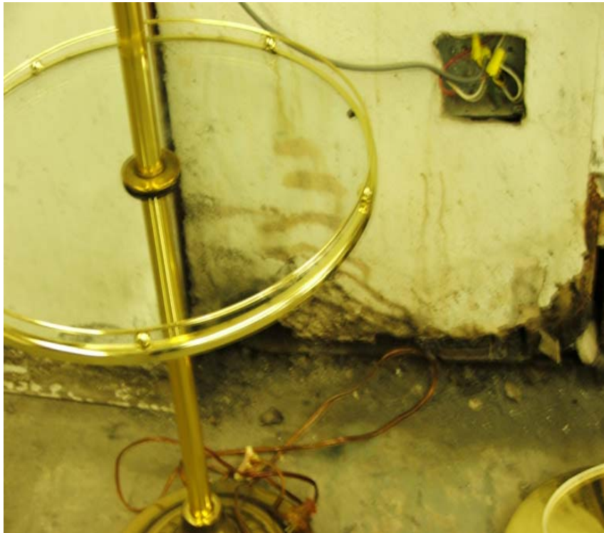
Interior wall of LFJ Manufacturing, note staining and dry wall damage.
