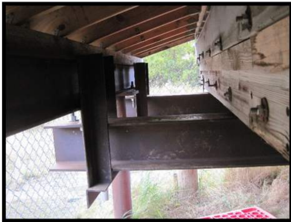
11. Foundation Modification at North Edge of Original Building - 2
