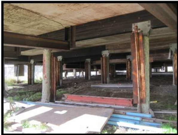
13. Foundation Modification at South Edge of Original Building - 1
