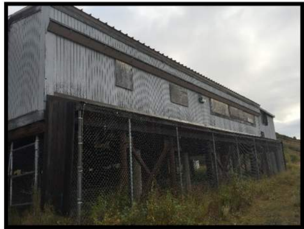
8. South Wall of Academic Room
