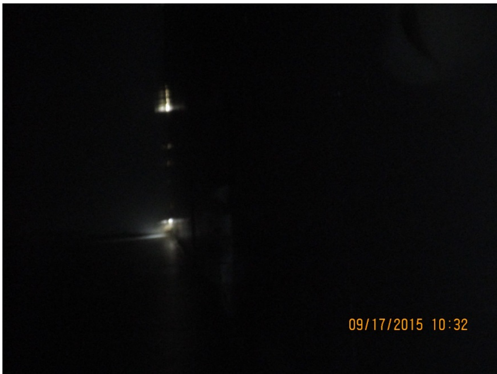
Daylight is visible through cracks at the wall/ceiling connection at the northeast corner of the Gym. Water has been intruding through these cracks causing damage to the ceiling, wall, and floor below.
