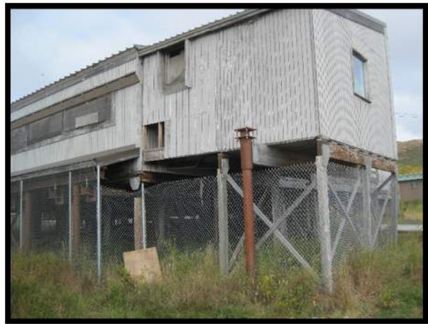
4. Cold Storage Room
