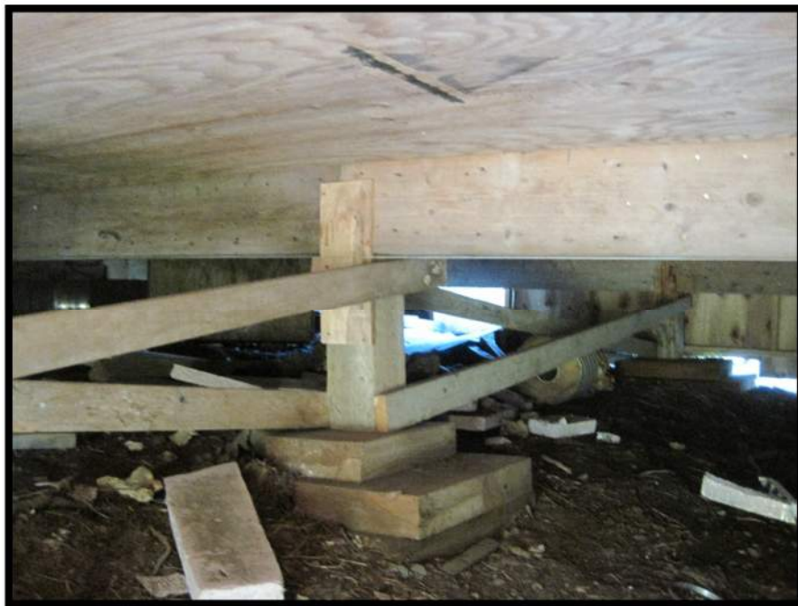
40. Typical Housing Unit Foundation
