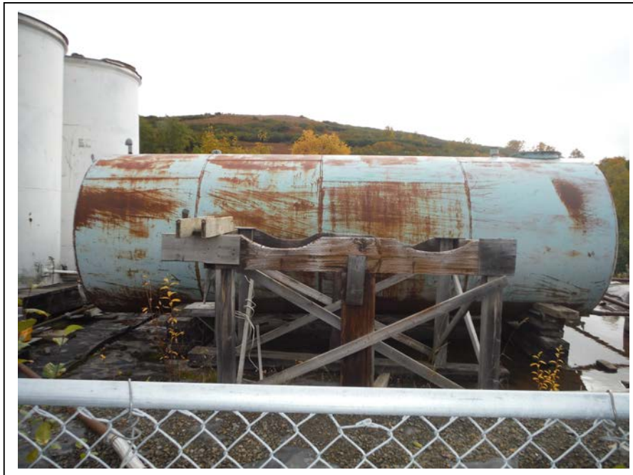
Photo 7: Looking east at Tank Farm wood support of former School ASTs. (September 16, 2015)
