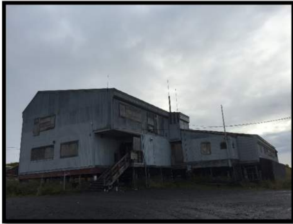
9. View Looking NE
