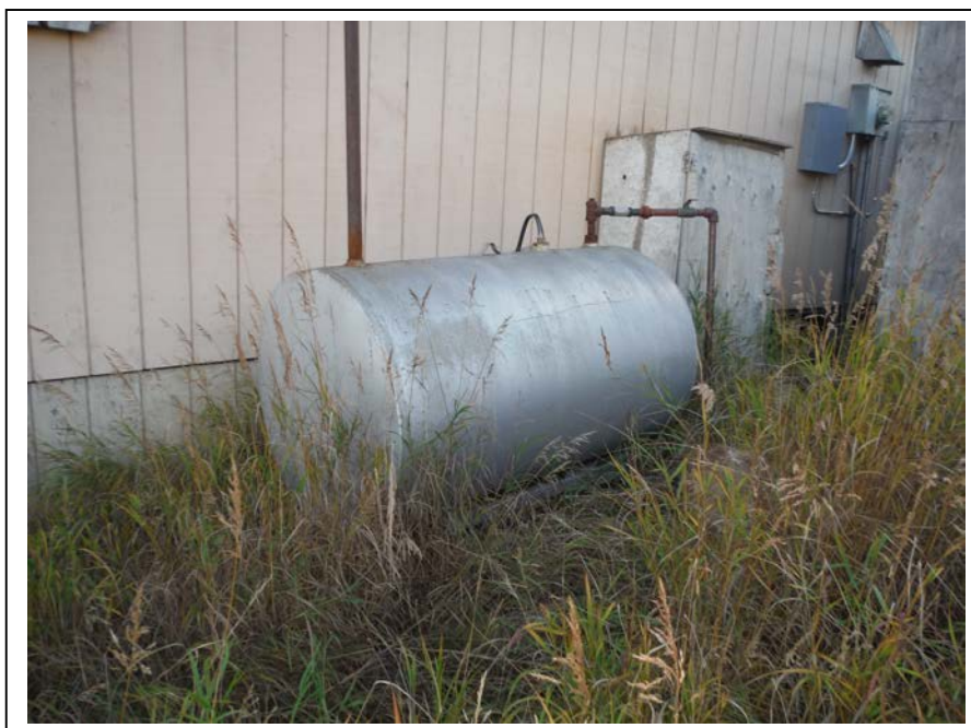
Photo 12: Looking southwest at AST9 located on the north side of Teacher Housing Building #2. (September 16, 2015)
