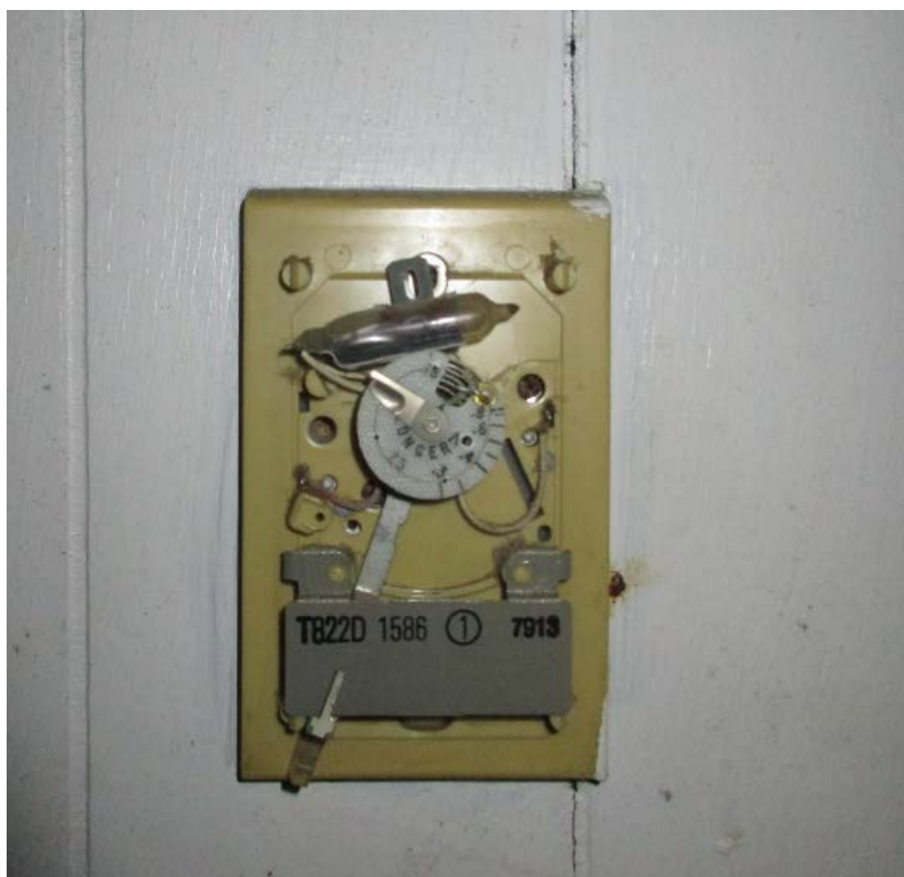
Thermostat with mercury filled ampule in Teacher Housing Unit 2.
