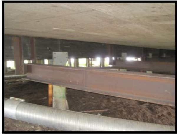
10. Foundation Modification at North Edge of Original Building - 1
