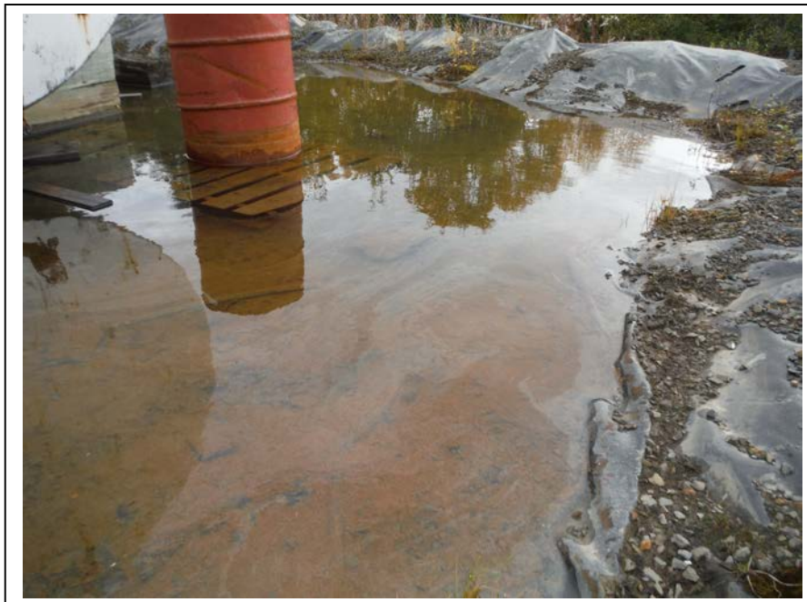
Photo 8: Looking south at the southeast corner of the Tank Farm. A sheen was present on the surface water ponded within the lined Tank Farm. (September 16, 2015)
