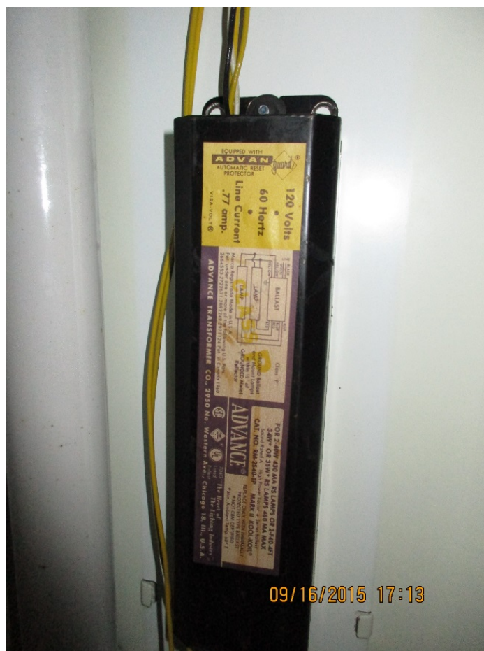
PCB containing ballast in a fluorescent light fixture in the Kitchen in Teacher Housing Unit 2.
