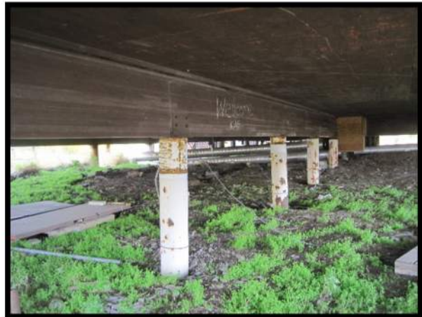
14. Steel Pipe Pile Foundation at Addition
