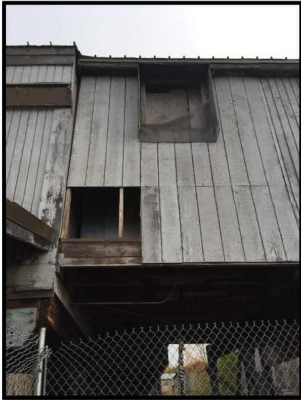
5. Cold Storage Room – Separation of Structure From Existing Building
