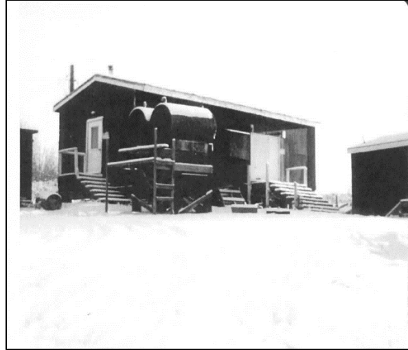
FIGURE 7 – FORMER GENERATOR BUILDING, SHOWING FORMER ASTS
