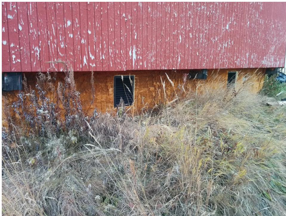
Photo 28 – Vents installed in crawlspace skirting
