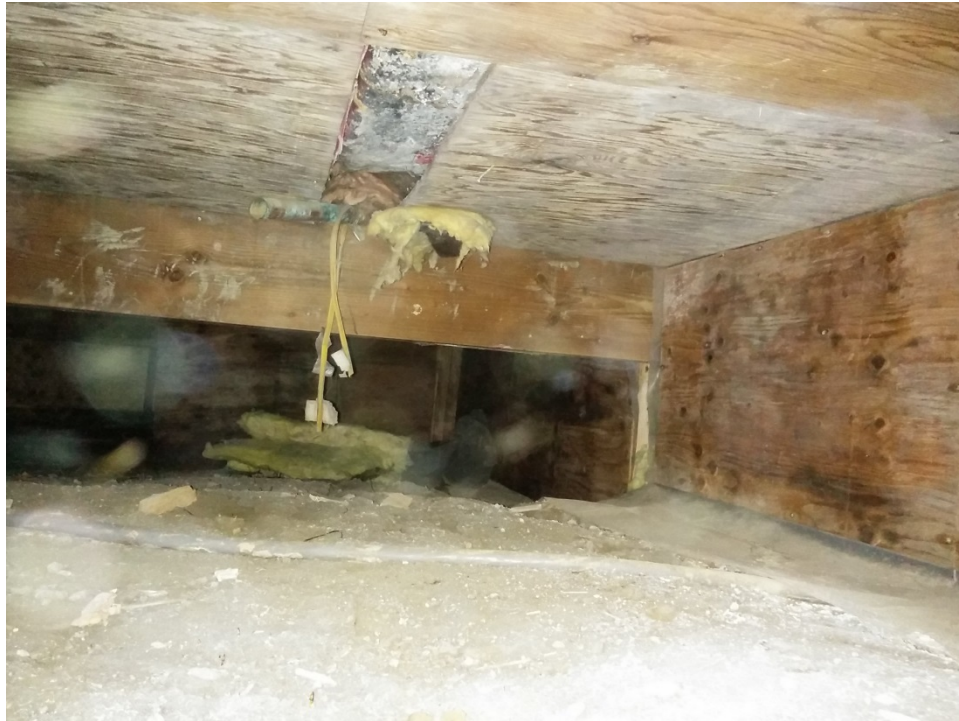
Photo 27 – Crawlspace under northeast end of building
