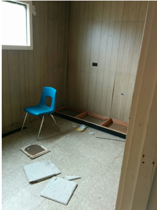
Photo 9 – Classroom in northeast end of building
