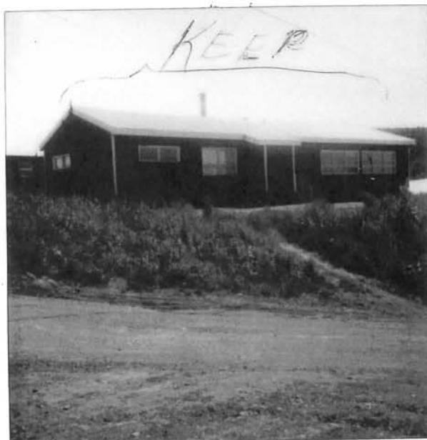
Keep newer portion of School building
