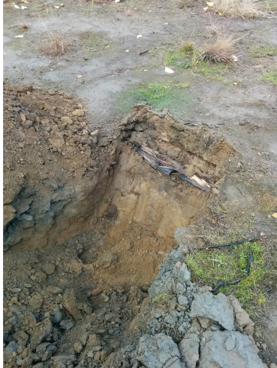
Photo 13 – Possible tank support in former generator building area
