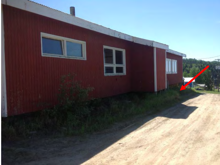
Photograph 2 View to west on north side of building. Possible UST location indicated by arrow.
