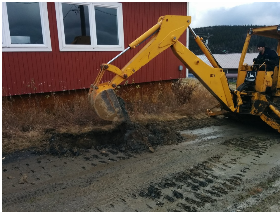
Photo 16 – Excavating test pit TP-02
