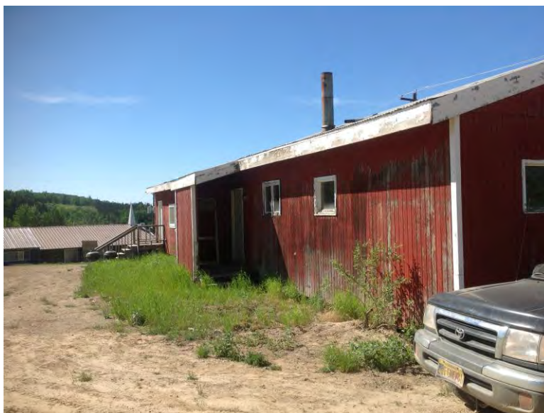
Photograph 1 View to west on the south side of the "Old Headstart Building"
