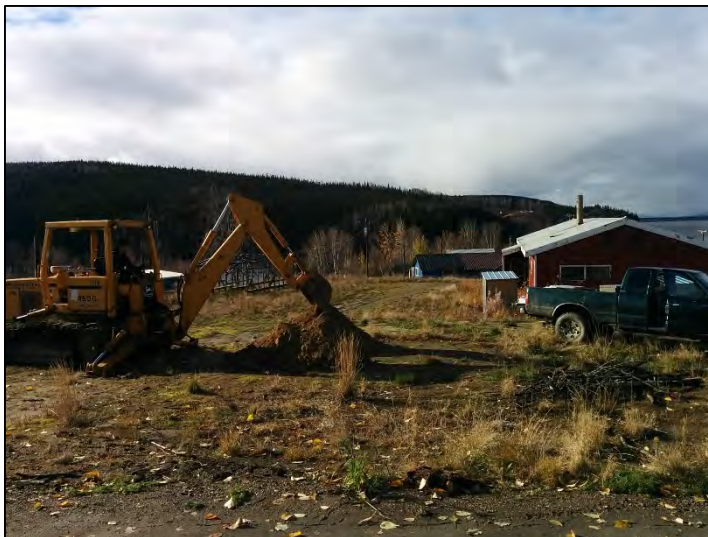
FIGURE 10 – TEST PIT IN FORMER AST AREA
