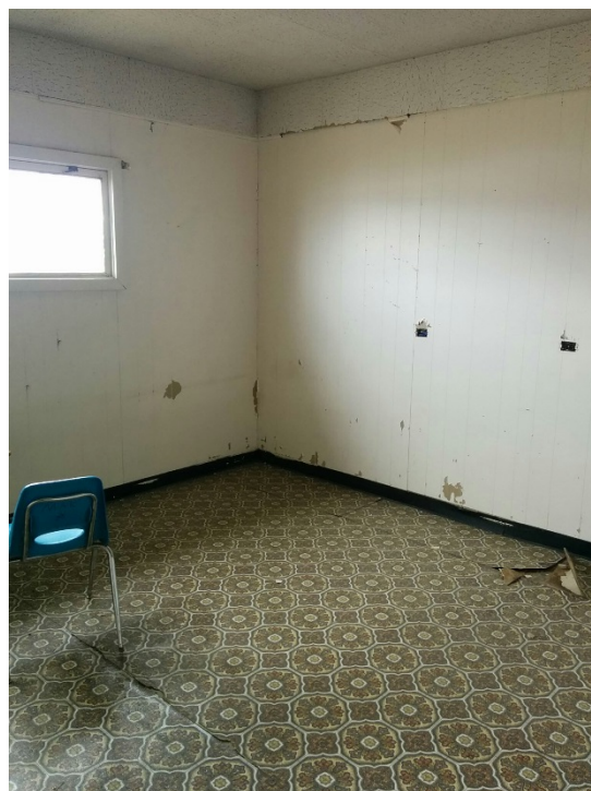
Photo 8 – Classroom in northeast end of building
