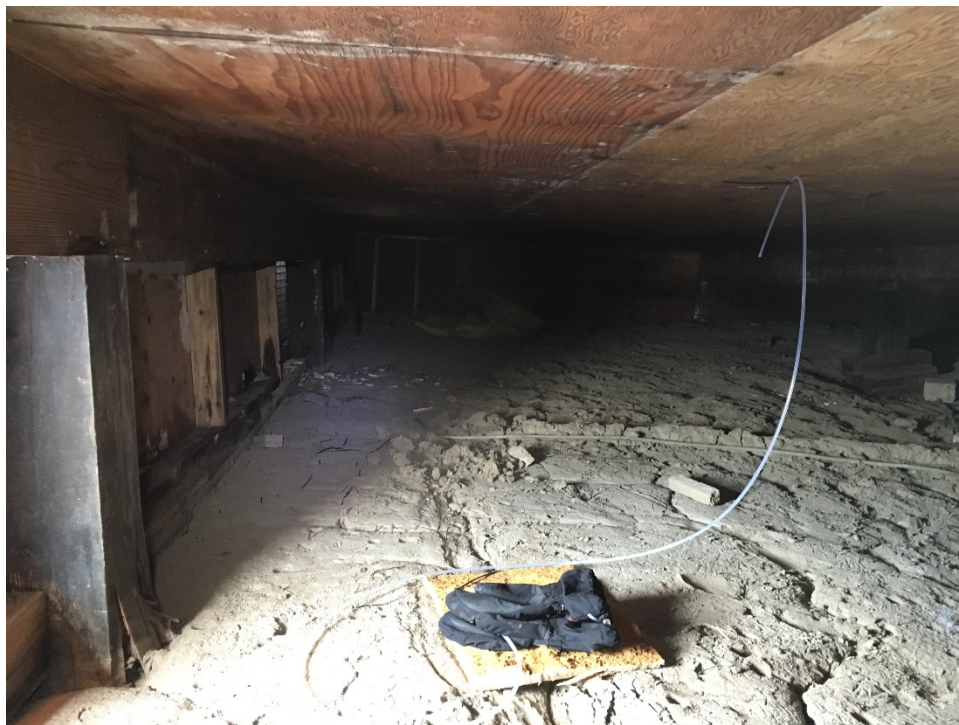
Photo 37 – Southwest crawlspace air sampling location
