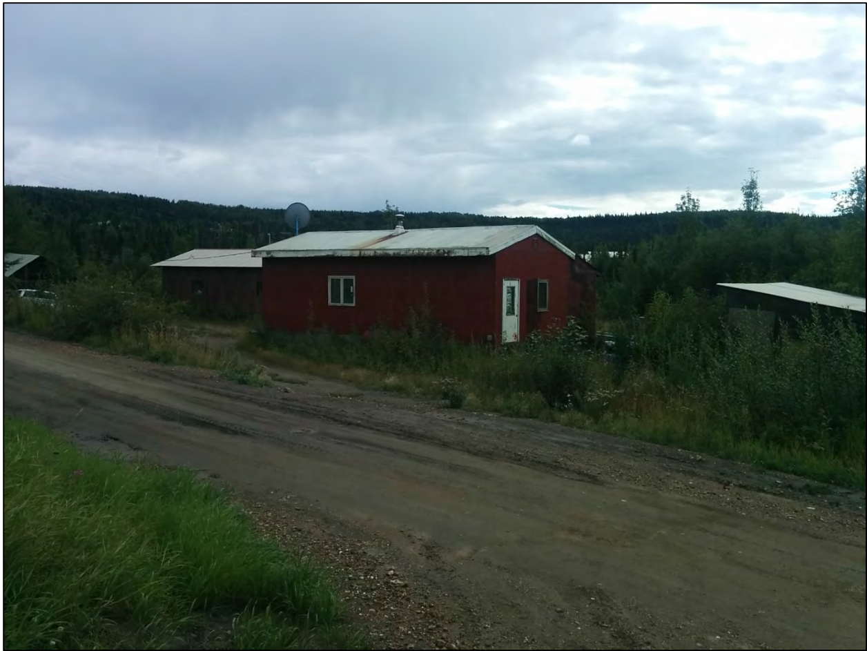
FIGURE 8 – FORMER GENERATOR BUILDING, REPURPOSED AS CABIN ON ADJOINING PROPERTY
