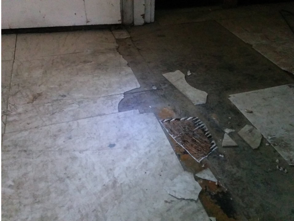
Photo 31 – Mastic for off-white tile (Room C, sample AS05, 1.2% asbestos)
