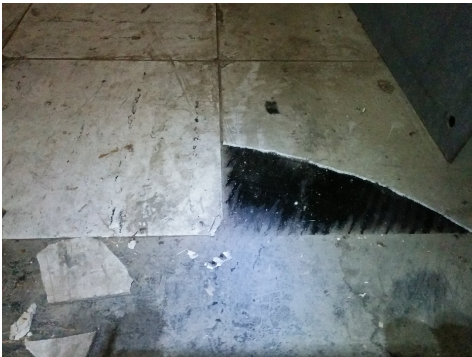
Photo 32 – Off white/black 9x9 floor tile and mastic (Room D&E, sample AS07, 1.3-3.8%)
