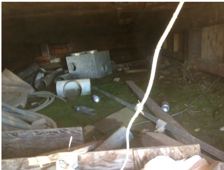
Photograph 5 View of crawl space from access point.
