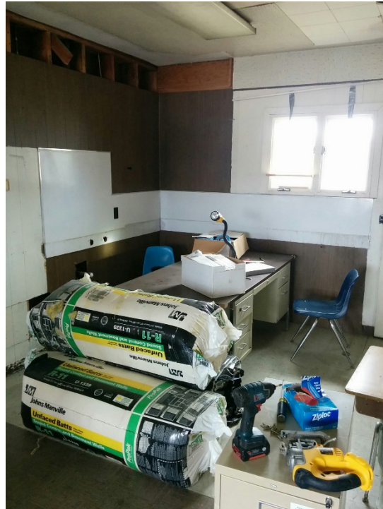
Photo 7 – Building material staged in former Headstart building
