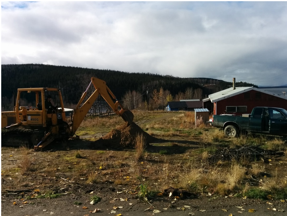
Photo 14 – Excavating test pit in former generator building area
