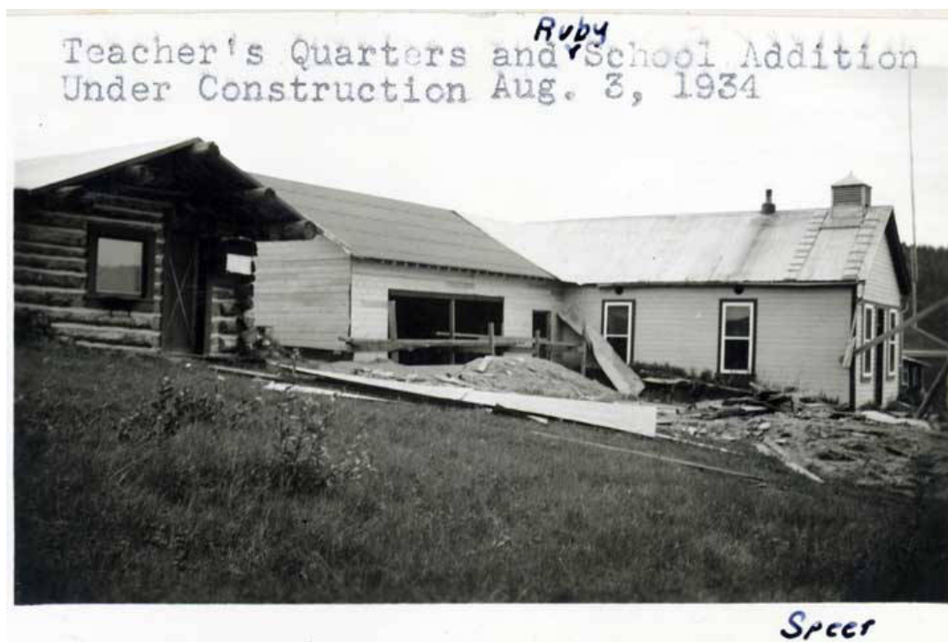
1934 Photo of Territorial School Additions Under Construction
