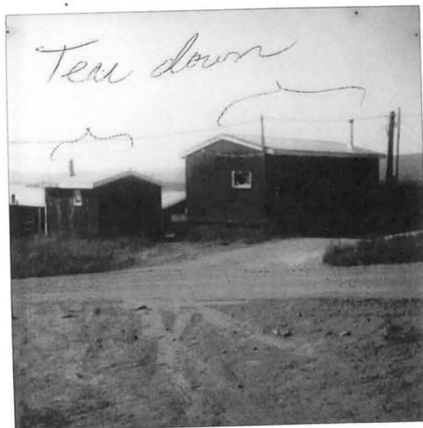
2 storage sheds (rear view)
