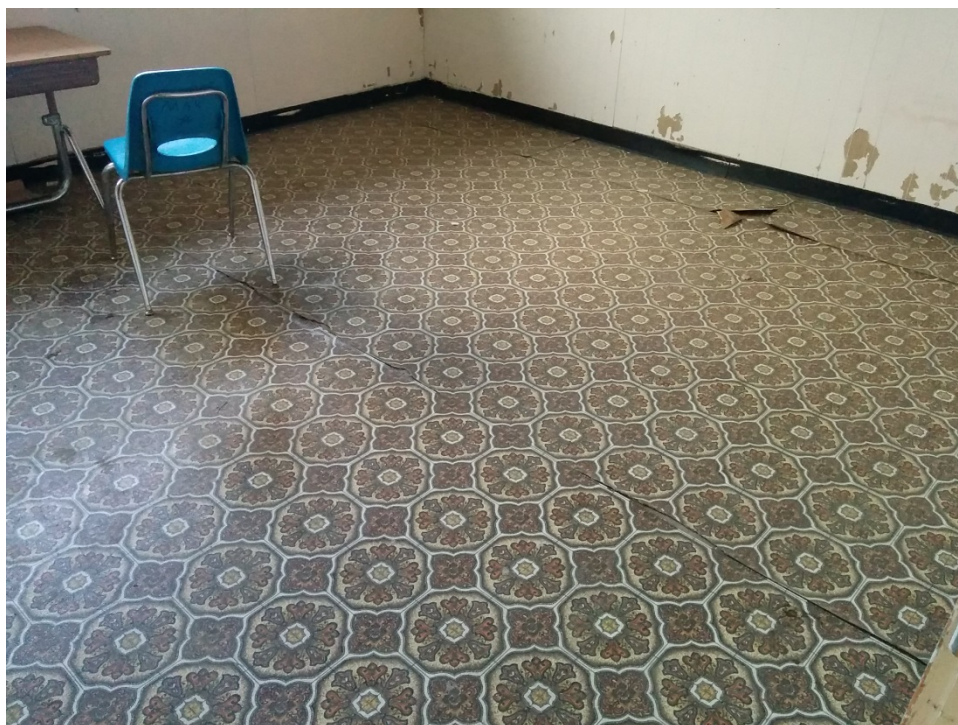
Photo 30 – Sheet vinyl (Room B, sample AS04, 25% asbestos)
