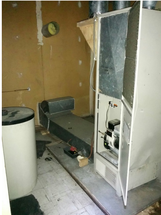
Photo 11 – Forced-air furnace
