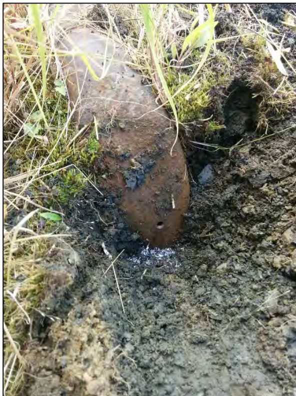
FIGURE 9 – UST FILL/VENT PIPE
