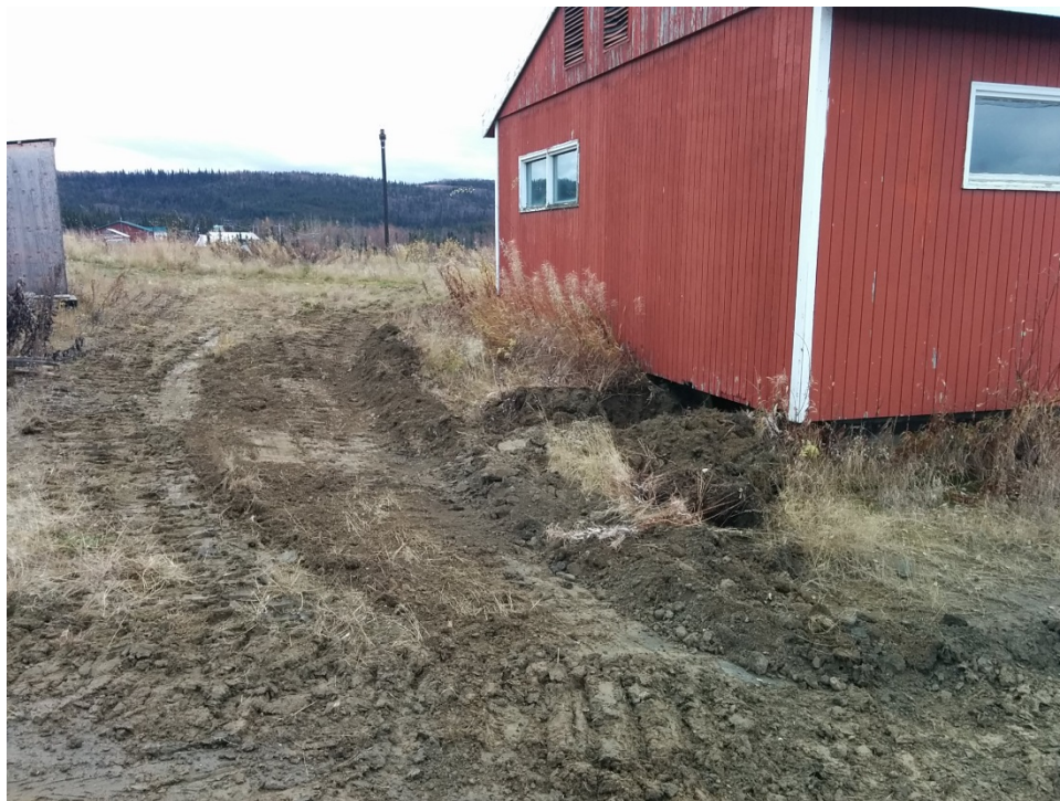
Photo 19 – Drainage improvements on northeast end of building
