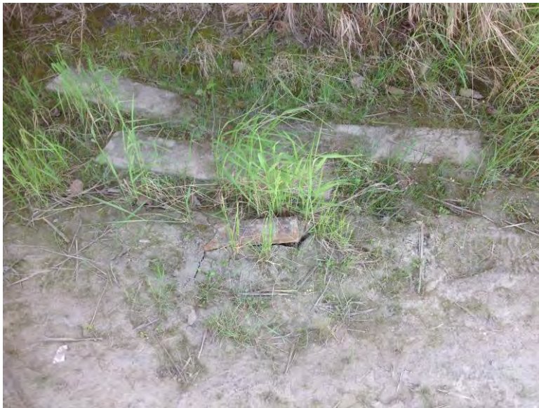
Photograph 3 Crushed pipe at possible UST location.
