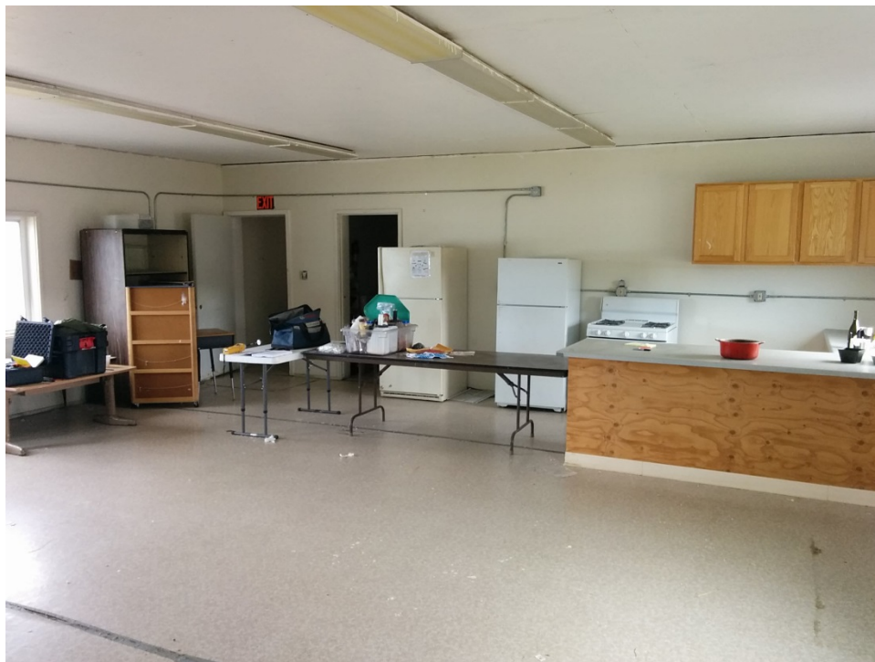
Photo 5 – Main room of former Headstart building, facing NE
