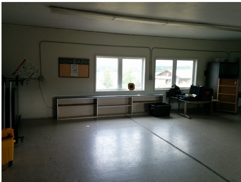
Photo 6 – Main room of former Headstart building, facing N
