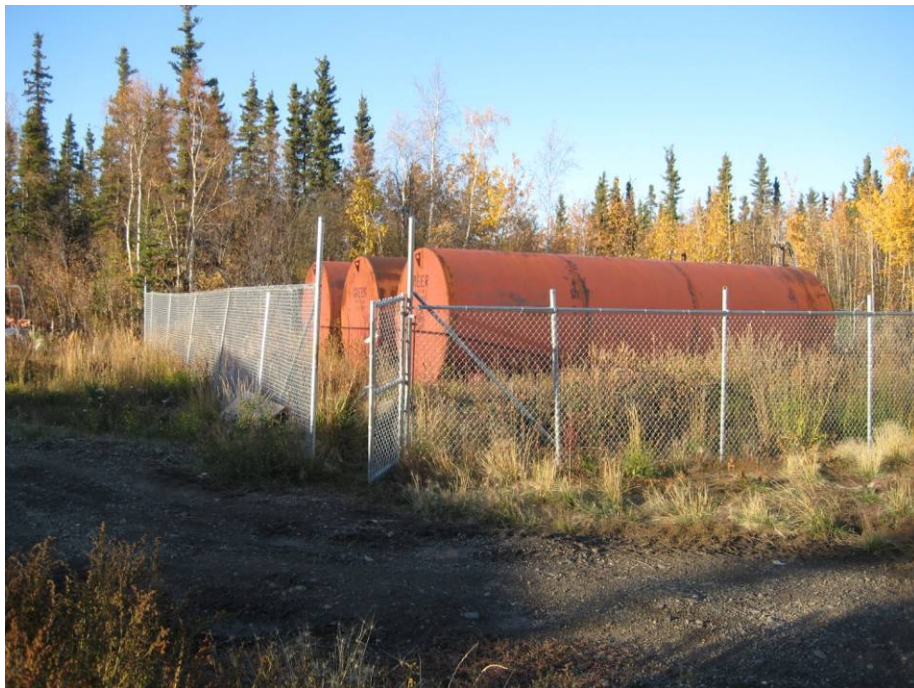
Photograph 2: The Beaver Joint Utilities (BJU) Tank Farm. The Burned Generator Building Site is left of the fence and tanks, across the path. (September 2009).
