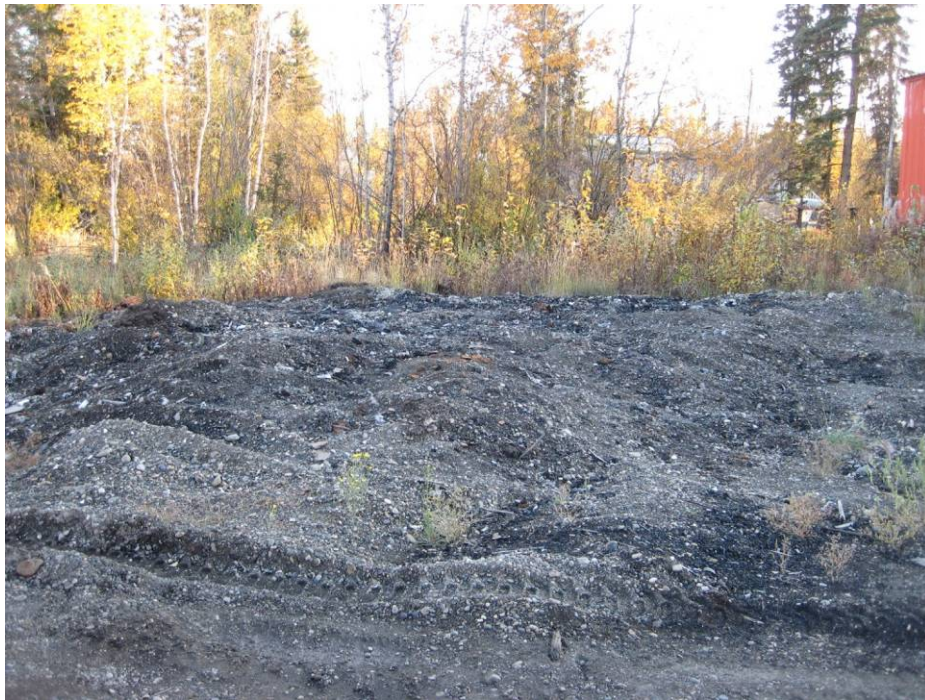
Photograph 1: The Burned Generator Building Site (September 2009).
