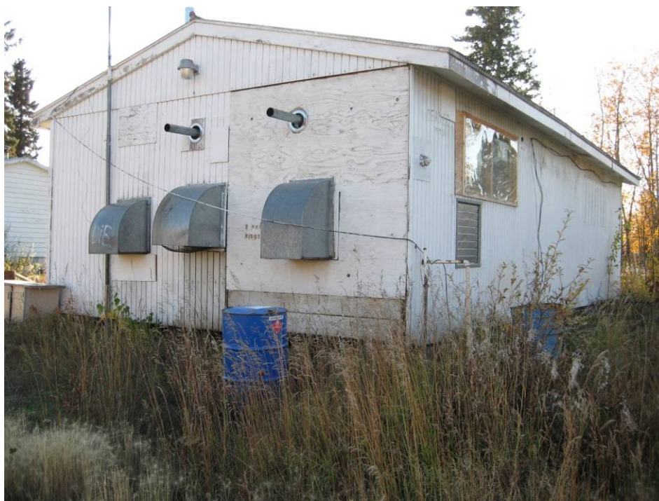
Photograph 7: Unleaded gasoline drums stored at generator building (September 2009).
