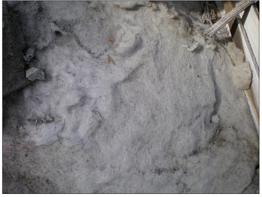
PHOTOGRAPH 4: SUSPECT MATERIAL POTENTIALLY CONTAINING ASBESTOS IN THE KITCHEN
