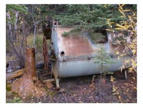
A second uncapped well casing was observed just north of the school. A storage tank is situated next to the well but appears to be disconnected. Moisture and corrosion around the well casing suggest the well may also be artesian, but it was not flowing at the time of the site visit.
