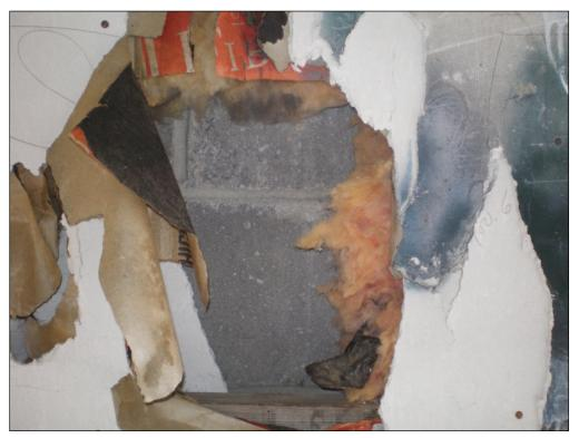
PHOTOGRAPH 26: INSULATION IN SHOP BUILDING, LIKELY FIBERGLASS, VIEW SOUTH-SOUTHWEST
