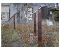
observed south of the former boiler room (see Photograph 18, Appendix E). It is unknown what the contents of the UST were and if any liquid remains in the tank. The size of the UST also is unknown; however, the tank is likely small, as the fill and vent pipes were approximately 3 feet apart. No stressed vegetation or staining was observed on the ground surface.
