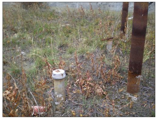
PHOTOGRAPH 18: FILL AND VENT PIPE OF UST, VIEW WEST
