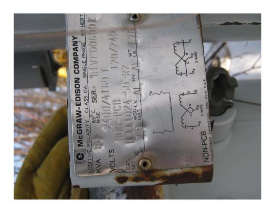
Photograph 11: Transformer ID plate identifying oils in transformer as Non-PCB (March 2010).
