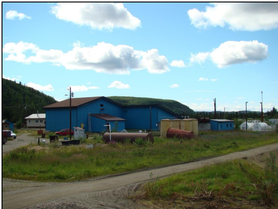
Photograph 2: School with the old tank farm (in front) and the new 6,000 gallon tanks (in rear).
