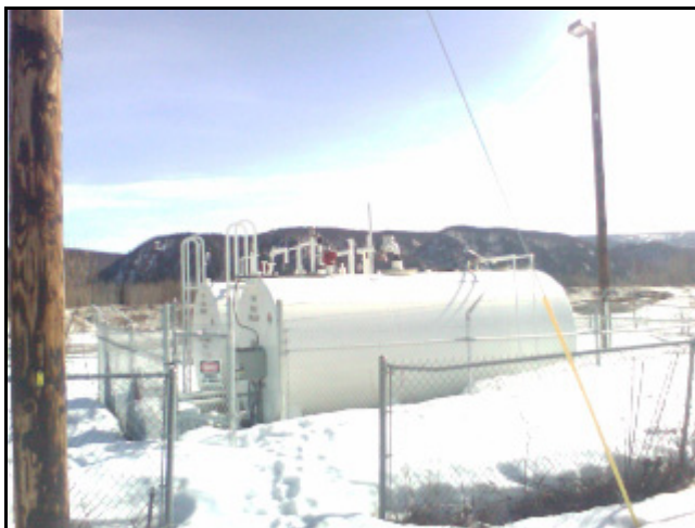
Photograph 5: Two new 6,000 gallon tanks for the school
