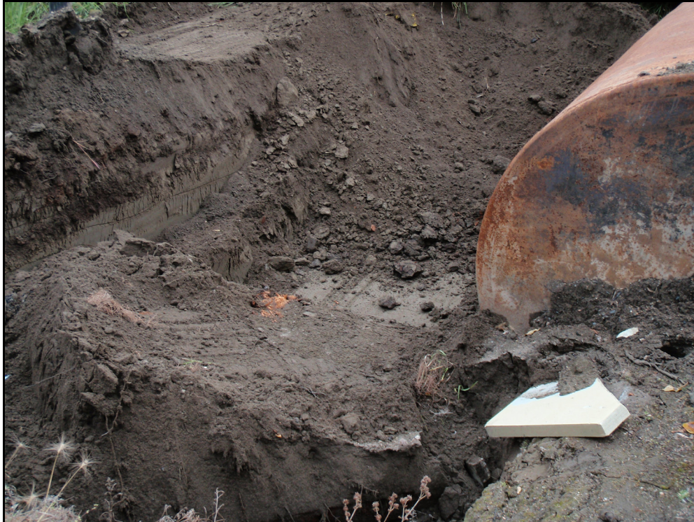
Photograph 1 – View of impacted soil being removed from around tank.
