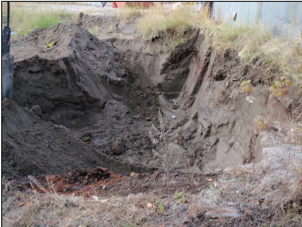
Photograph 2 – Completed excavation with tank removed.
