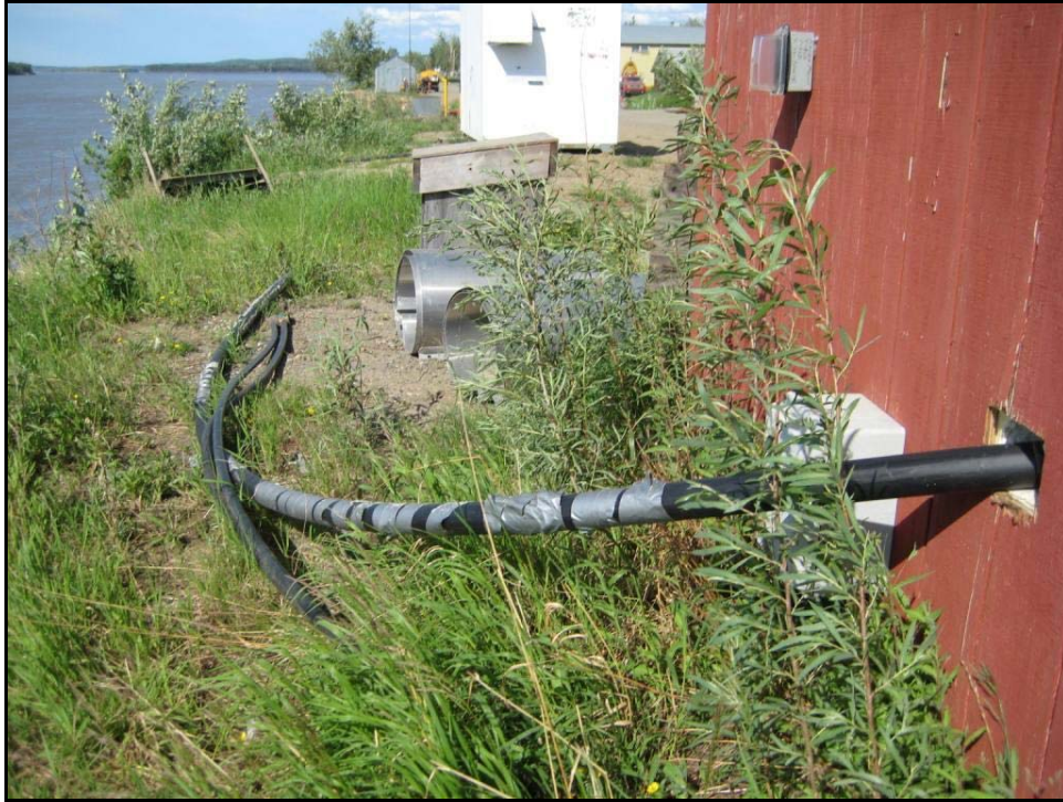
Photograph 3: Surface water collection hose. This hose collects surface water for the village during low water months.
