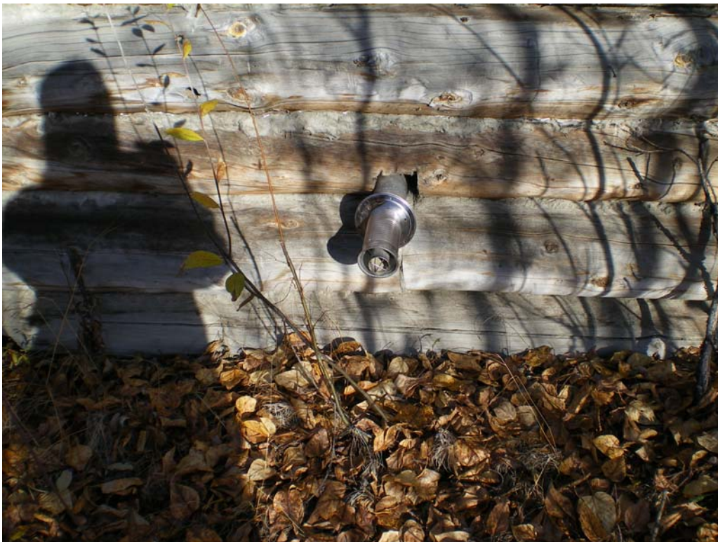
Figure 18. Monitor exhaust outlet from cabin at former village site.
