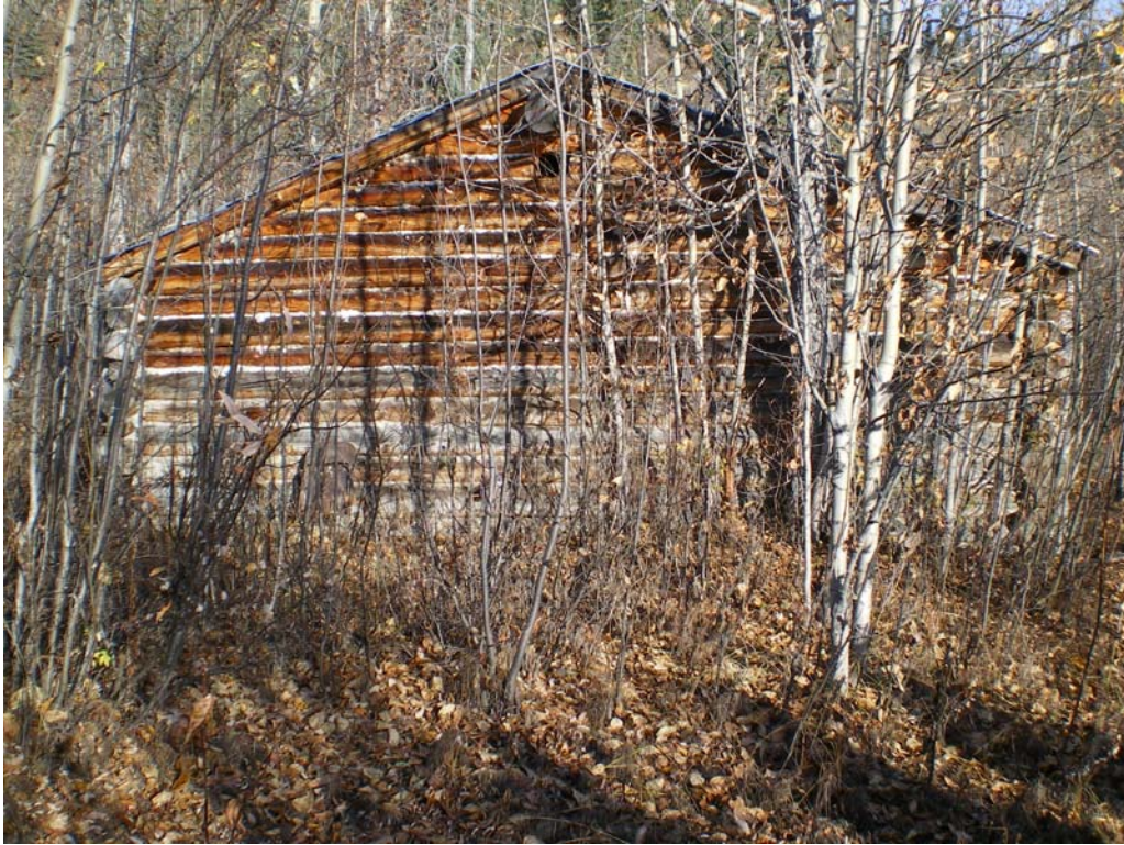
Figure A9. Flood-level marked by faded coloration on cabin at former village site.
