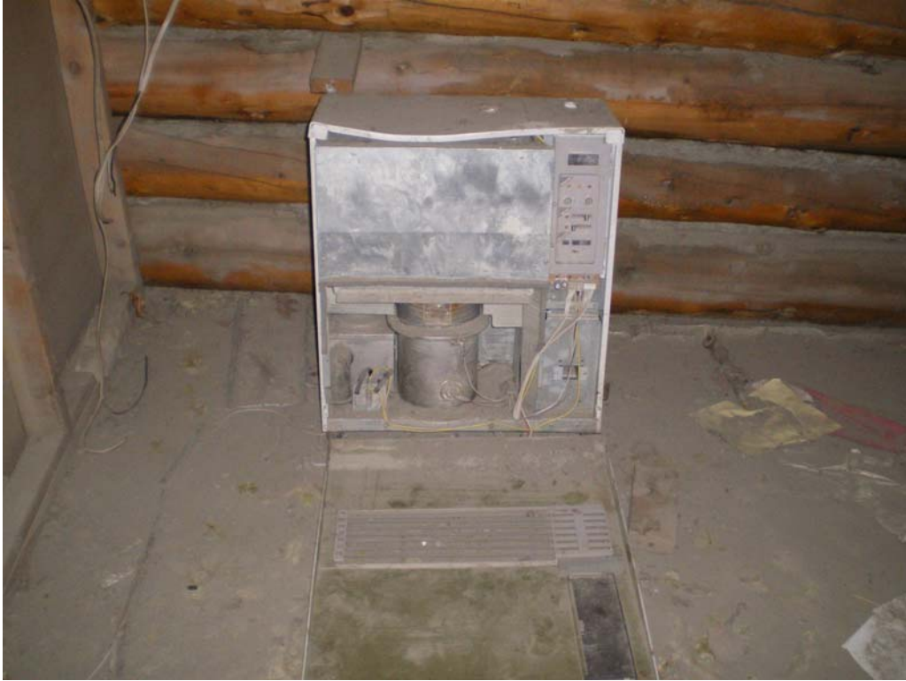
Figure 17. Monitor in cabin at former village site. This was the only cabin at the site with an oil-fueled heating system.
