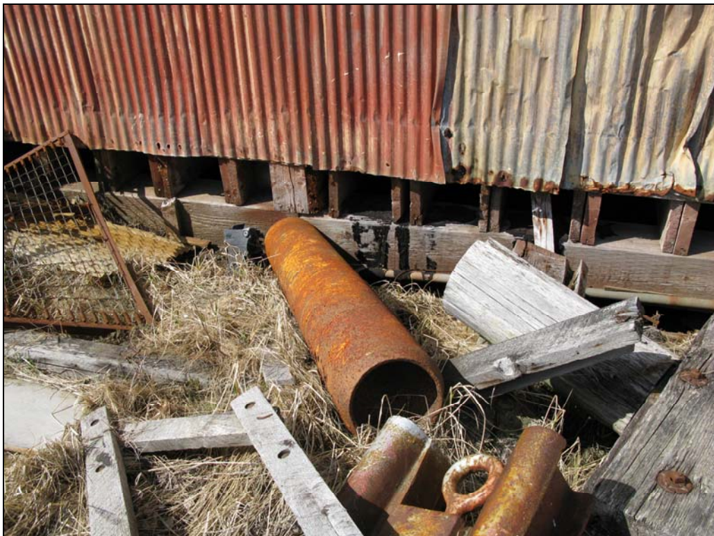
PHOTOGRAPH 12. OILY SUBSTANCES LEAKING FROM BUILDING H THAT PROBABLY ORIGINATED FROM WITHIN THE BUILDING.
