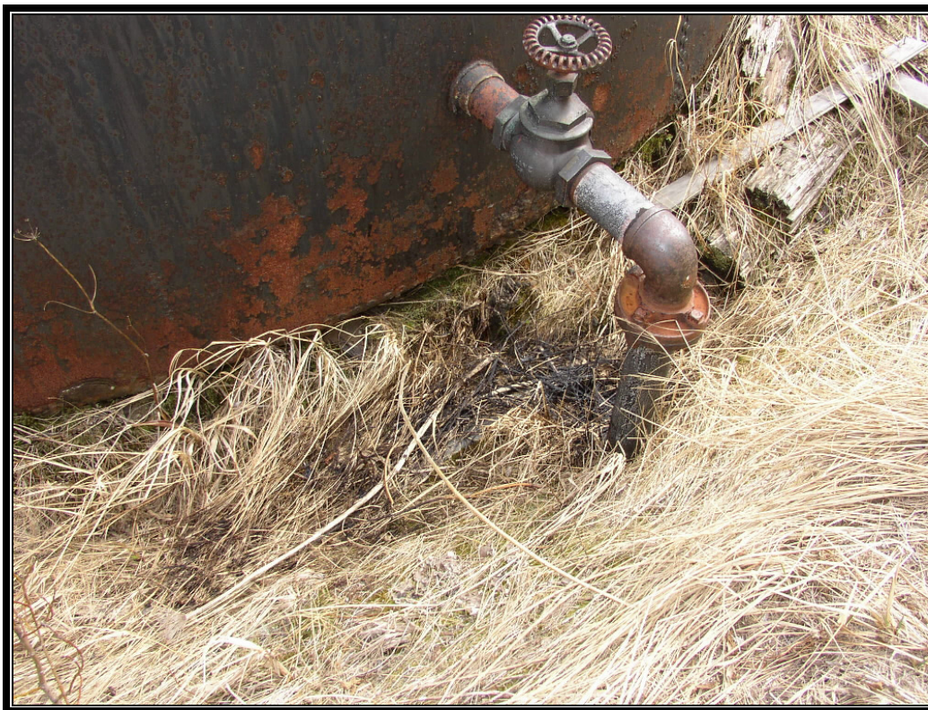
Photograph 18: Stain noted near the outlet of one of the aboveground storage tanks during the site visit. This stain was located inside the bermed area and was less than 1 square foot in area.
