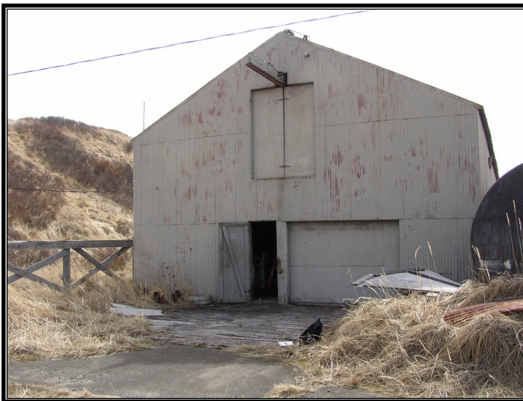
Photograph 24: North end of building J. Some of the original red paint is visible on the building exterior; most of the original paint has peeled off.
