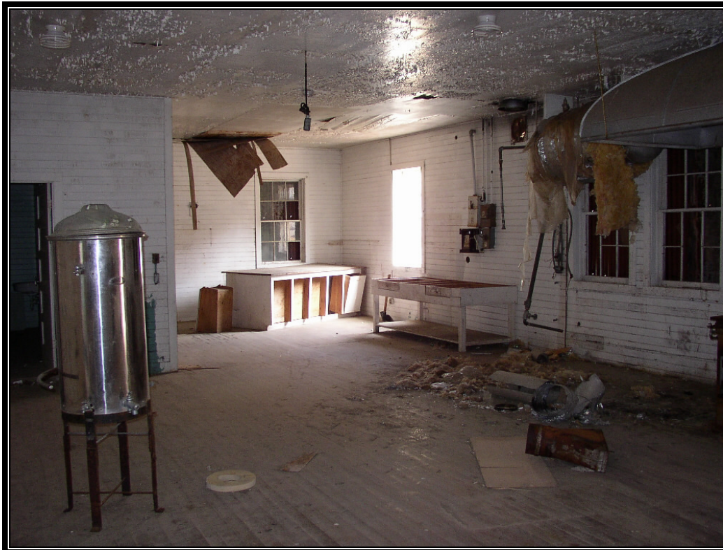
Photograph 11: Interior of the Former Cookhouse (Building E). Note the flaking ceiling paint and shredded insulation.
