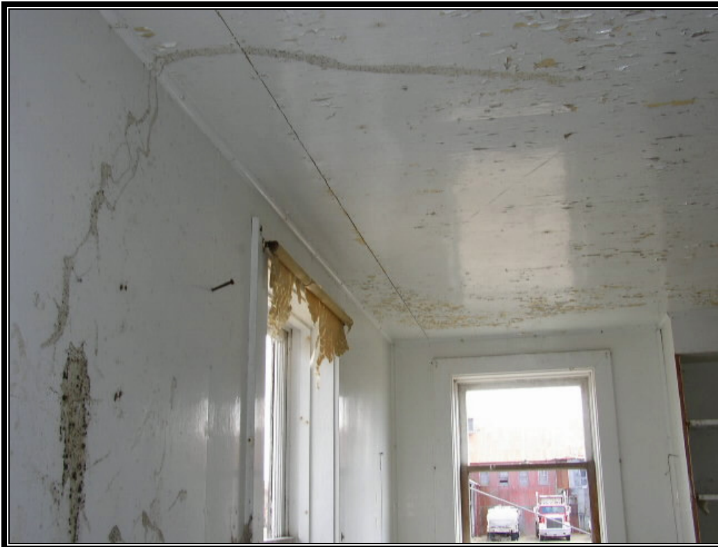
Photograph 41: Peeling paint noted on ceiling inside Building B.
