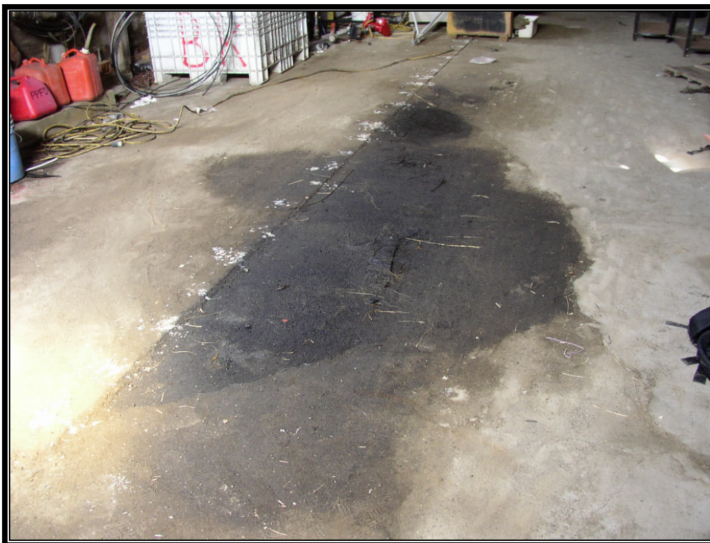
Photograph 2: Petroleum staining on concrete floor inside the Former Provision Warehouse (Building C).
