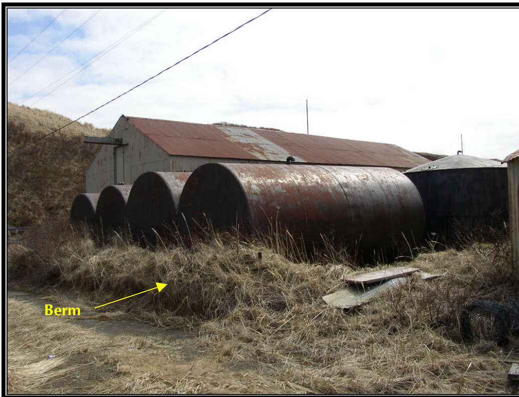
Photograph 16: Tank farm located at south end of subject property. The tanks are surrounded by an earthen berm. There was no liner present in the secondary containment area at the time of the site visit.
