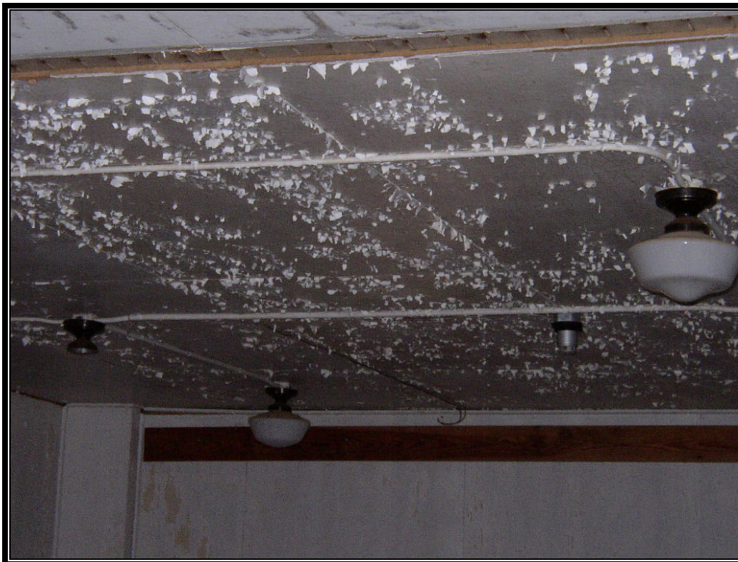
Photograph 8: Flaking paint on ceiling inside the Former Webloft (Building D).
