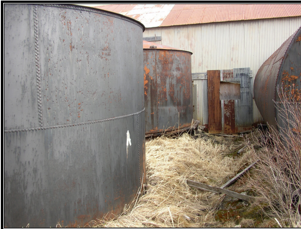
Photograph 19: Wooden debris located within the tank farm. There is visible rust on all of the tanks in the tank farm.
