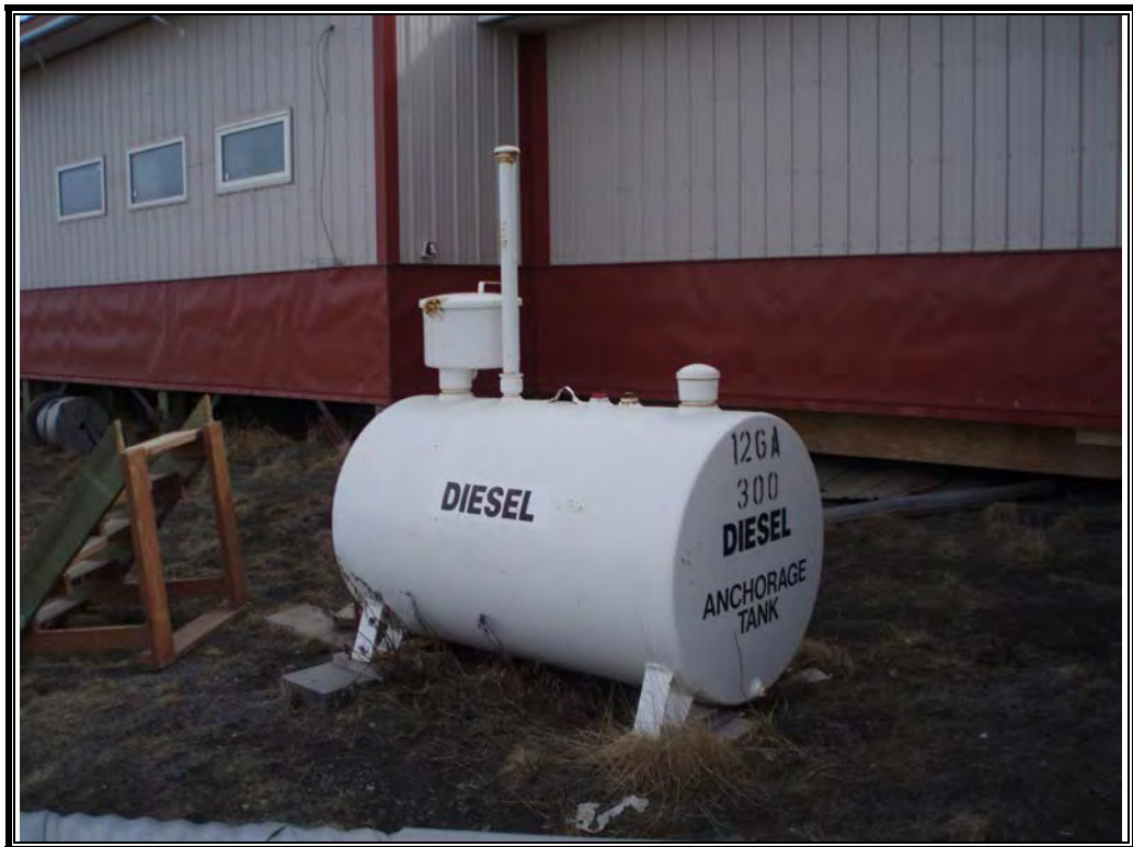
16. Photograph of representative heating oil tank located on the subject property. Two heating oil tanks are connected to the community center on the property.
