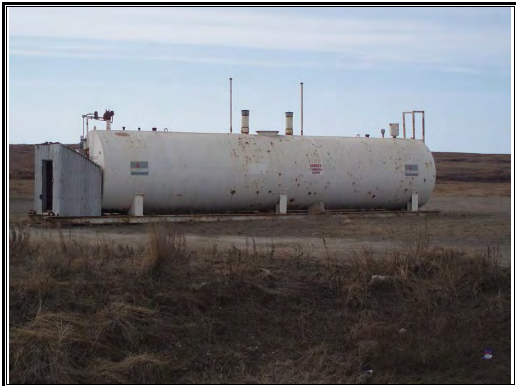
8. An empty, unconnected AST located on the property.
