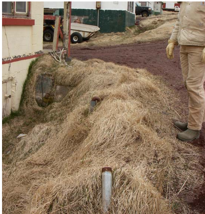
Photograph 4. Cottage D. Overgrown vent and fill pipes for UST on the south side of the building.
