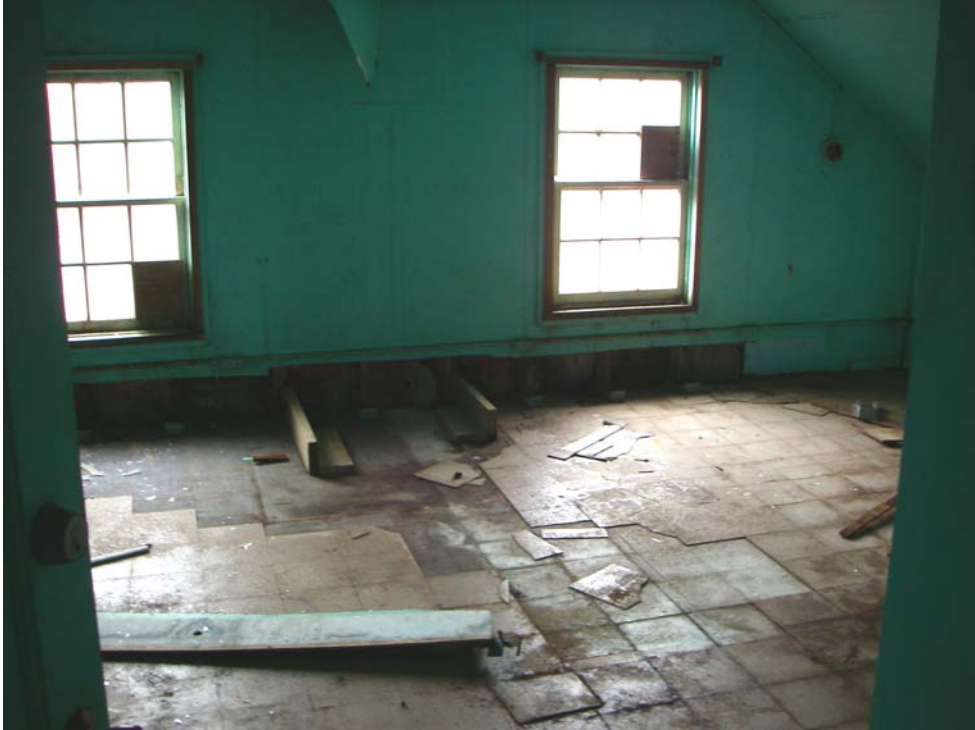
Photograph 7. Cottage G. Asbestos-containing floor tile from second-floor apartment.
