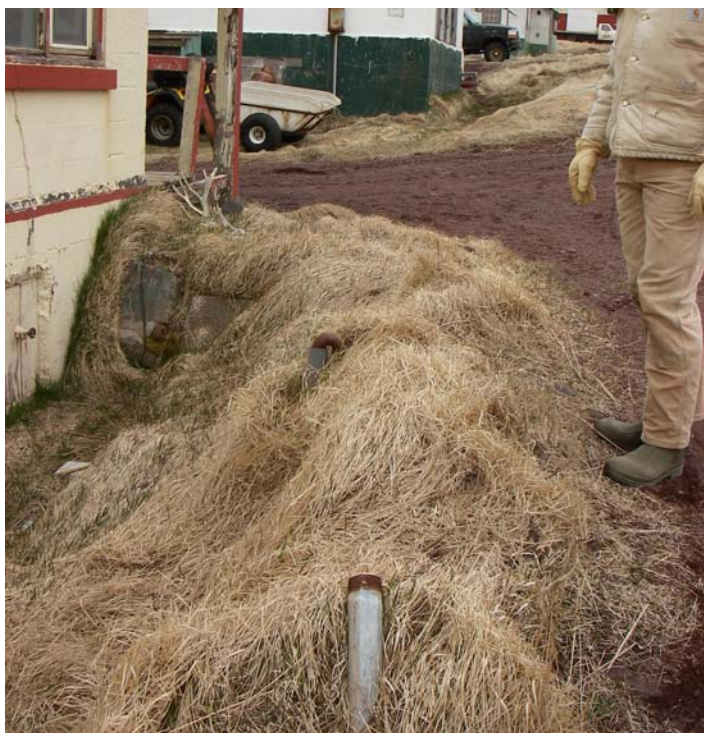
Photograph 9. Cottage D, south side. Overgrown UST fill and vent pipes
