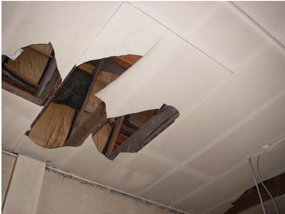
Photograph 2. Old Machine Shop. Asbestos-containing ceiling tiles.
