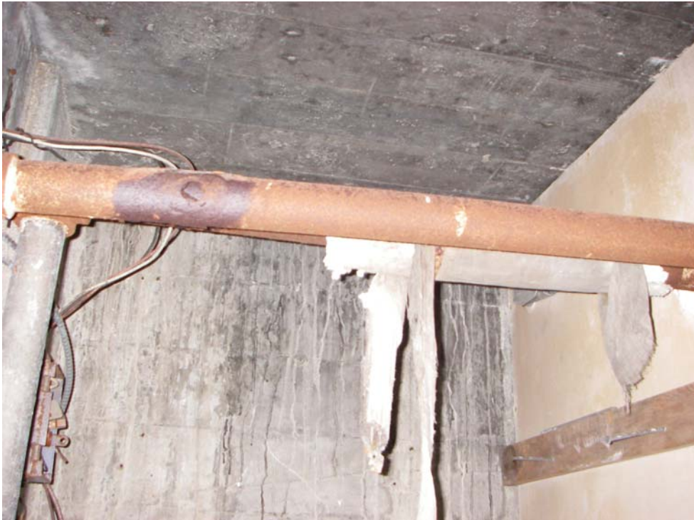
Photograph 3. Old Machine Shop. Asbestos-containing pipe insulation.
