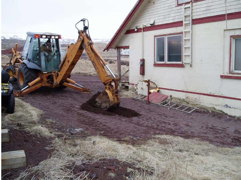
Photograph 5. Cottage D. Test pit 3 adjacent to active UST.
