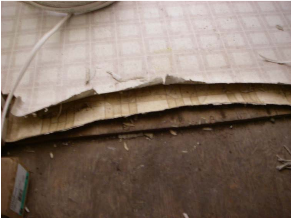
Photograph 6. Cottage G. Asbestos-containing flooring from entrance to furnace room in first-floor apartment.
