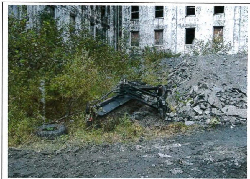
Photo H-34: Discarded materials observed between Sections E and G; looking west. (September 8, 2014)
