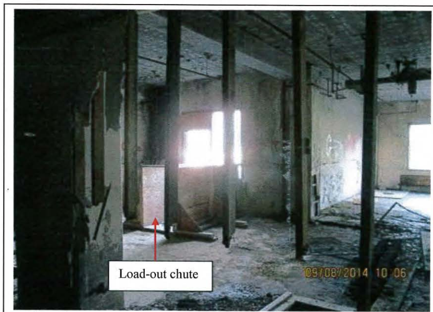
Photo H-22: What appears to be a load-out chute was observed on the ground floor level near the juncture of Sections A and C. (September 8, 2014)
