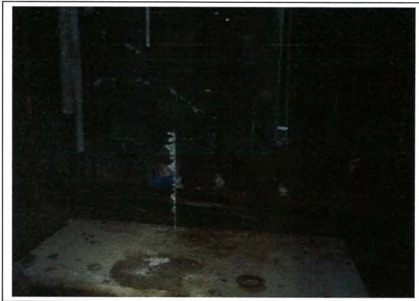
Photo H-6: Presumed concrete pad for the former generator in Section A of the basement of the Buckner Building. Note the surface stains on the concrete pad. (September 8, 2014)
