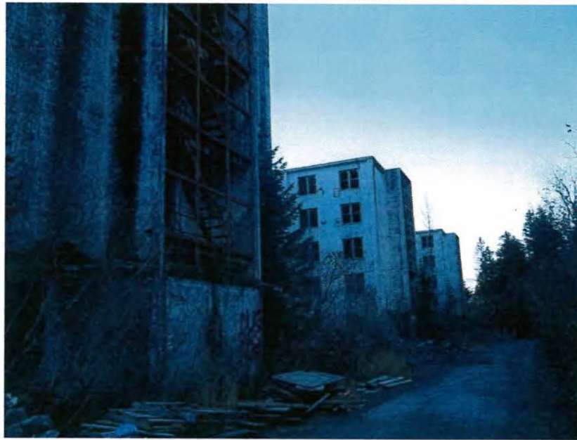
Photo H-35: Pallets and general construction debris observed between the Buckner Building and Eshamey Loop; looking northeast. (October 22, 2014)
