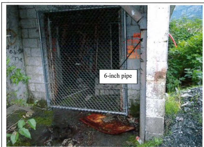
Photo H-30: Six-inch pipe observed near the northeast corner of the structure; looking northwest. (October 22, 2014)
