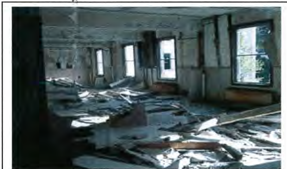
Photo 5: Representative second floor living quarters. September 8, 2014.
