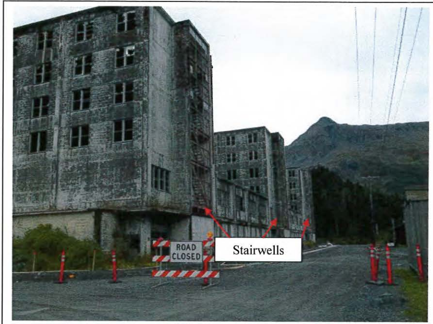
Photo H-1: Exterior of Buckner Building with exterior stairwells highlighted by arrows; looking southwest. (September 8, 2014)
