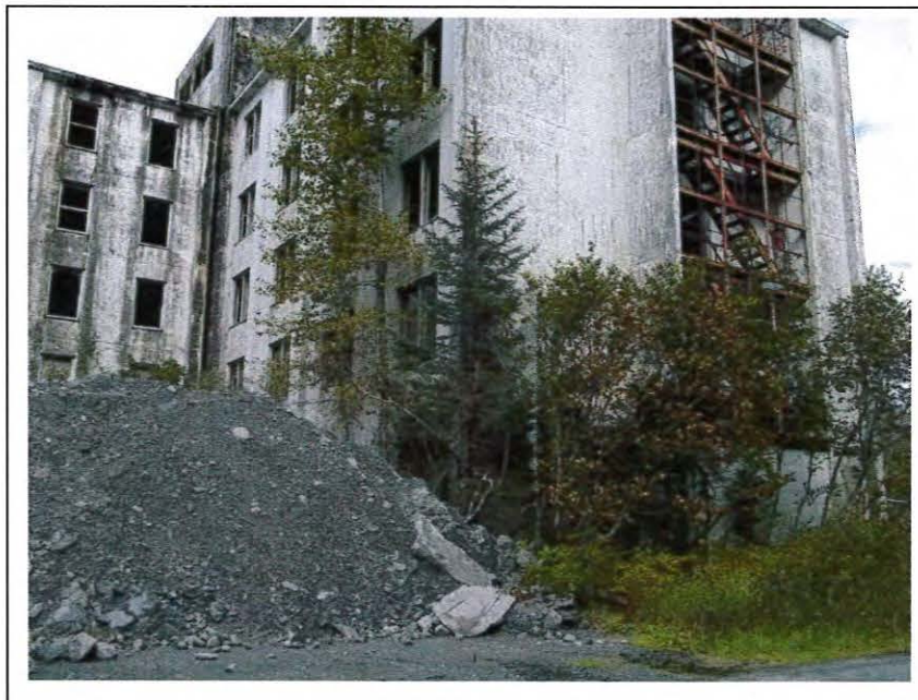
Photo H-32: Soil, asphalt, and concrete rubble stockpile observed between Sections E and G; looking north. (September 8, 2014)
