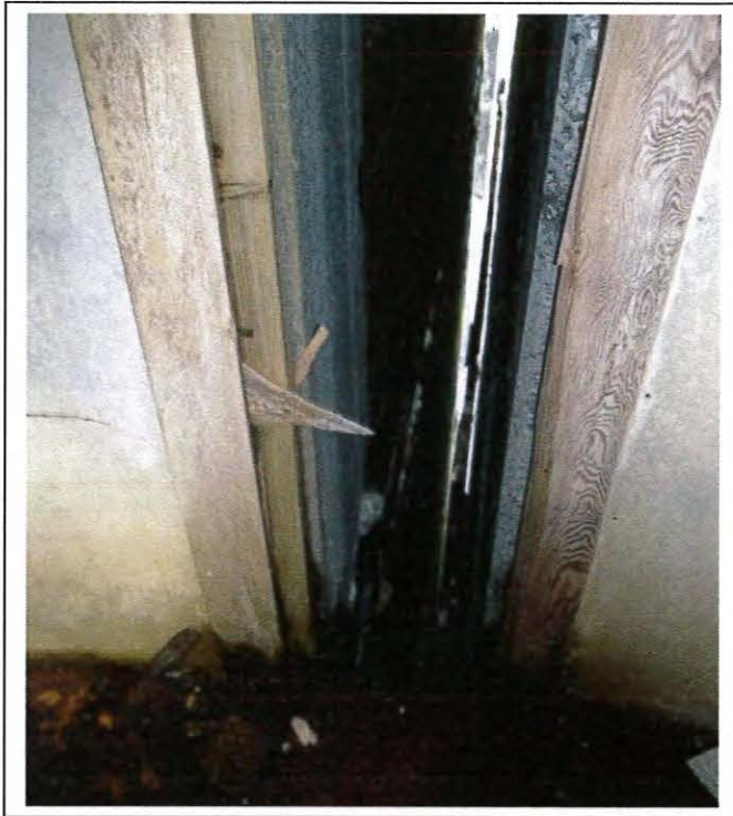
Photo H-3: Representative 8-inch "crumple" joint that separates the Buckner Building's seven structural sections. (September 8, 2014)
