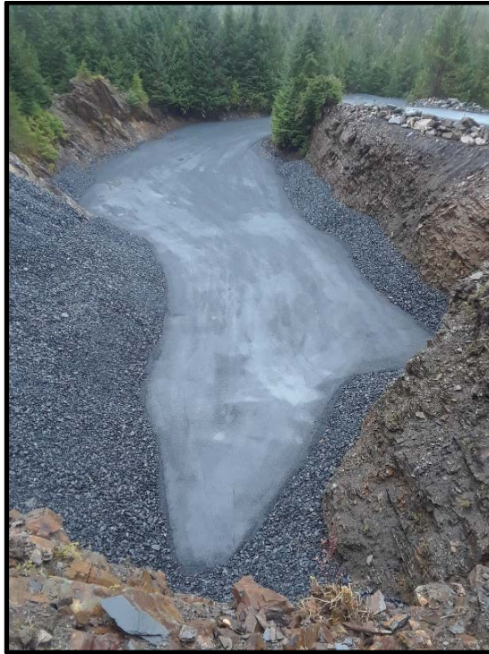
Photo 1: Looking north from above at the monofill repository site after completion of two-foot base course of drain rock. Site drainage is to the north into a drainage channel along the west and northern edges of the repository beginning in upper left of image, then to the east.
