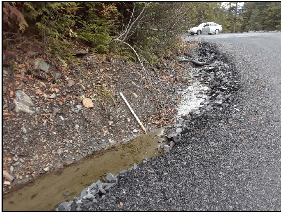
Photo 3: Looking northeast at the drainage channel along the northern edge of the repository site. Note surface water in portion of channel at left prior to entering the French Drain which diverts flow subsurface to the east beneath parking area rock pad (location of car in image).
