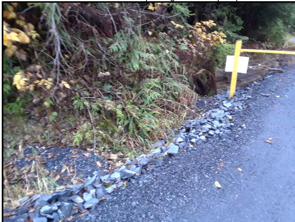
Photo 4: Looking north at continuation of secondary site drainage channel along west side of access driveway to the site. Note absence of water in the drainage. This drainage provides overflow of water beyond carrying capacity of the French Drain system.
