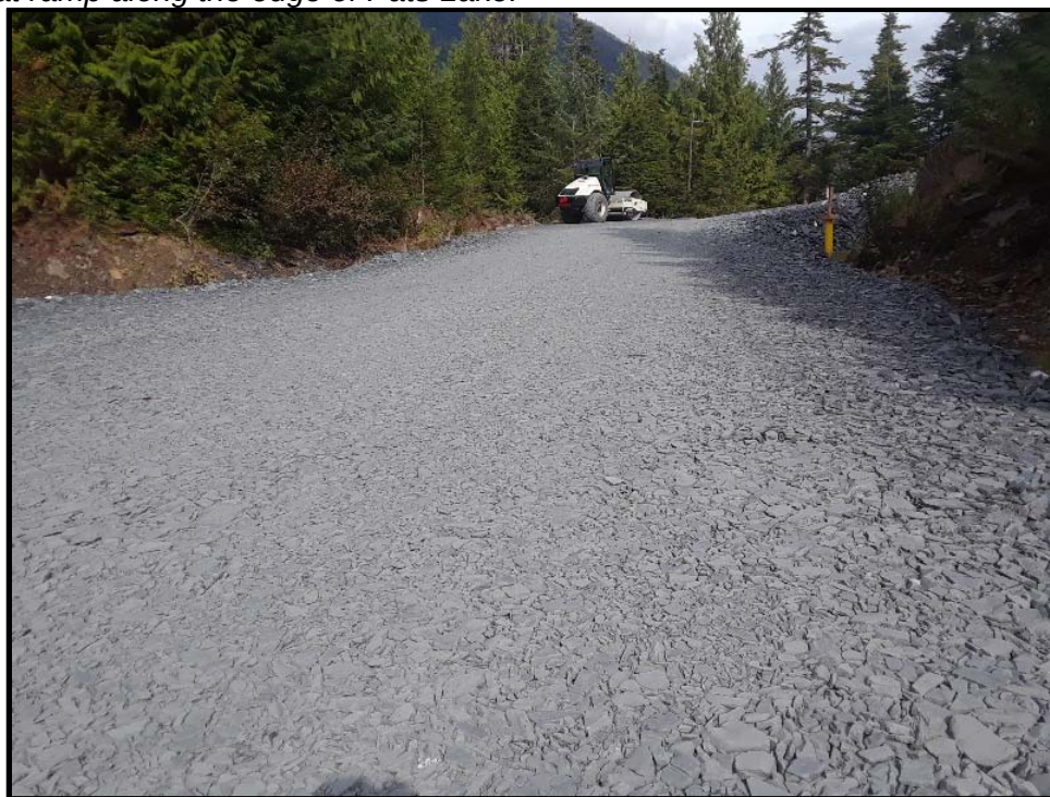
Photo 18: Looking northeast at monitoring well (yellow monument at image right) remaining in the northeastern portion of the repository site. Samples MW-3 and MW-13 (duplicate) were collected from this well.
