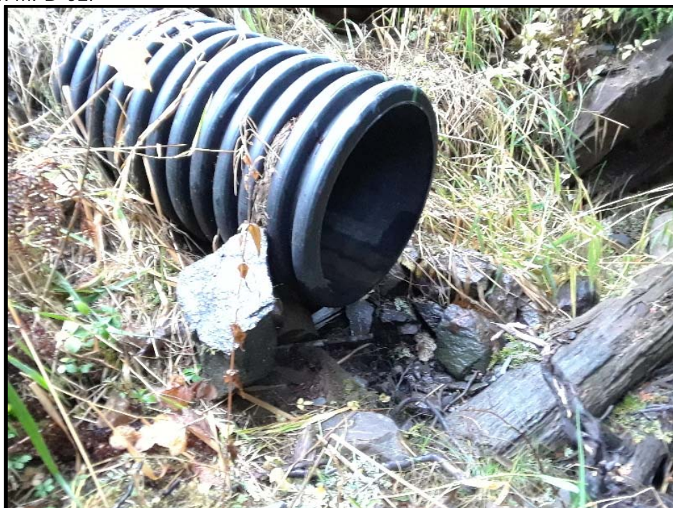
Photo 8: Looking southwest at sampling location MFD-02. This culvert discharges water from the repository site via the secondary site drainage channel, beneath Pats Creek Road and into a forested slope north of the Road.
