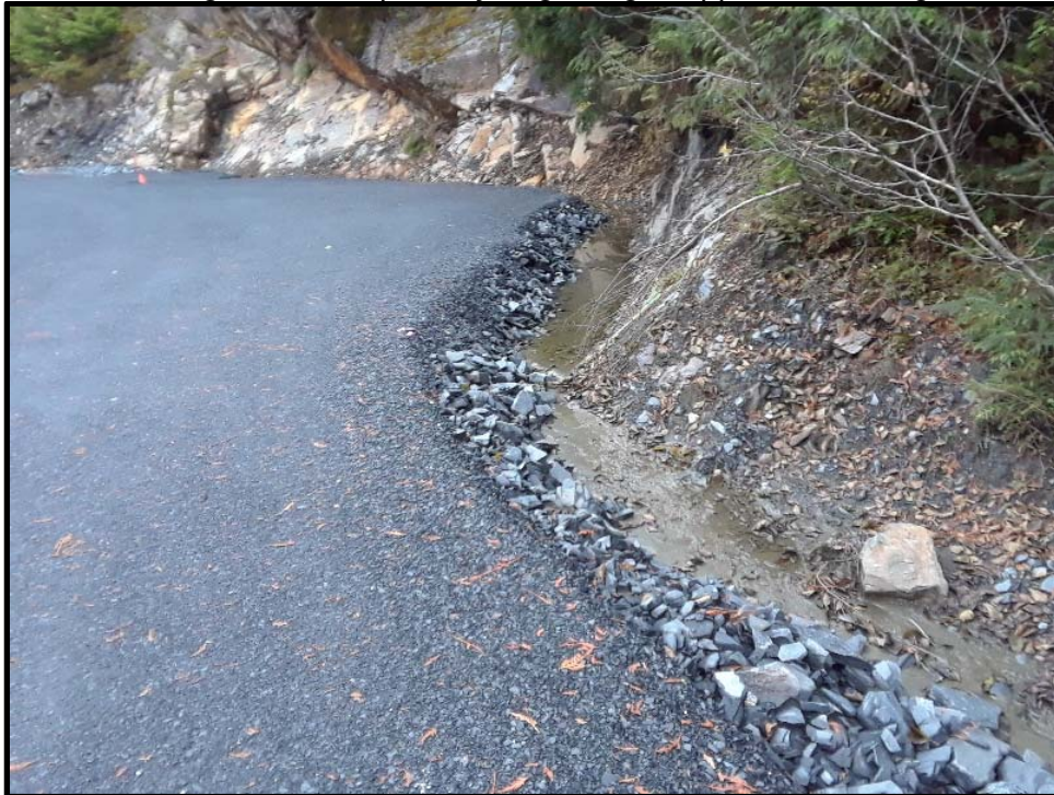
Photo 2: Looking west at the drainage channel along the northern edge of the repository site.
