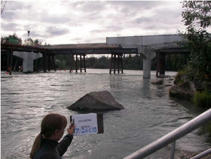
Figure 10: Kenai River Mile 21 (Soldotna Bridge) on 07/26/05.
