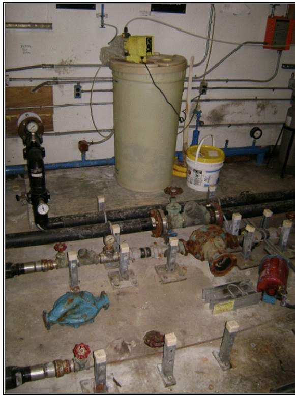
Photo 15: Watering point distribution piping circulation pumps (foreground) dismantled and inoperative.
