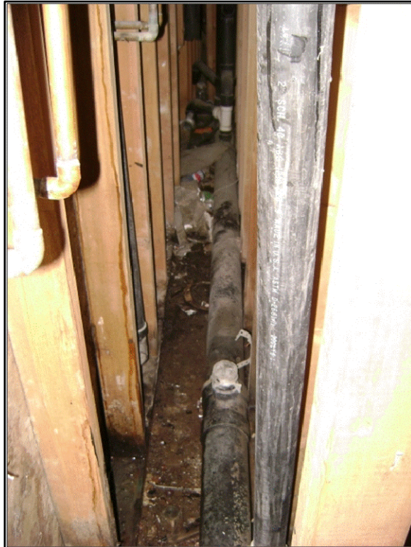
Photo 10: Showing disconnected drainage piping improperly sealed.
