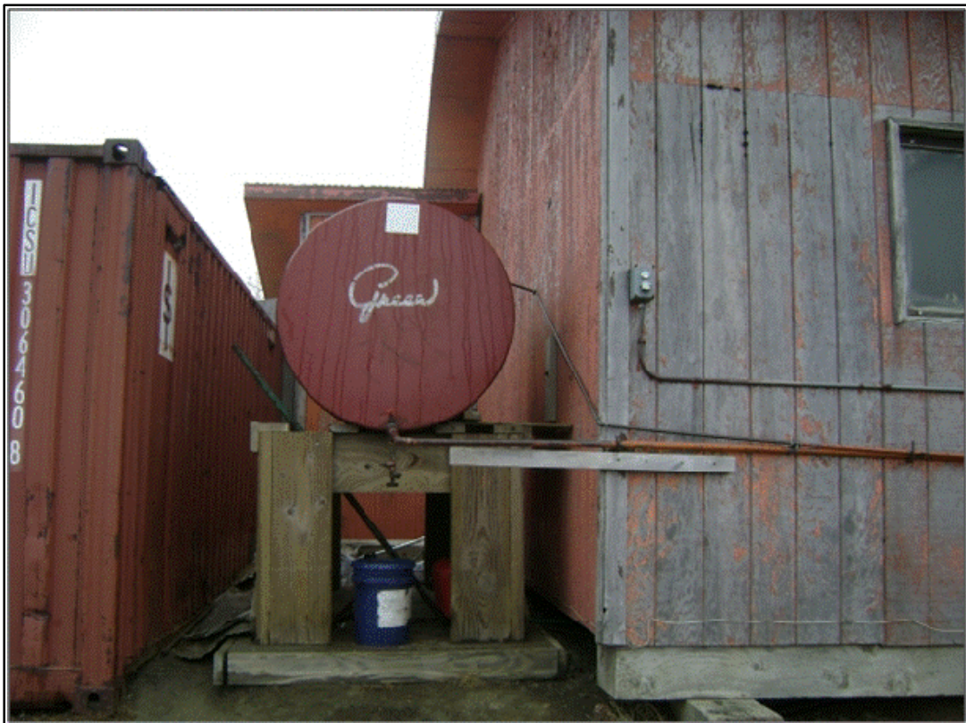
Photo 12: Building fuel supply tank located too close to building. Piping is not properly connected. Fill access is at rear contributes to fuel spill potential.
