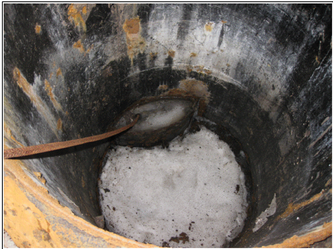
Photo 38: Ice blocked outlet baffle in septic tank #1 on the In-Complete septic system.
