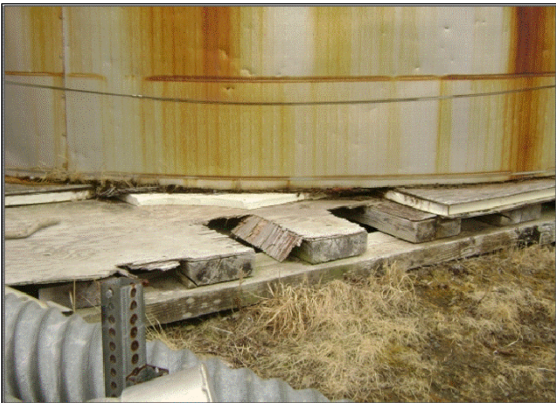
Photo 6: Deteriorated tank foundation.
