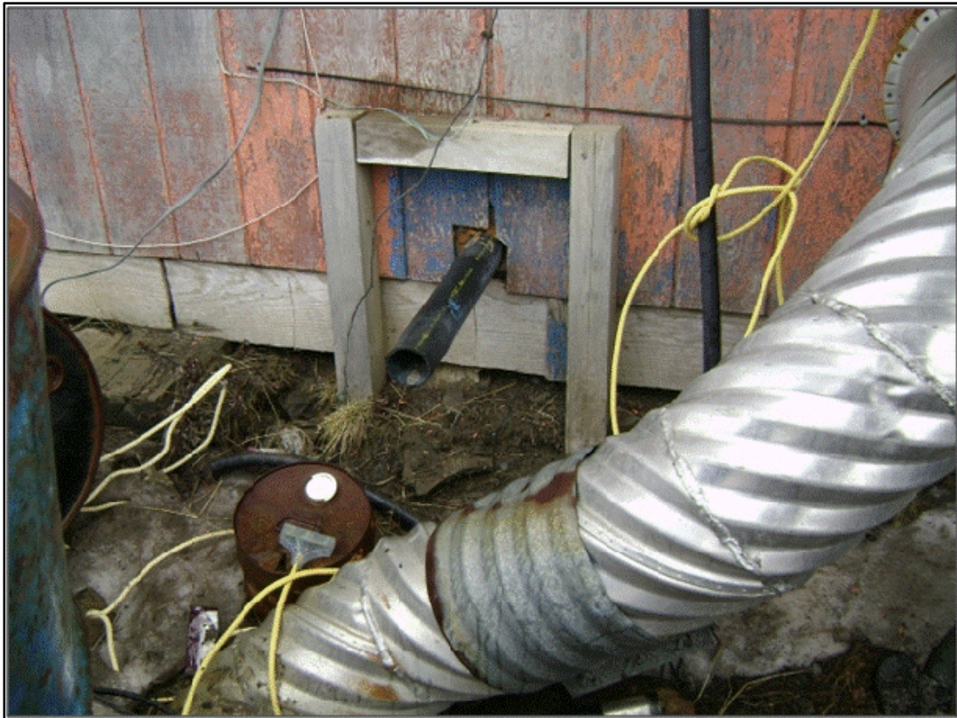
Photo 5: Discharge from filter backwash above Arctic pipes.
