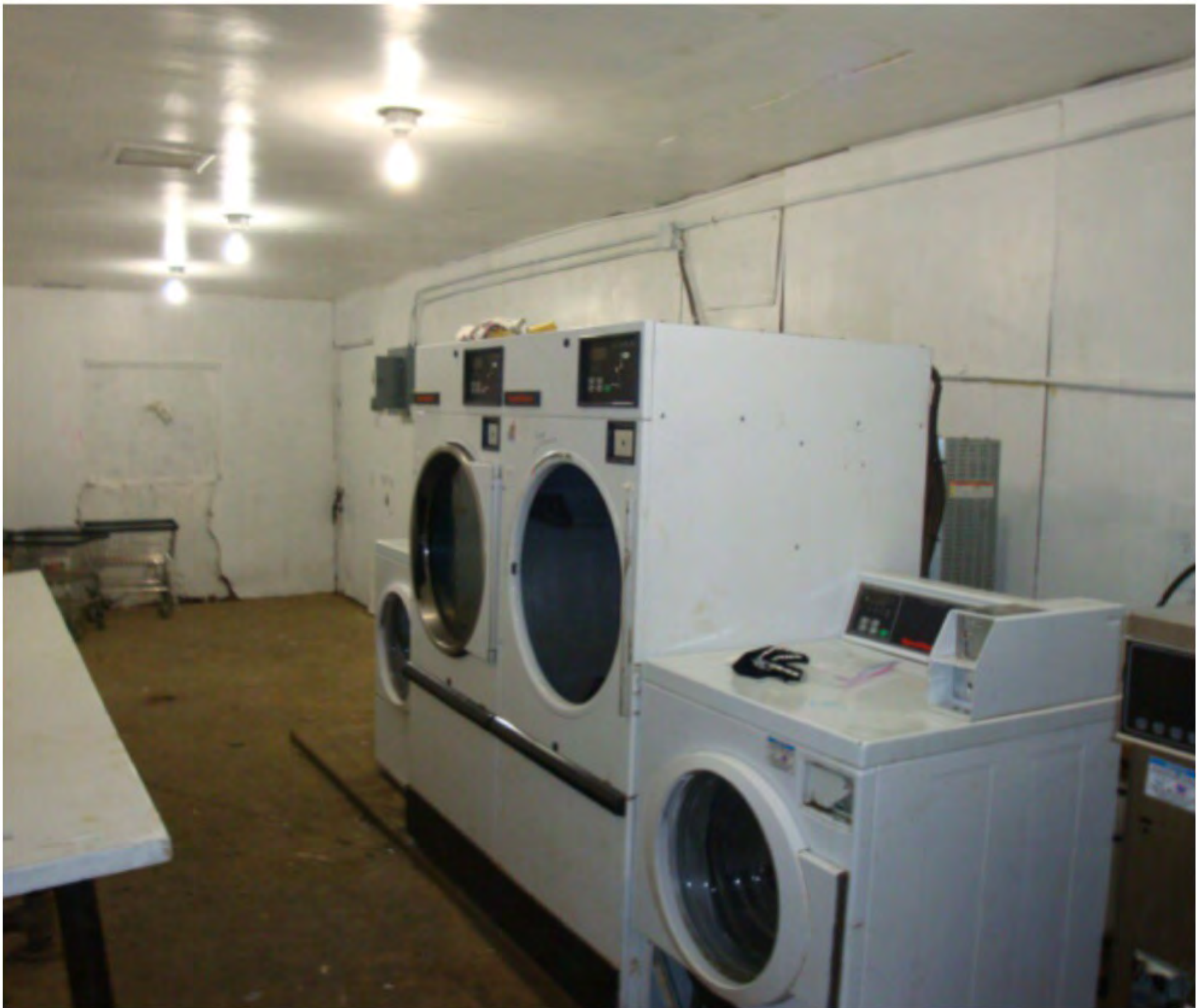
Tununak Washeteria - Speed Queen SWRX7 18 pound capacity washers and 30 pound electric dryers.
