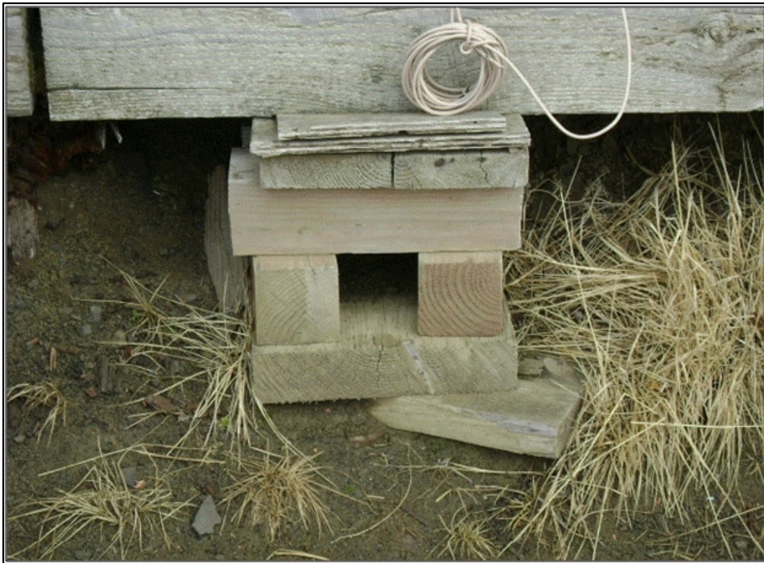
Photo 4: Another footing eroded along south wall of water treatment plant building.
