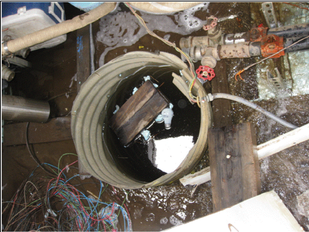
Photo 22: Interior condition of flooded well casing in Un-Named Creek well house.
