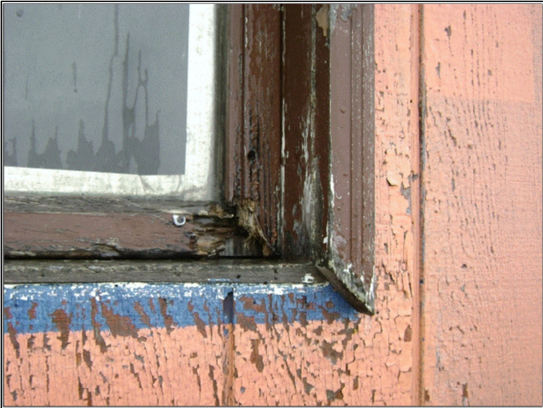
Photo 7: Rotted window frames and replaced glass with single pane Plexiglas or plywood.
