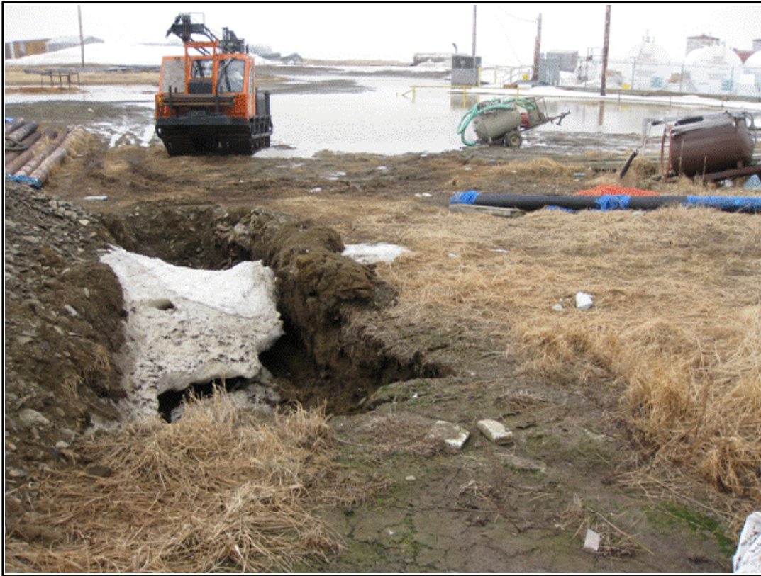
Photo 39: Open trench used for disposal of FTH hauled waste located near off-loading ramp on the In-Complete septic system.
