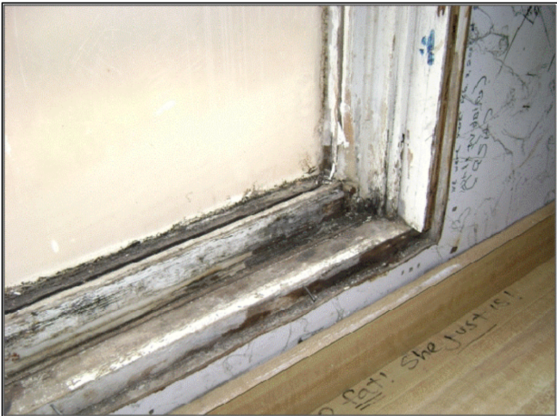
Photo 8: Rotted window frames and replaced glass with single pane Plexiglas or plywood.
