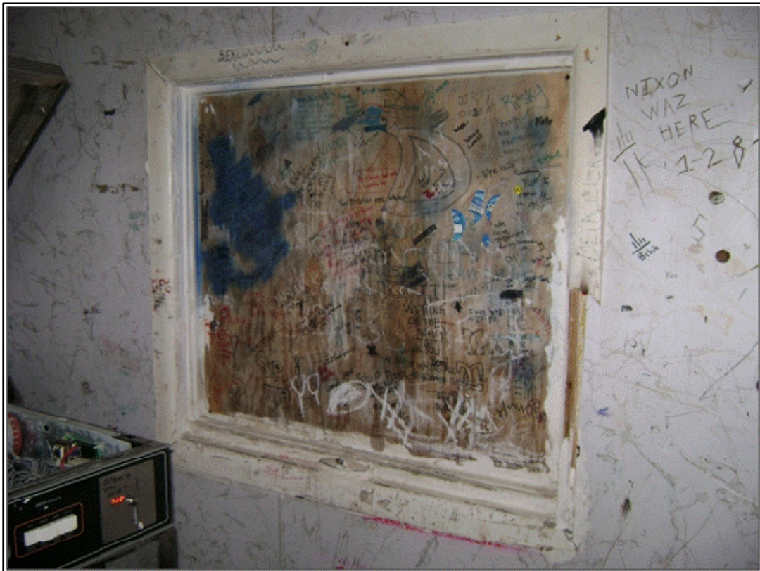
Photo 9: Rotted window frames and replaced glass with single pane Plexiglas or plywood.
