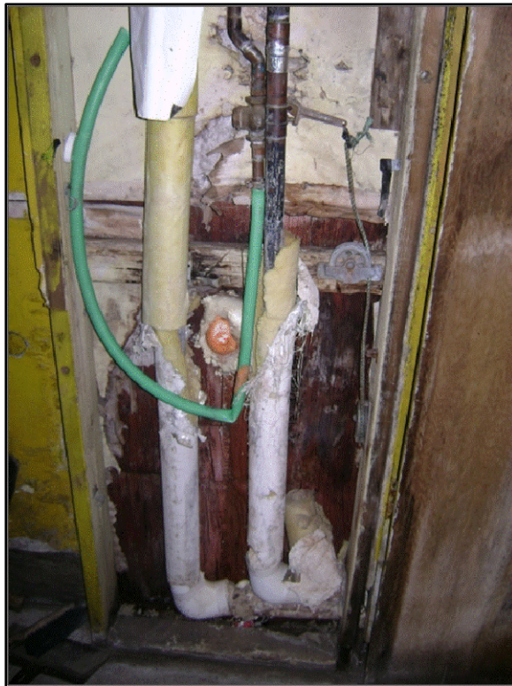
Photo 14: Abandoned watering point at south side of WTP showing deterioration of insulation and building envelope. Exterior siding is visible from building interior.
