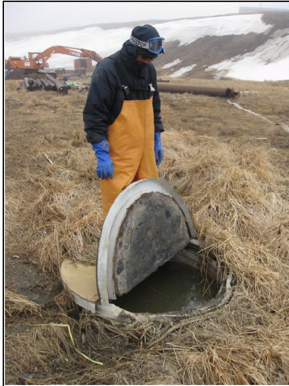
Photo 41: Overflowing sewage in manhole on septic tank serving the Washeteria, teacher housing, and school.
