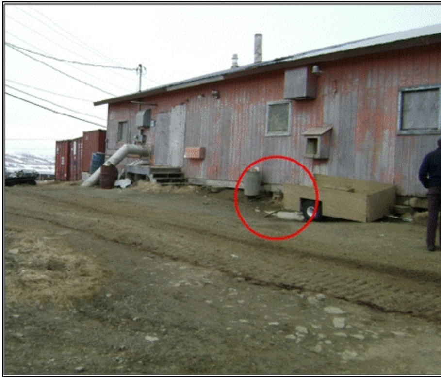
Photo 1: South side of the Water Treatment Plant Washeteria Abandoned watering point drainage area (circled). Boarded-up door to boiler room. Arctic pipeline to clinic in background.
