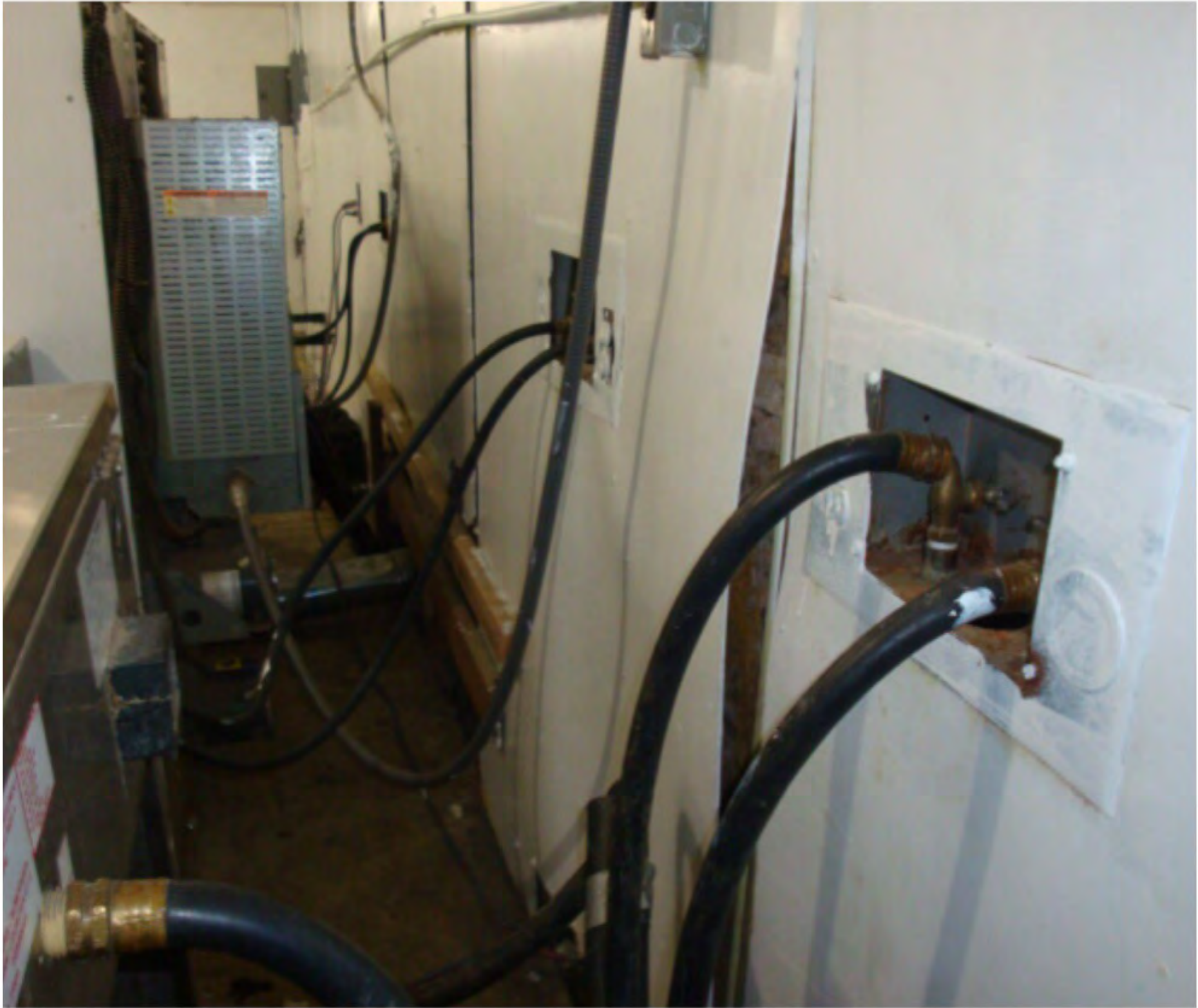
Tununak Washeteria - space behind machines. Note the wall splitting, and corrosion.
