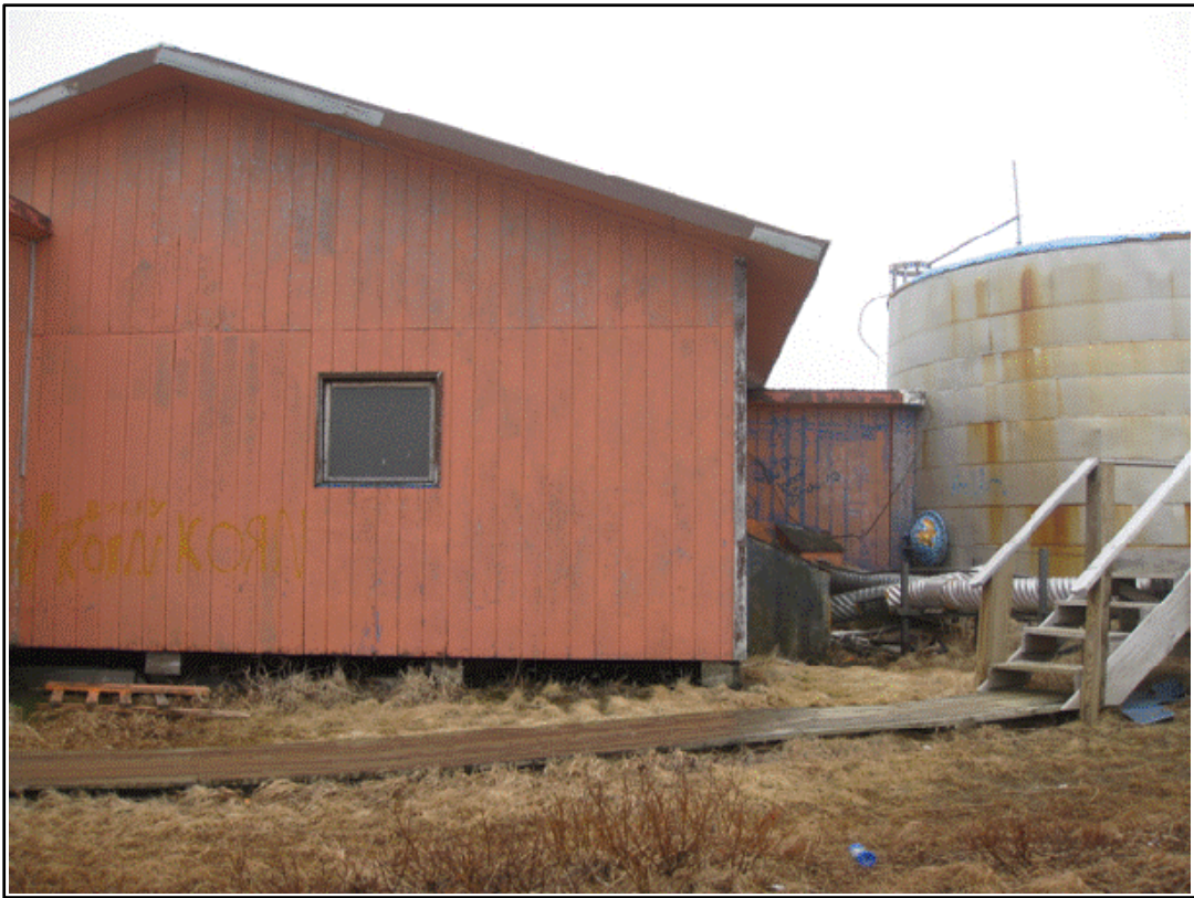
Photo 35: WTP/Washeteria connection to water storage tank.
