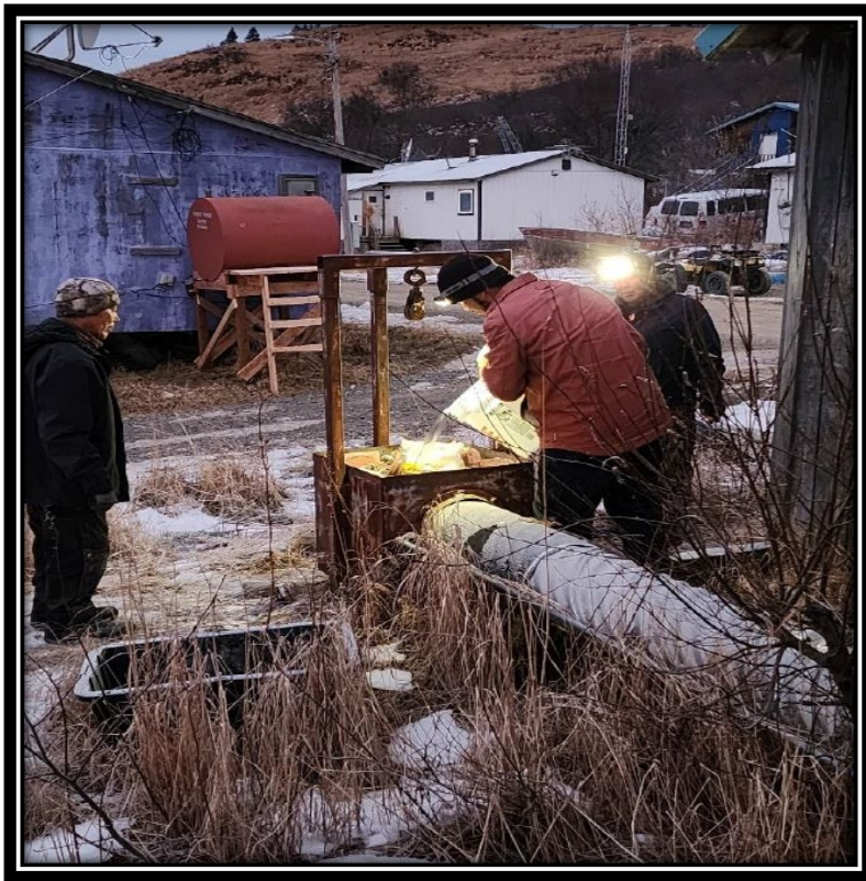
BBAHC RMWs assisting with well chlorination in Manokotak
